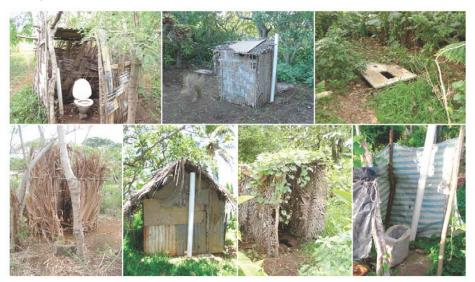
Figure 4: Examples of poorly constructed and maintained VIP latrines on Tanna Island.
