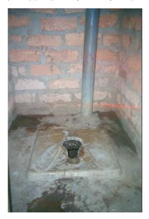
**Figure 7**: The ventilation pipe could be inside or outside depending on choice. The critical technical specification being the height of the pipe above the pit and the way the faced the prevailing winds. (Photo provided by Paul Deverill, WEDC).
