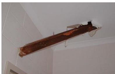
Houses damaged by wind-borne debris during TC Larry (Innisfail, Qld, 2006)
