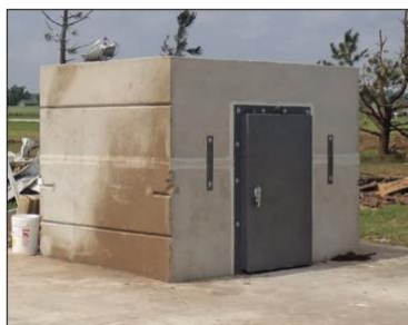
Stand-alone room near a house still intact after a tornado (FEMA Taking shelter from the storm, 2014.)
