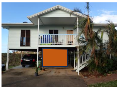
Strong room added under a high-set house
