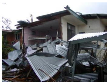
Houses damaged by wind-borne debris during TC Larry (Innisfail, Qld, 2006)
