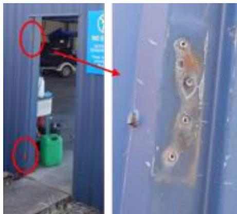
**Figure 4.49 Failure of door hinges**
