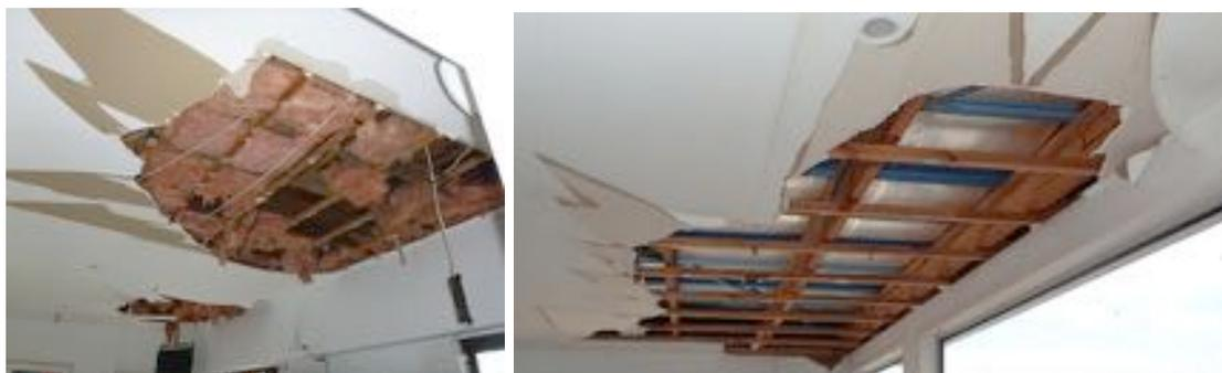
**Figure 5.2 Examples of damage to plasterboard ceiling caused by rain being driven under inadequately secured flashings**
