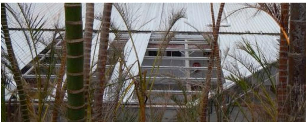
Figure 4.5 Clip-fixed roof cladding failure
