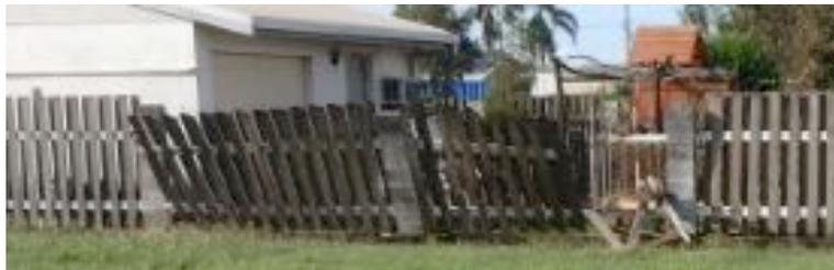
(b) Masonry column failure
