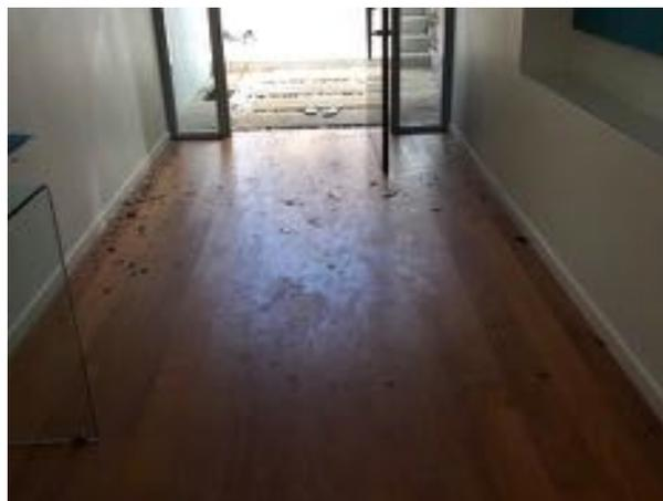
**Figure 5.32 Water ingress under swinging door**
