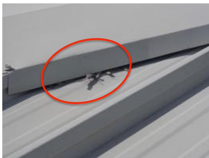
**Figure 5.20** Leaves driven under roof flashing
