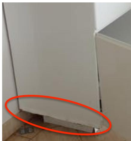
**Figure 5.8** Water damage to cupboards
