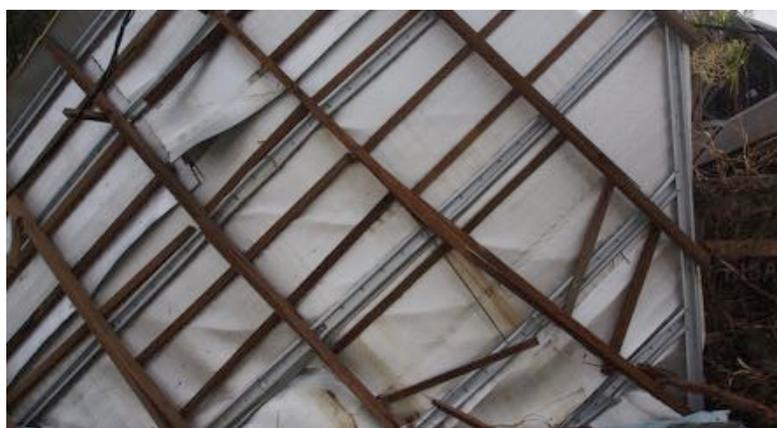
**Figure 4.19 Failure of roof structure to wall connections**
