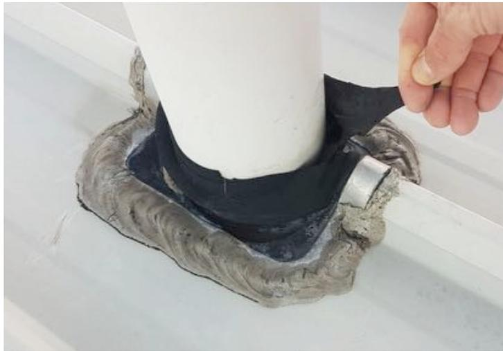
**Figure 7.15 Seals on vent pipes**
