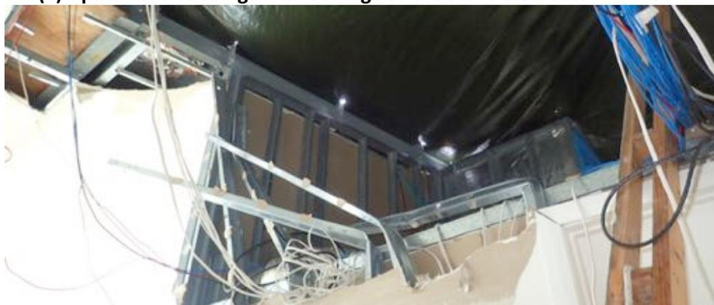
**(b) Loss of part of roof structure at the top of walls**
