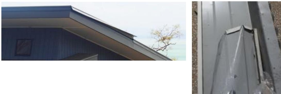
**Figure 5.13 Examples of barge flashings with no fastenings to walls**
