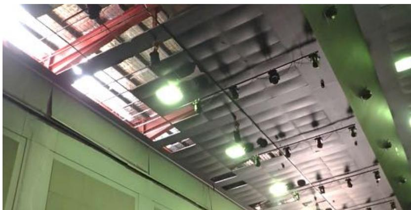
**Figure 4.36 Ceiling panels pushed down**
