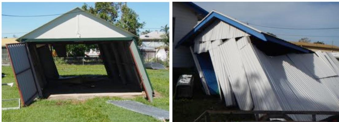
**Figure 4.44 Racking failures of framed sheds and garages**
