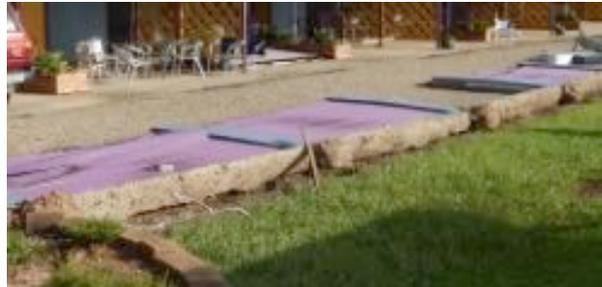
(a) Concrete footing over turning failure
