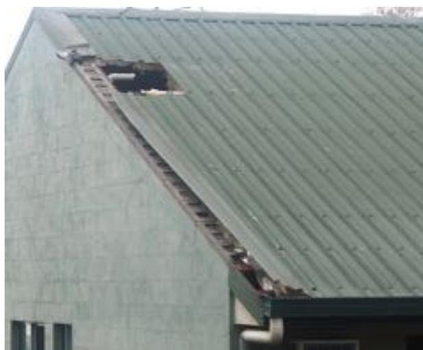
Figure 5.18 Loss of flashing contributed to loss of roof sheeting
