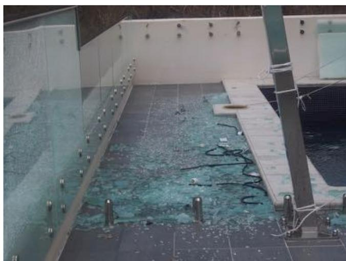
**Figure 7.7 Failure of unframed glass pool fence**
