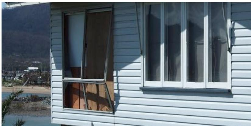
**Figure 4.28 Window frame of low strength**
