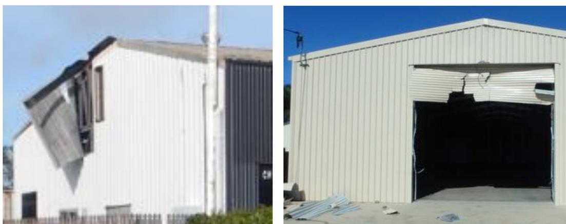
(a) Side wall cladding failure
