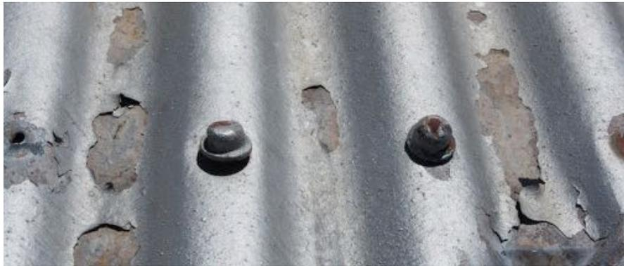
**(a) Nails used to secure roof cladding**
