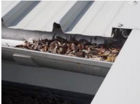
**(a) Blocked eaves gutter**
