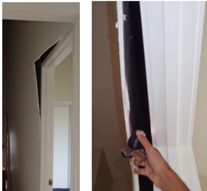
**Figure 5.5 Water damaged plasterboard wall partially detached from frame**
