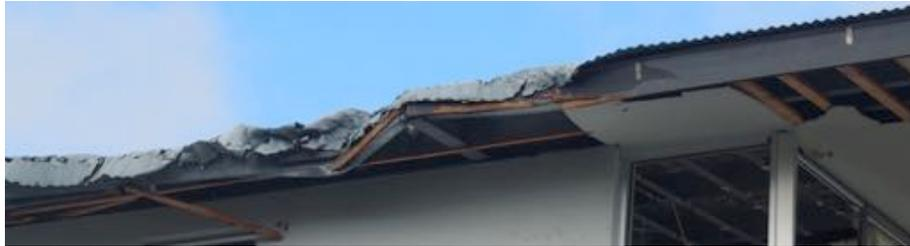
**(a) Debris damage to brittle soffits**
