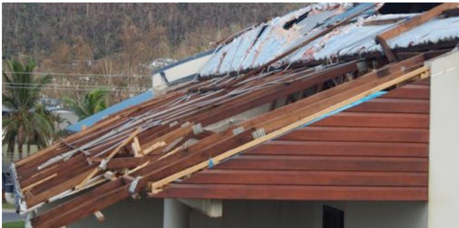
Figure 4.10 Batten-to-truss connection failures in contemporary apartments
