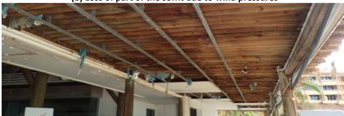
(c) Loss of all of the soffit linings
