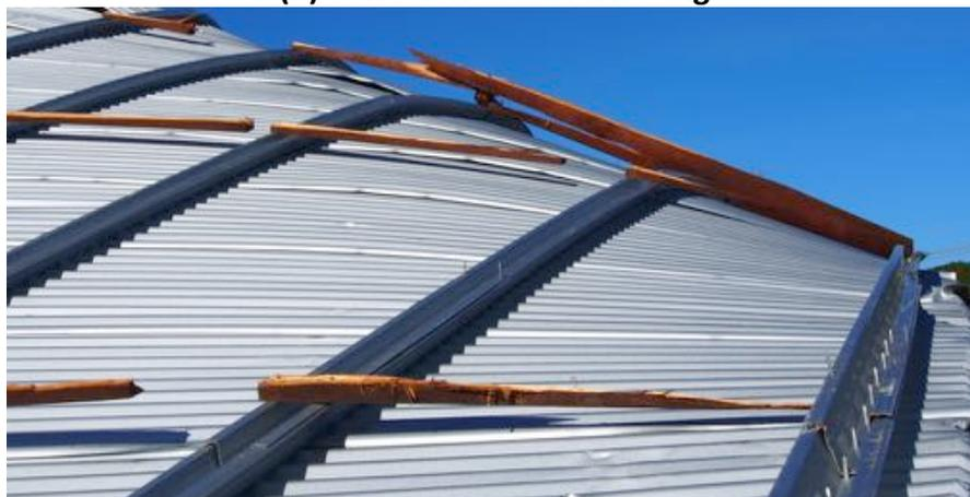
**(c) Failure of rafters in tension perpendicular to grain**
