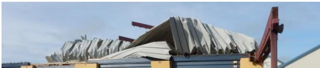
**Figure 8.5 Failure of a previously repaired roof**
