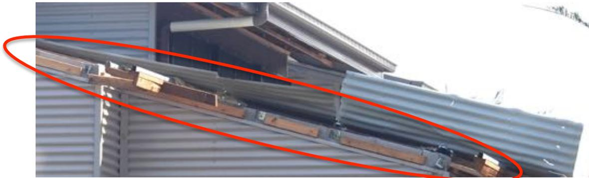
**Figure 4.14 Failure of brackets holding outriggers**
