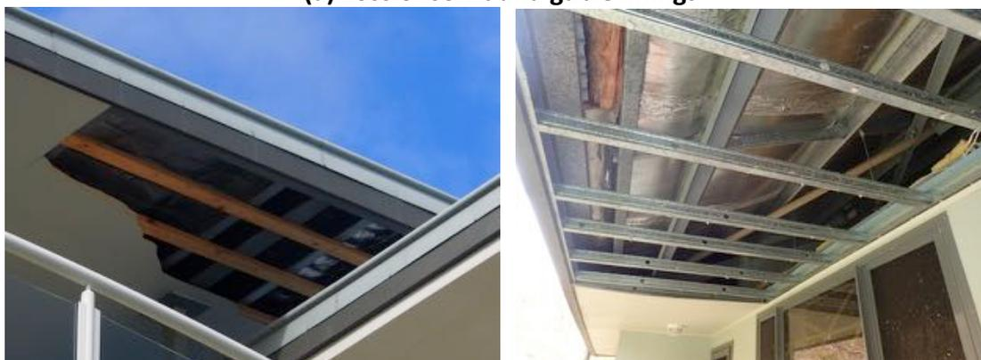
(b) Loss of part of the soffit due to wind pressures
