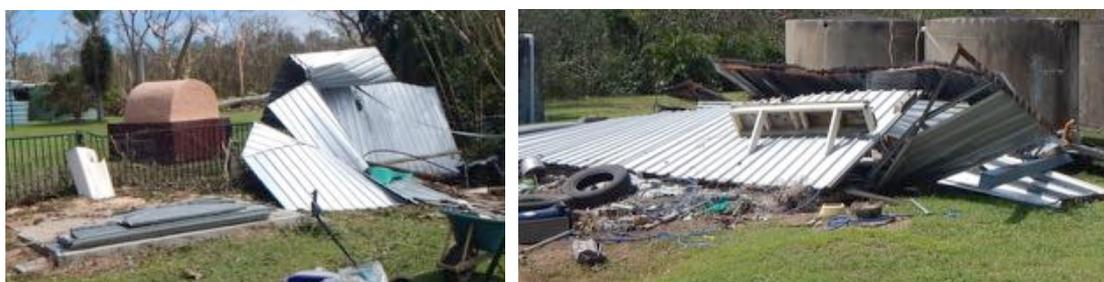
**Figure 4.45 Panel failures of garden sheds**
