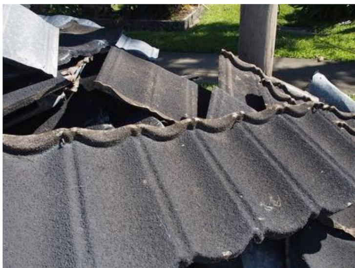
**Figure 4.3 Loss of metal roof tiles**
