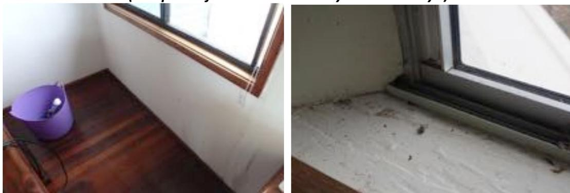
**(b) Damage to plasterboard under sliding windows**
