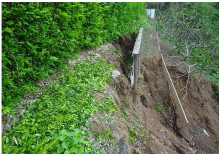
Figure B1 Erosion of landscaping over significant portion of property down slope
