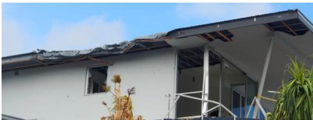
**Figure 4.51 Damage from larger debris items**
