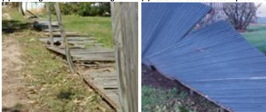
(a) Connection failure
