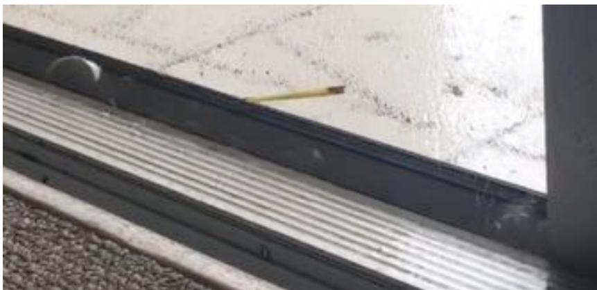
**(a) Rainwater bubbling and spurting through glass sliding door frame
