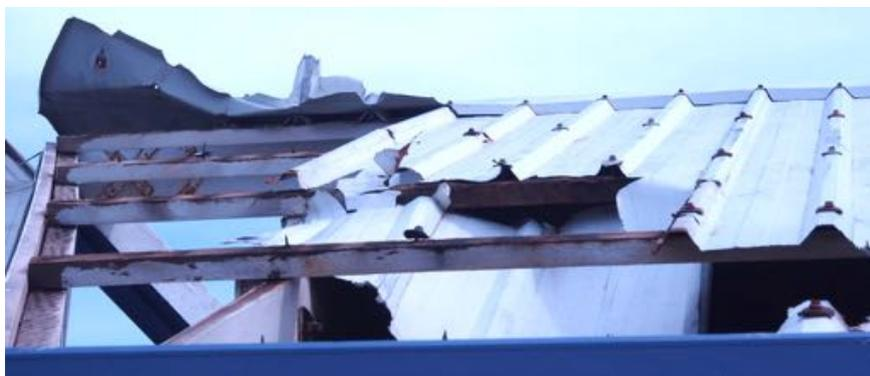
**Figure 8.6 Failure of roof due to corrosion of screws**
