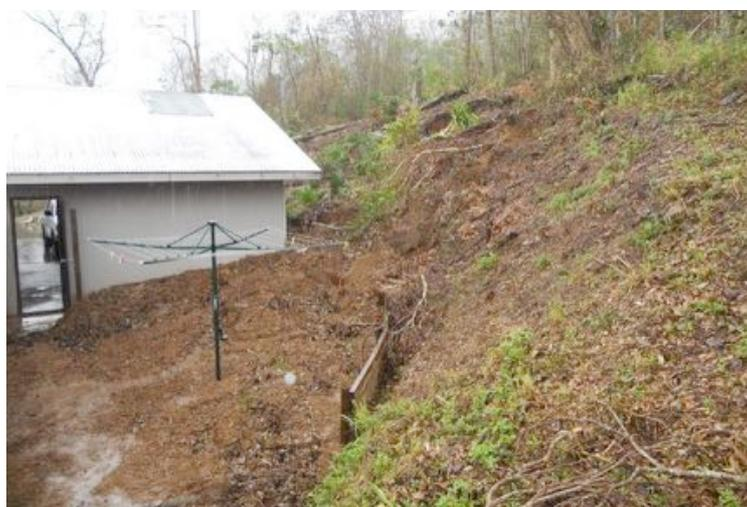
Figure B2 Landslide debris impacting house with material entering into house
