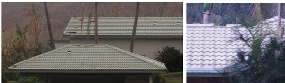
**Figure 4.8 Failure of tiles and ridge capping**
