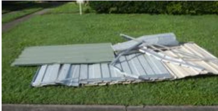
(b) Sheet metal fence panel failure
