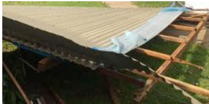
(b) Failure of roof panel
