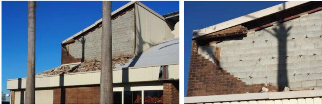
Figure 4.6 Failure of brick cladding
