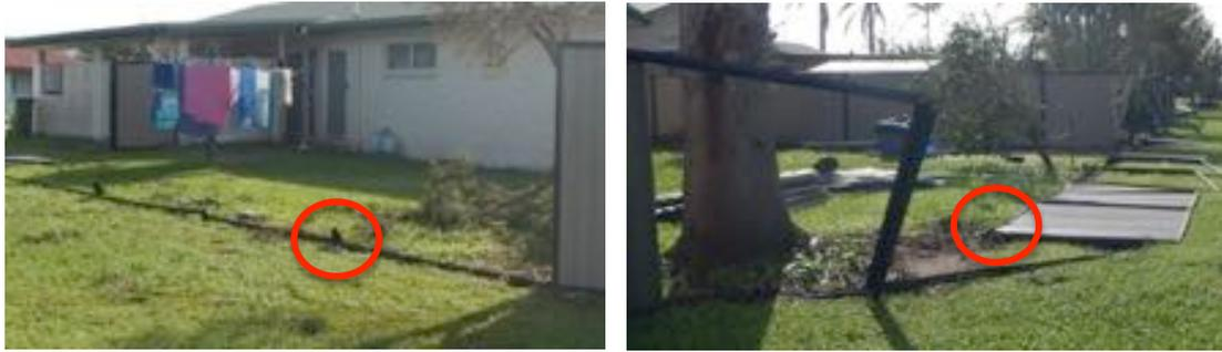
(a) Post failure of steel fence
