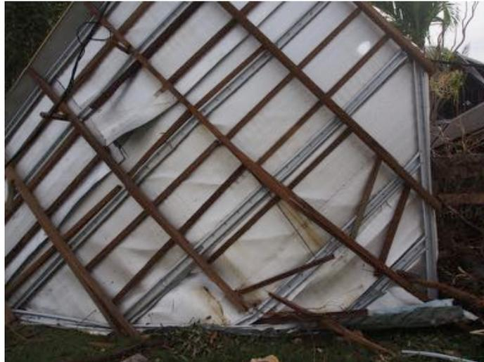
(a) Failure of roof where tiles had been replaced by sheeting
