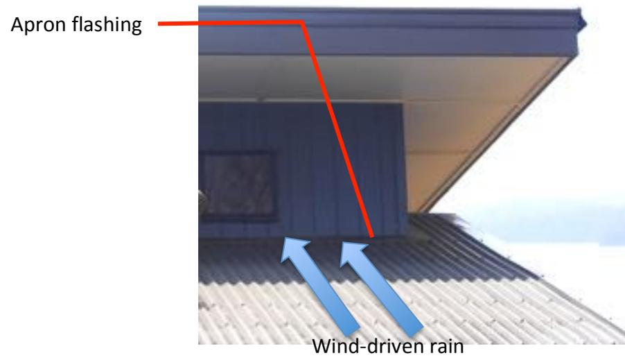
**Figure 5.21 Apron flashing on skillion roof**
