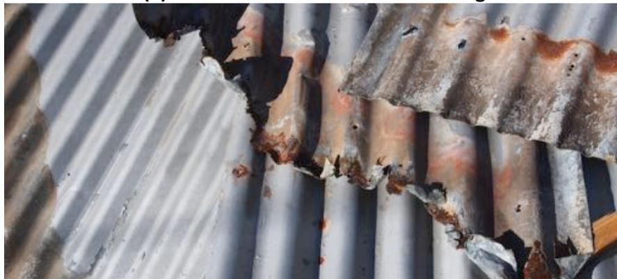
**(b) Corrosion of roof sheeting**
