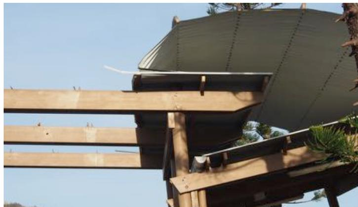
**(a) Purlin to rafter failure**
