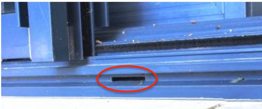
**Figure 5.25 Weep hole in glass sliding door frame**
