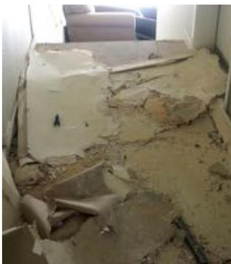
**Figure 5.3 Collapsed lower storey ceilings**
