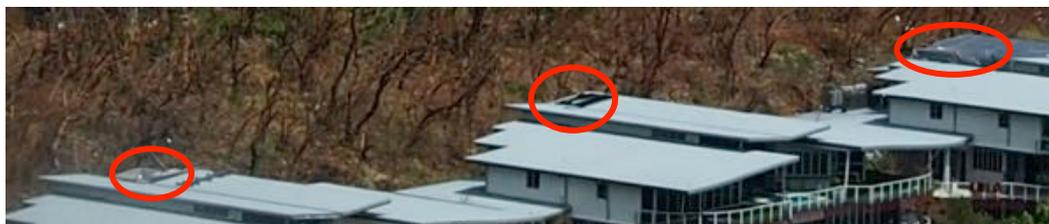
**(a) Apartment buildings with damage to the same elements in all roofs**
