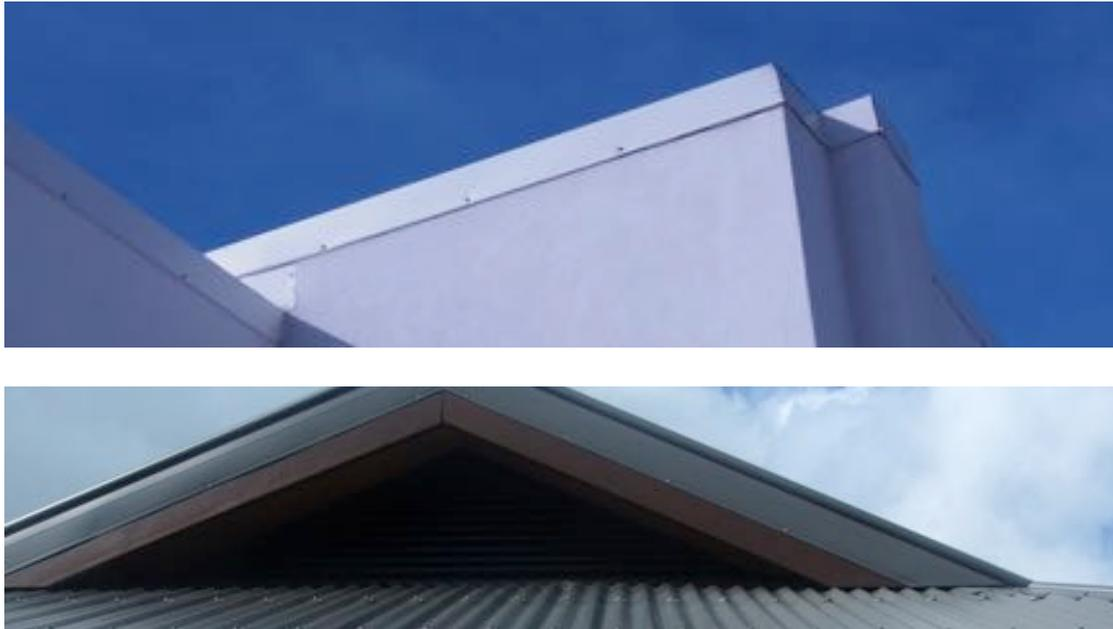
**Figure 5.15 Flashing fastened with screws on buildings in exposed locations that performed well during TC Debbie**
