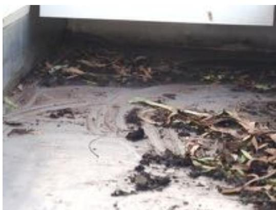
**Figure 5.23 Box gutter that had been blocked by tree debris**
