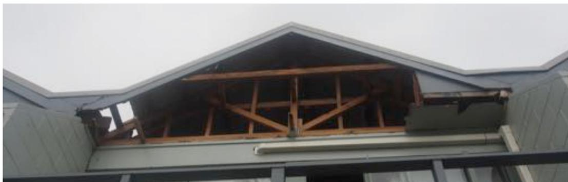
(a) Loss of soffit and gable linings
