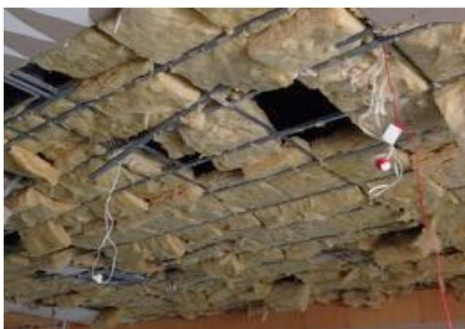
**(a)** Damage from ceiling loss
