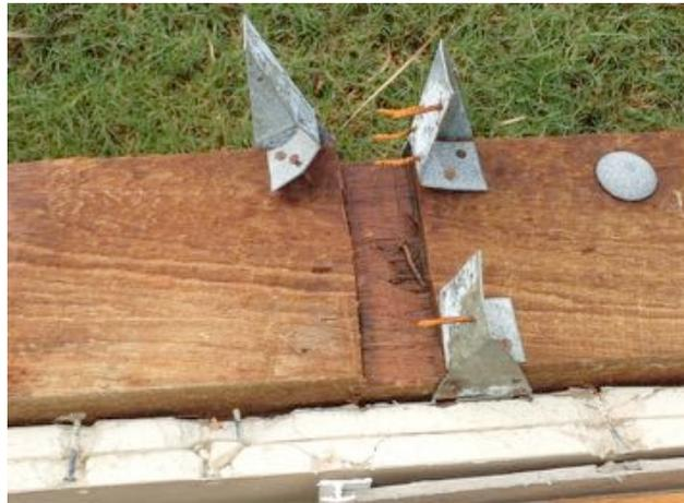
**Figure 4.16 Framing anchors between truss and verandah beam top plate**
