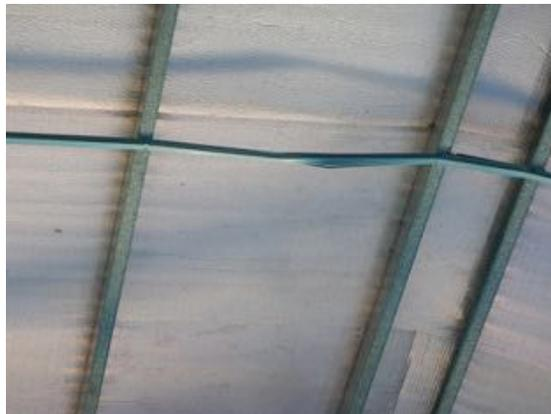
**Figure 4.47 Buckling of bridging elements**
