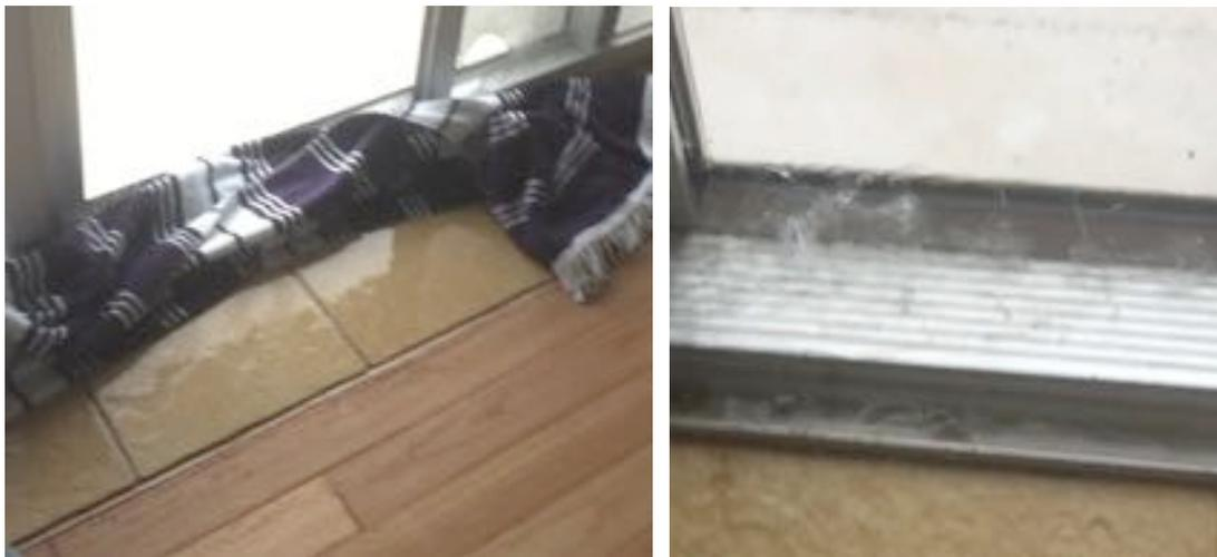
**Figure 5.1** Towels placed in front of large windward wall windows to control large amounts of water (*still photos from video by Shane Howden*)
