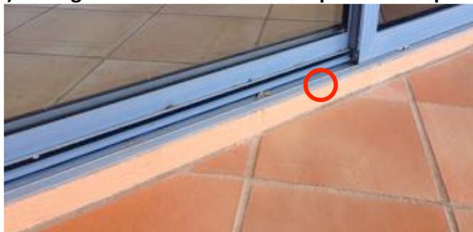
(b) Sliding glass doors with baffle that concealed the weepholes
