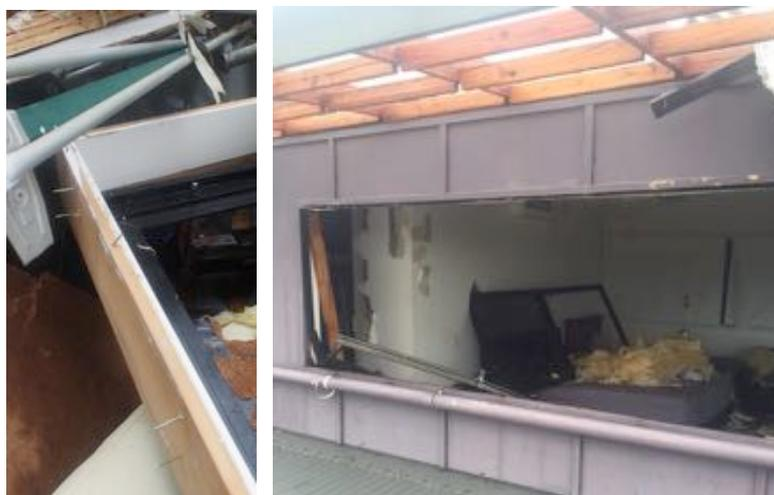
**Figure 4.26 Window frame blown from house frame
