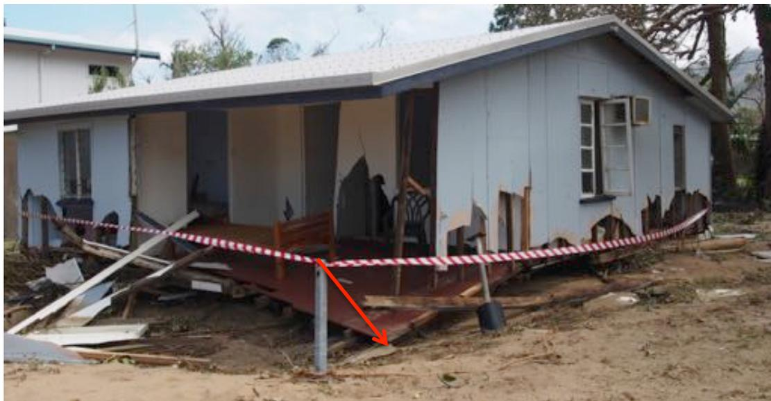
Figure 6.11 House pushed off stumps by storm surge
