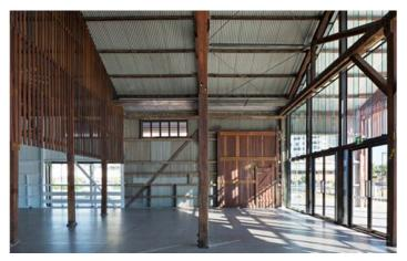
Removal of the lean-to structure yielded a substantial amount of Queensland maple, brown penda decking, and other structural timber members. The timber was recycled and used to build new timber pavilions, play structures and follies along the waterfront. The thick hardwood boards were planned on three faces to reveal the warm, dark hues of the native hardwoods, while the undressed external face was painted for weather protection using traditional methods.
