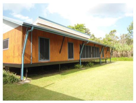
The cool breezes cross through the building, ventilating it and keeping it healthy. This passive design principle is called 'cross ventilation'.
