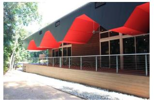
Much of the external wall cladding is extruded aluminium sheet with a decorative profile that is long lasting in the tropics, does not require painting and is easy to keep clean.
