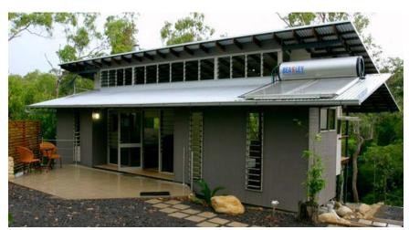
winter decks with a split roof form – was made into a rational design taking account of breeze paths, sun angles and functional space forms.
