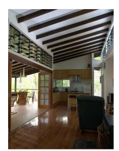
glazing from the high roof. The main roof falls down to the southern edge of the summer deck to maximise the shading from the summer sun, and to direct views down to the river.
