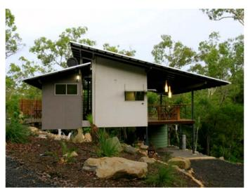
Power requirements are minimised through excellent passive ventilation, carefully designed shading to all glazed areas (supplemented by shade from the forest), and abundant natural light provided by the windows and amplified by the deliberately small footprint.
