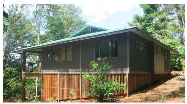
A high energy-rated 3 bedroom dwelling that was quickly constructed to minimize disruption to guests staying at the Rose Gums Wilderness Retreat. Using Jon Nott's newly patented wall fixing process FASTABUILD, the project was completed on-site in 3 weeks as the wall frames were assembled off-site the previous prior.
