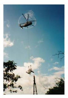
metre long lines, so that the blades never came close to the trees. The towers themselves were flown-in in sections and assembled on site; some tower sections weighed up to five tonnes each. The cableway haul rope was then laid and tensioned across towers by the helicopters.
