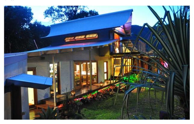
The house is long and narrow which enabled the principals of passive tropical design and making the most of the natural features of the site. Recycled timbers were used extensively throughout the project and the unnecessary use of materials was taken seriously. Soffit lining, fascias, trims etc are all eliminated.
