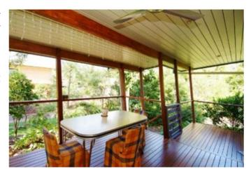
Site earthworks were kept to a minimum as a post and beam construction style was chosen negating the need to bench (flatten) the house site. This choice reduces the disturbance of top soils and the risk of soil erosion and run-off during the construction period.
