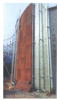
and stress in the fixings during large wind events. The cladding is mounted on substructure framing. The fixing spaces varied across the building and screw fixings and support framing was carefully detailed and electrically isolated to account for the diversity of the materials being employed.
