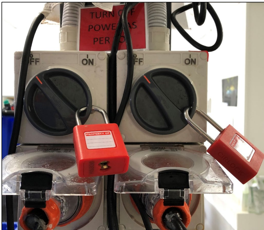
Figure 1. Before commencing any work with the water, turtles, or equipment, the electricity must be turned off and locked out. The electricity can be restored when all work is completed at the end of husbandry or project work.
