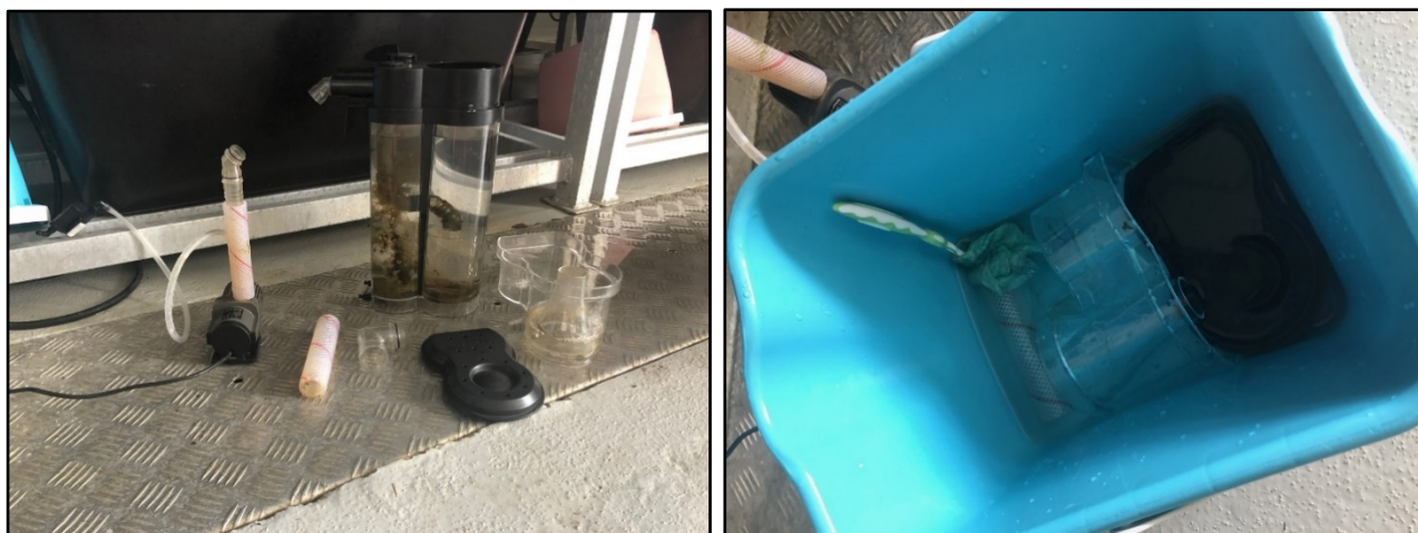
Figure 12. Disassemble the skimmer body and place foam cup, lid and outlet pipe in the system bucket to be cleaned.
