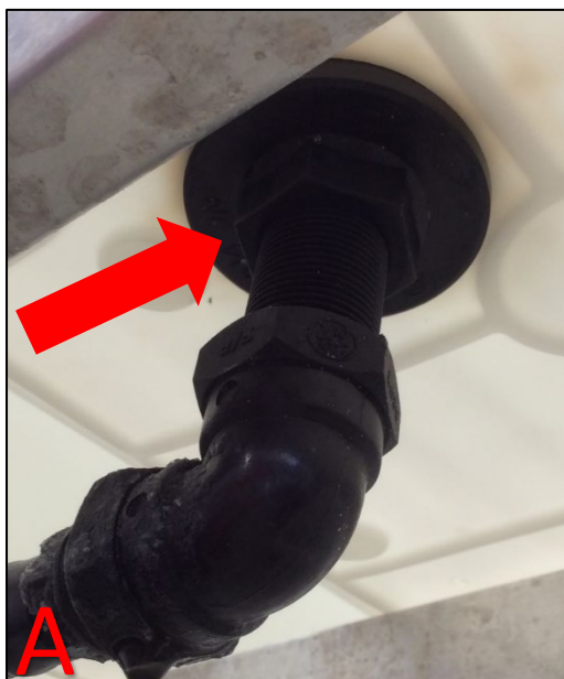
Figure 34. A) If the bolt comes loose, the tank may begin to leak. This is the part you need to hold when unscrewing the standpipe. B) Hold the bolt in place while unscrewing the standpipe during a water exchange.
