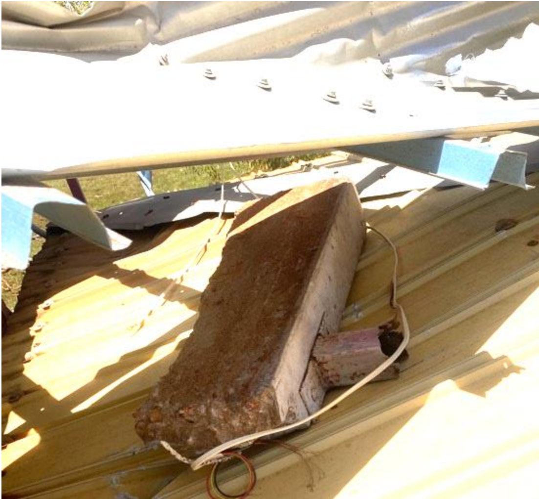
Figure 3-5 Footings still attached to the base of the veranda post after failure.
