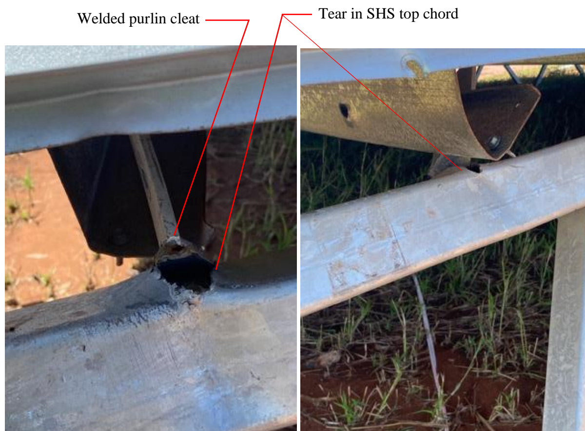
Figure 3-12 Torn SHS top chord at cleat plates.
