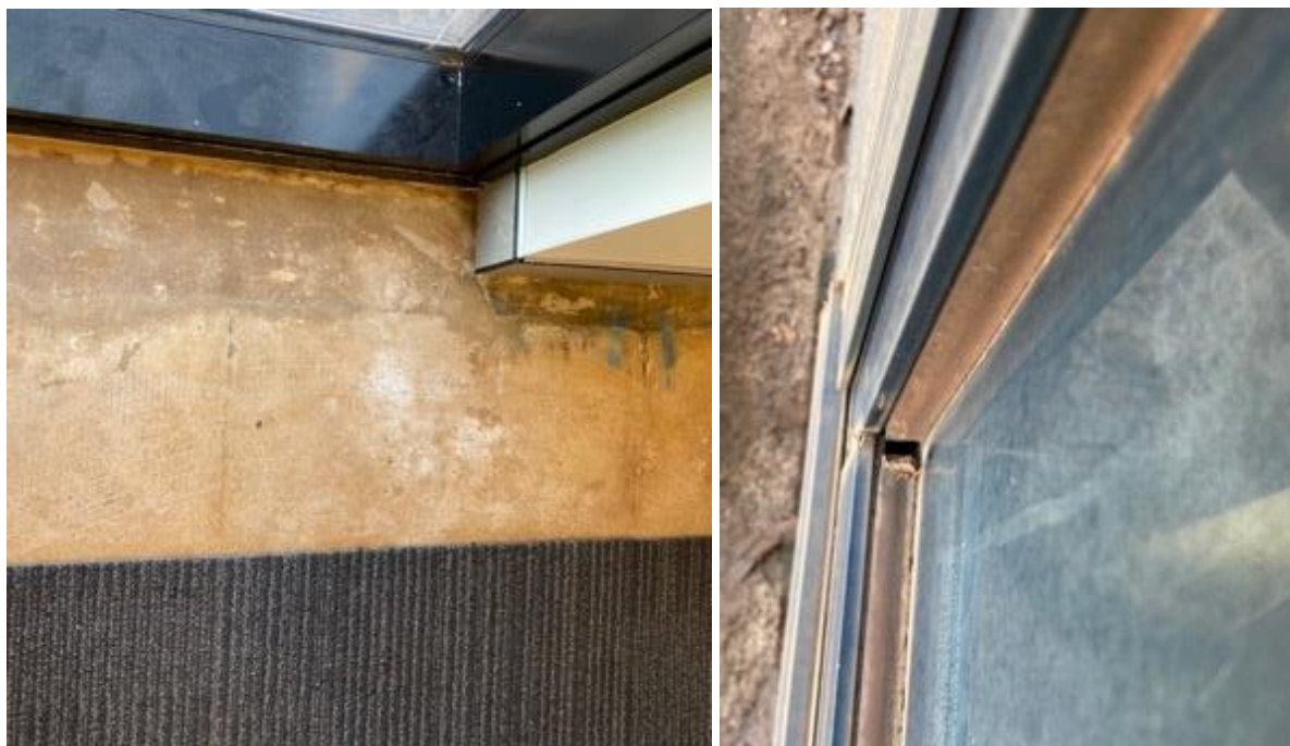
Figure 3-2 Water ingress through windows.
