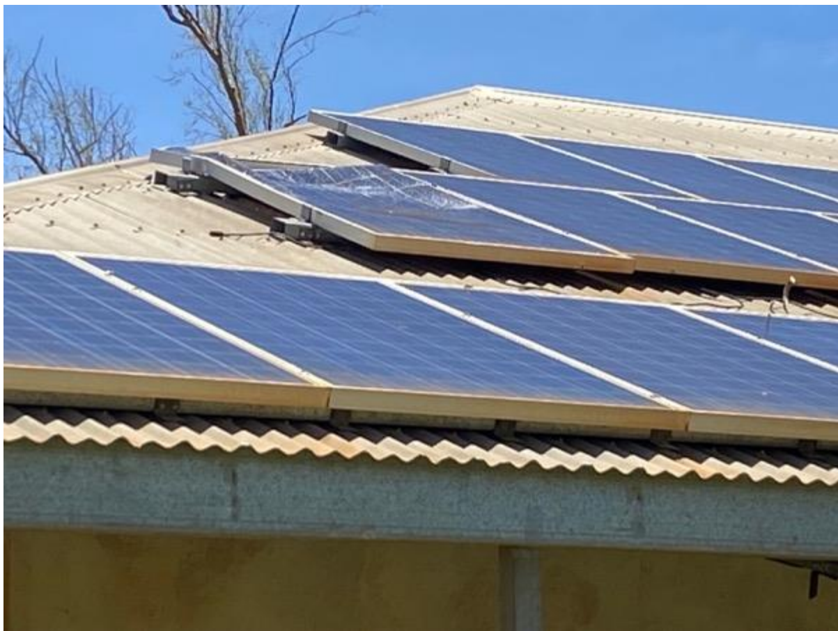
Figure 3-15 Debris damage to roof-mounted solar panels.
