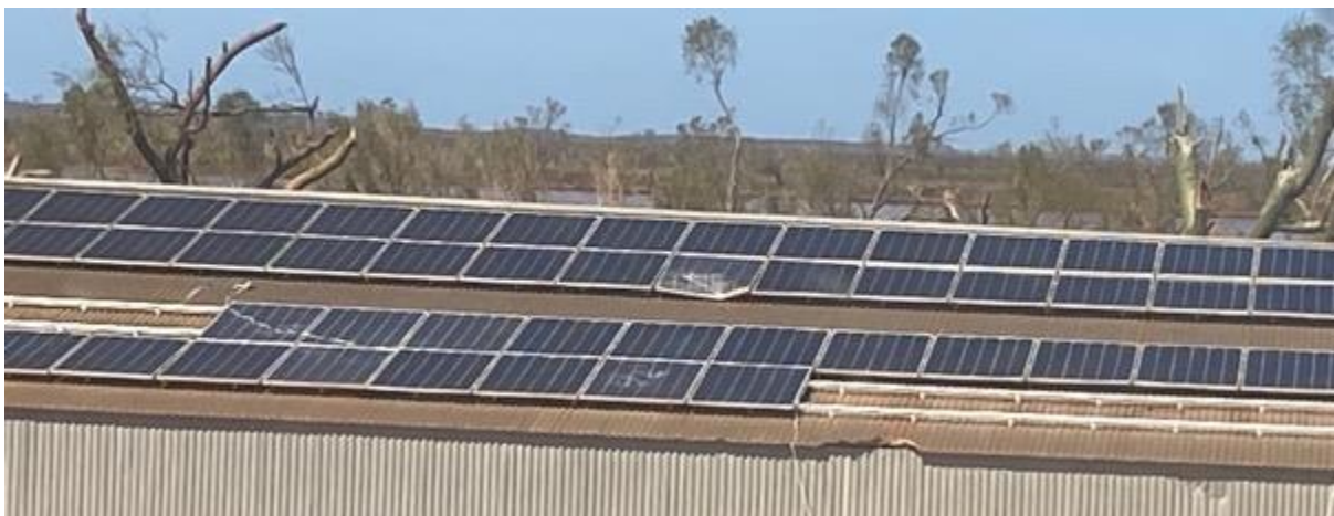
Figure 3-14 Missing roof-mounted panels due to clamp failure.
