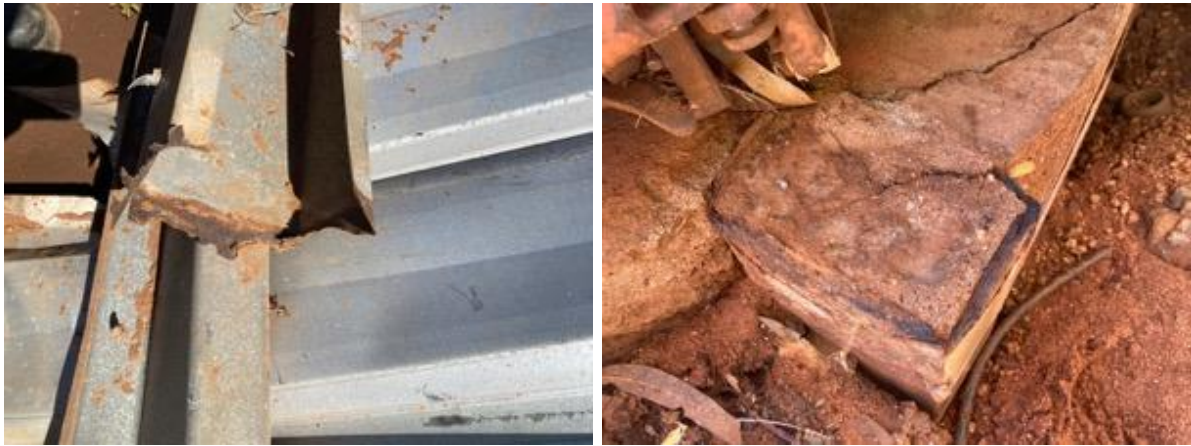
Figure 3-7 Corrosion at the base of the steel posts.
