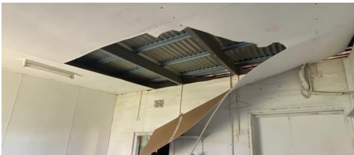
Figure 3-6 Water damage as a consequence of veranda loss.
