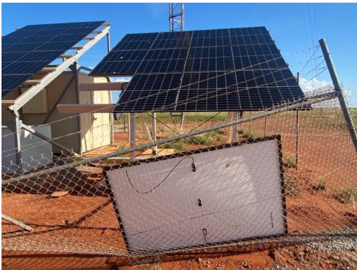
Figure 3-9 Failure of anchorage on ground mounted solar panels.
