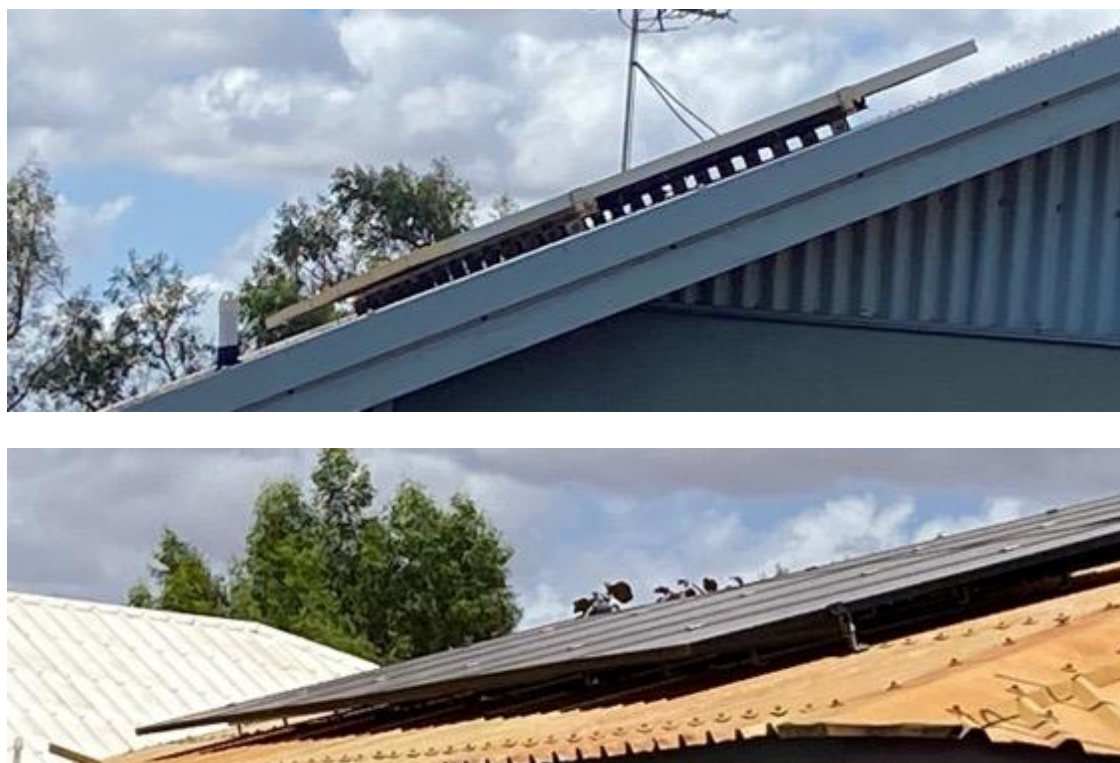
Figure 3-4 Varying frequency of L-foot brackets in roof-mounted solar panel systems.
