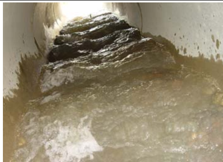
Two and one half standard baffle heights flow depth – looking D/S (11/04/06)
