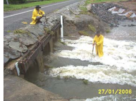
Velocity measurements on apron downstream of culvert fishway barrels (27/01/06)
