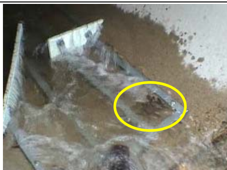
Glass perch resting at D/S end of offset baffle fishway – pipe Barrel 1 (28/01/06)
