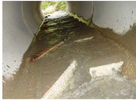
One standard baffle height flow depth – looking U/S (11/04/06)
