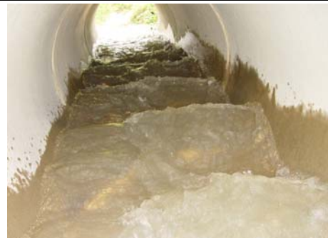
Two and one half standard baffle heights flow depth – looking U/S (11/04/06)
