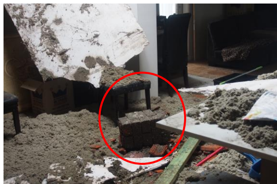
(c) Brick pillar (circled) inside dining room
