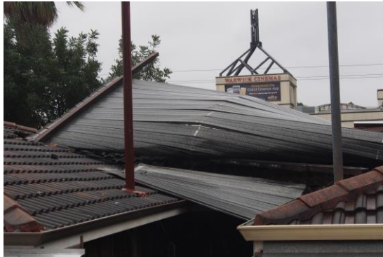
Secret-fixed roof sheeting on a carport became detached from its clips and folded back over the house roof
