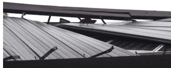
Secret-fixed roof sheeting on a carport became detached from its clips and folded back over the house roof
