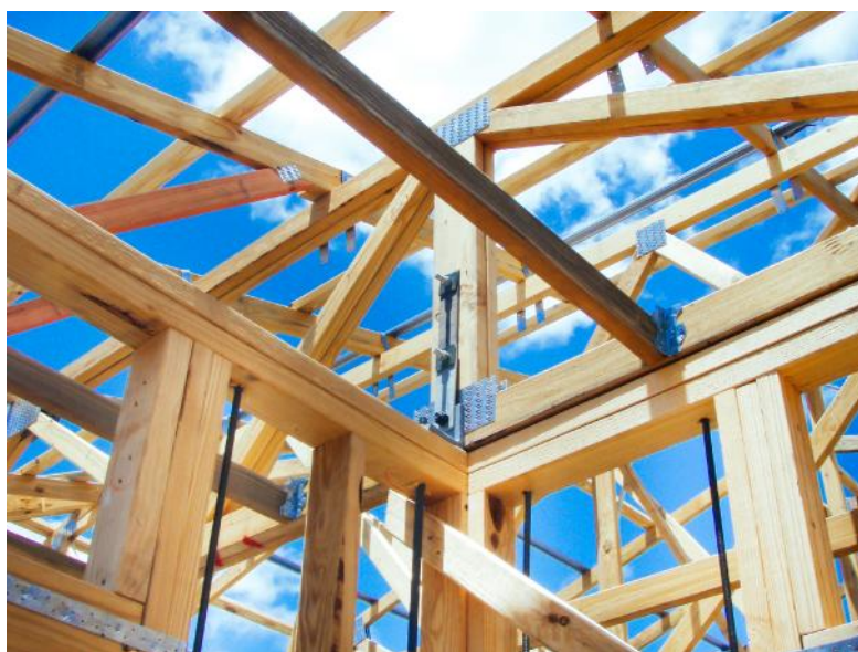
Cyclone rods installed during construction
