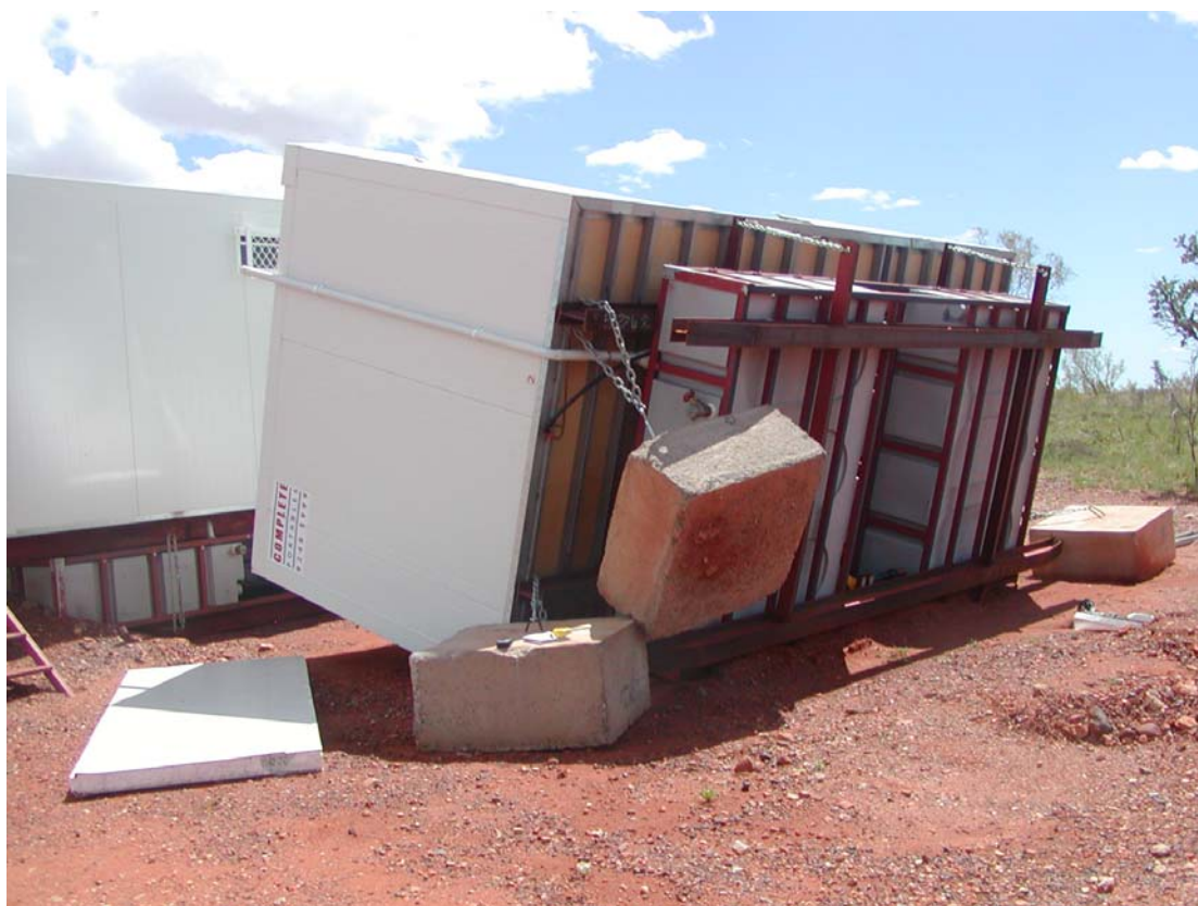
Figure 3.7 Overturned toilet block North of Rail Camp 1
