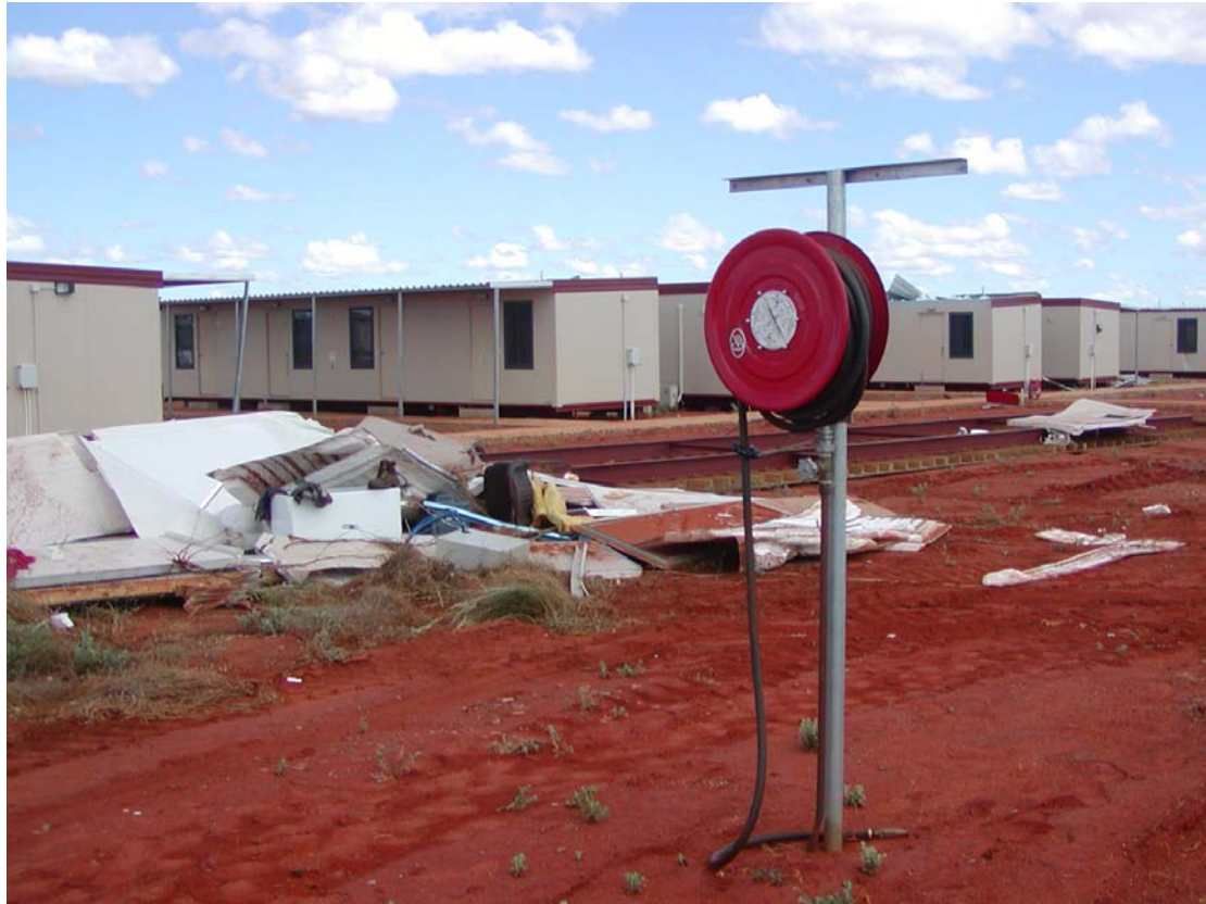
Figure 3.5: Hose reel at Rail Camp 1
