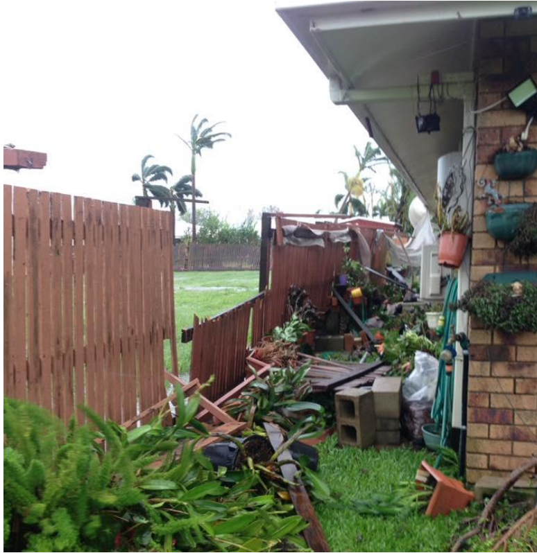
Figure 22. Damage to fencing in Proserpine
