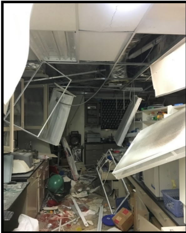
The remains of the steel tank at the site of the explosion.
