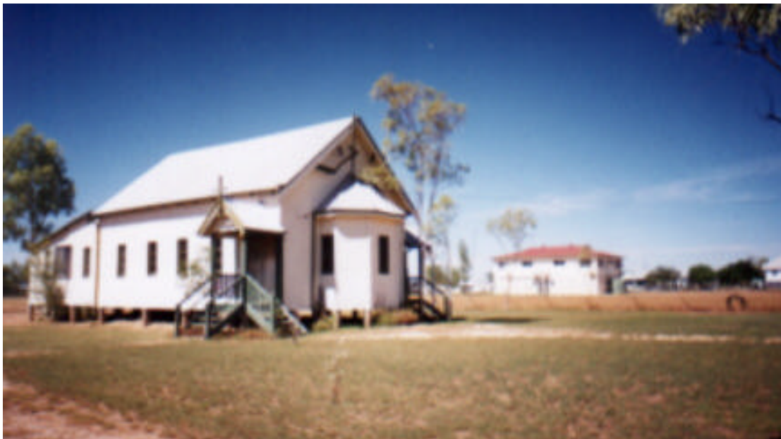
Photo: Julia Creek Uniting Church (David Ireland 2001)
