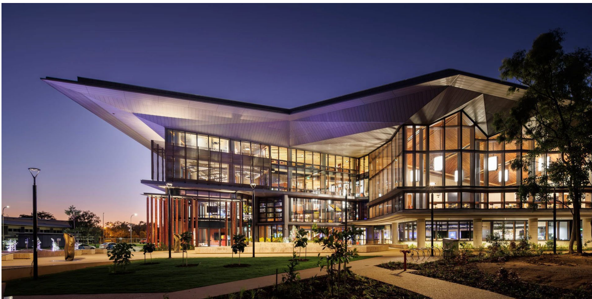
Image by James Cook University The Engineering and Innovation building lit up at night with a purple sky behind Dec 2024
