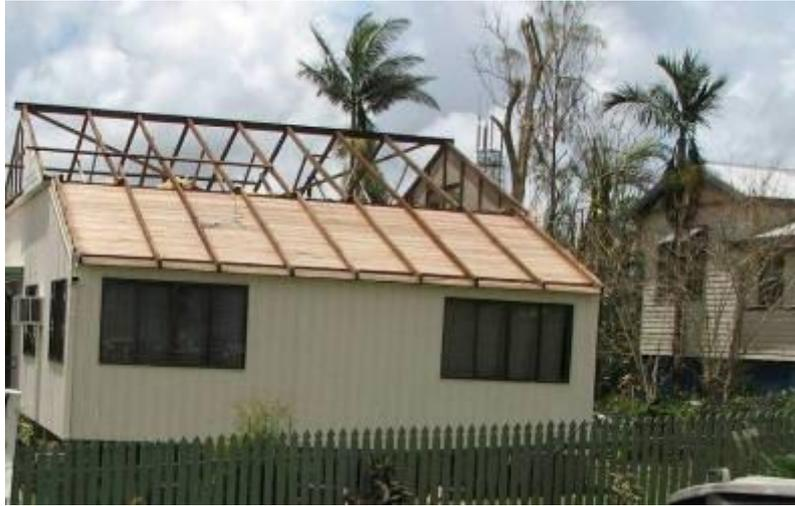
**Figure 3.12 Batten loss**
