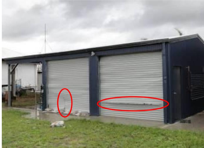
**Figure 3.29 Failure of door curtains under repeated combined bending and tension loads**
