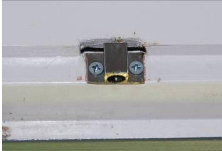
**Figure 3.6 Door keeper connections not strong enough
