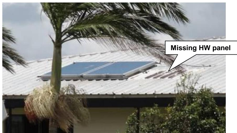
**Figure 3.70 Solar hot water panels**
