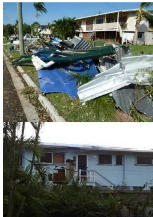
Debris and wind driven debris damage
