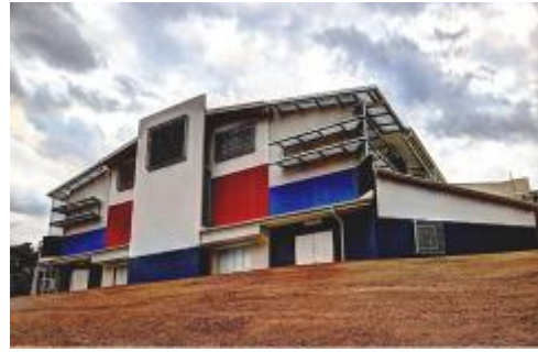
Queensland Community Cyclone Shelter under construction in Bowen
