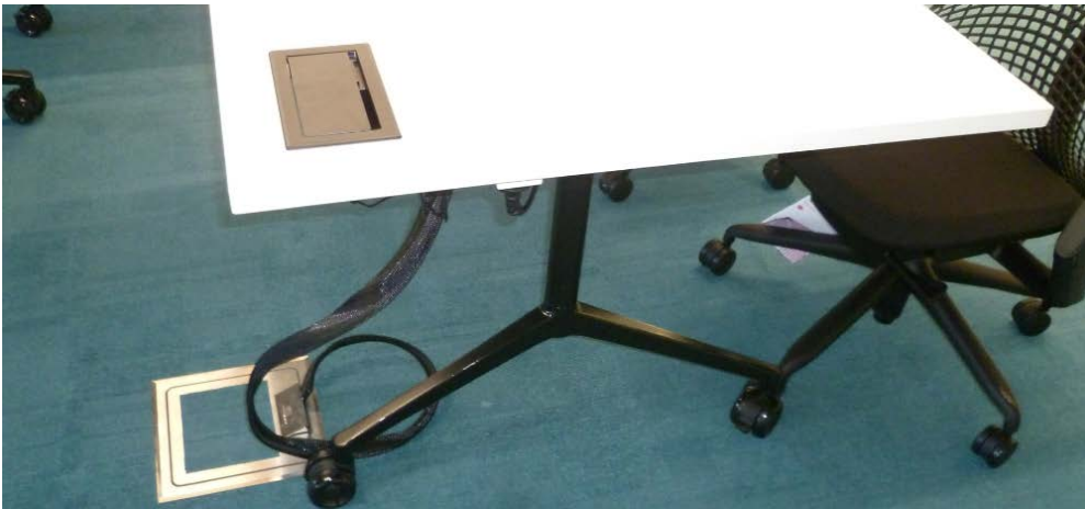
Image above showing correct location of Judge's Table 1 in relation to the floor box.
