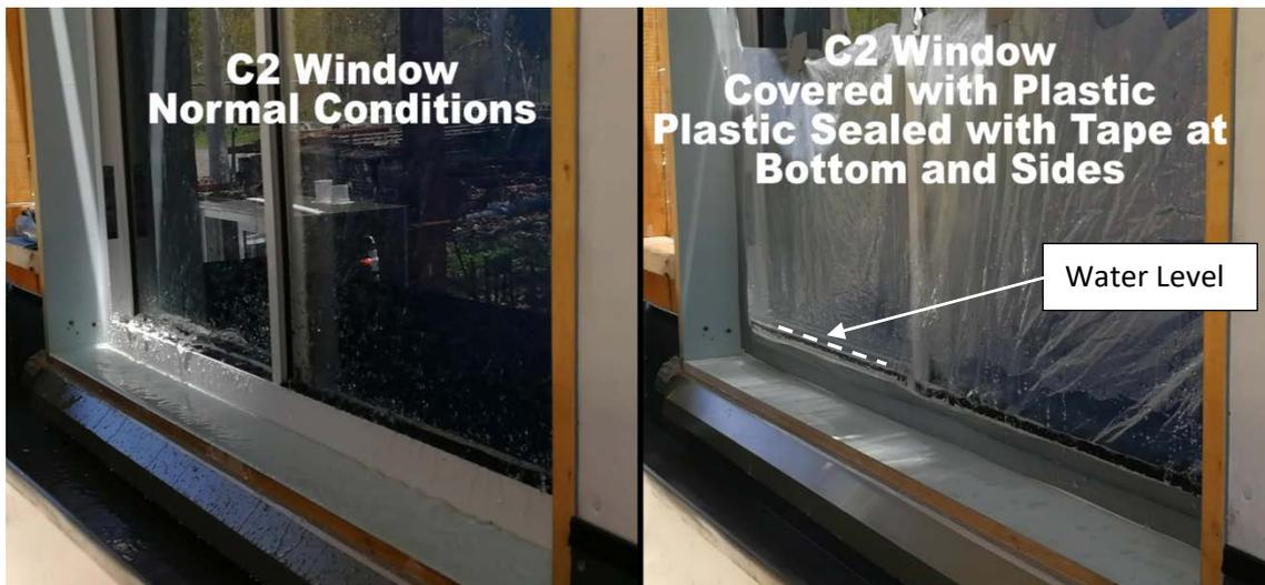
Despite this set-up some water can still leak through the tape or from above the window, you can place a towel on the window sill to absorb this water **before** the cyclone.
