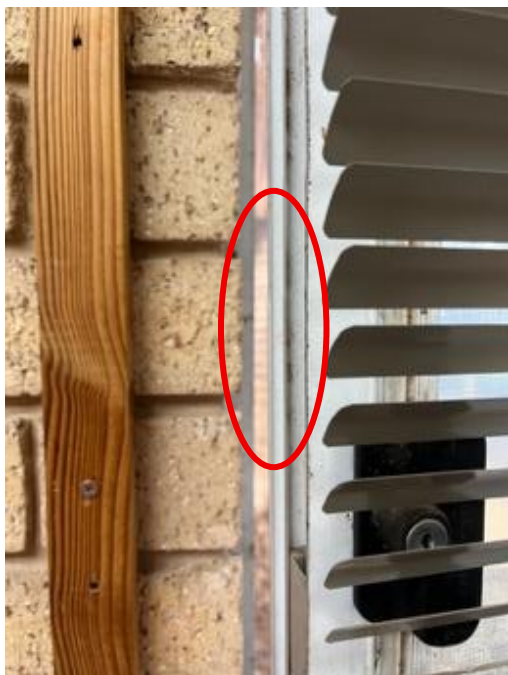
(a) Frame moved from brickwork
