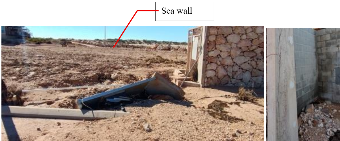
Figure 7-3 Marine debris washed more than 40 metres from sea wall
