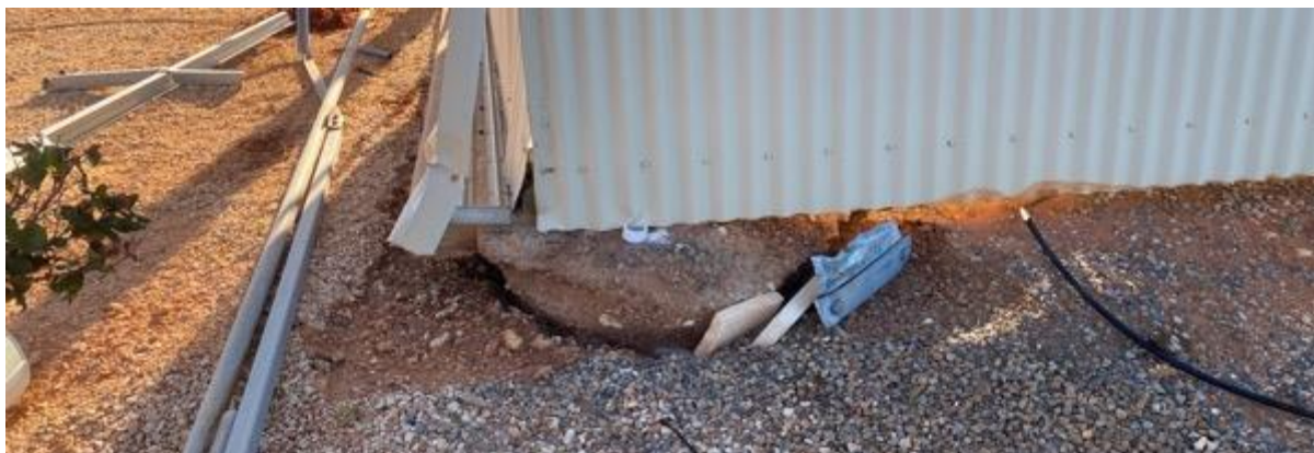
Figure 6-7 lifting of footing under an end portal leg
