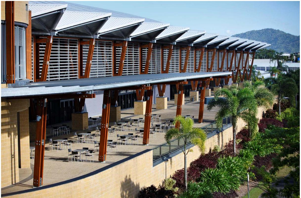
The proposal for the building of the Cairns Convention Centre was the outcome of a collaborative response to a design competition to construct Australia's first environmentally planned major public building. The Centre's iconic double pleated roof is not only geometrically striking, providing a visual reference on arrival to the city of Cairns, but captures the seasonal tropical downpours, channelling rain water directly into storage.
