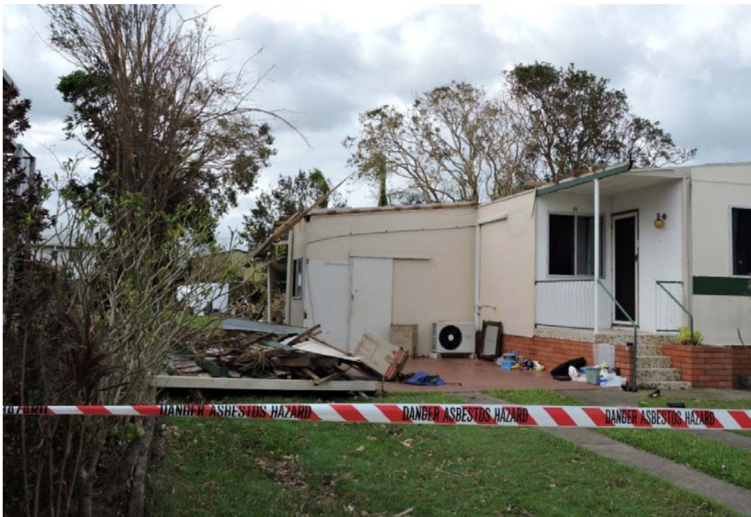
Figure 13. Asbestos identified as a further hazard in damaged housing, Proserpine
