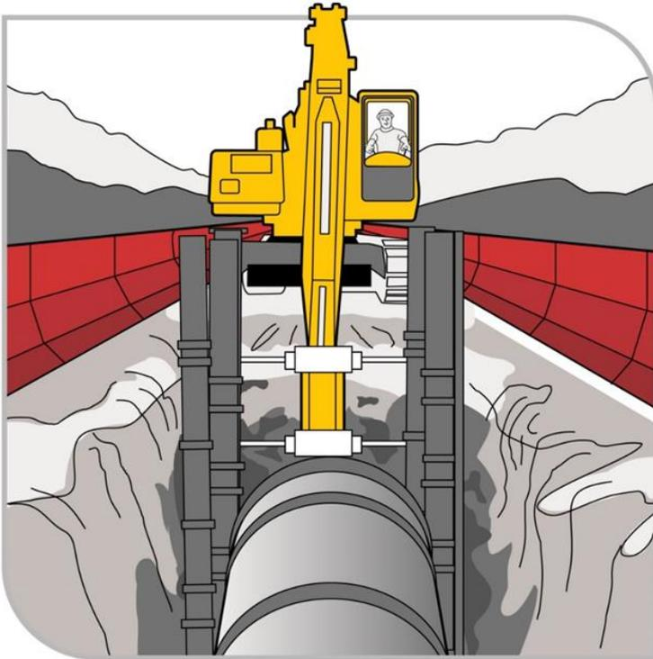
**Figure 6** Extending trench shields above the excavation
