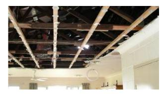
Increase in wind speeds due to speed up over steep topography did cause increase in damage to buildings. This was more apparent in the older housing. However there were a few cases of damage to contemporary houses, where the construction details were inadequate for the site topography. This highlights the need for each building site to have the topographic wind speed modifiers (AS/NZS1170.2, or AS4055) correctly specified.
