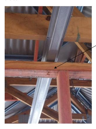
Internal partition wall restrained at top by gun nails fired into metal ceiling batten.
