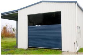
House near Mission Beach undamaged except for garage door failure. Shed also with failed roller door.
