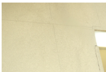
Figure 4-26 Movement cracks at panel joints
