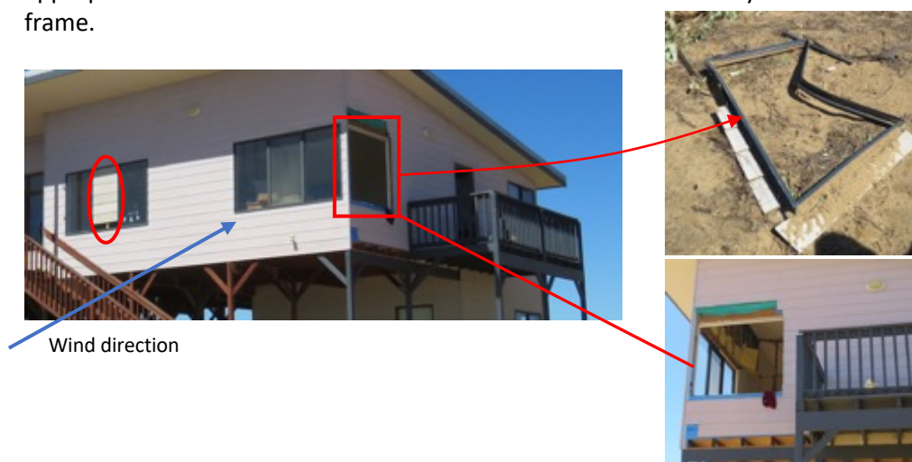
Figure 4-28 Loss of complete side window after a windward wall window broke
