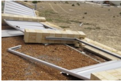
(a) Reinforced pillars with sheet steel infill panels
