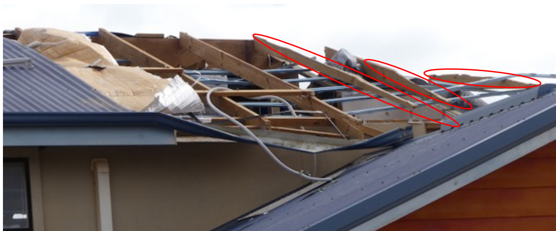
(c) Failure of rafters
