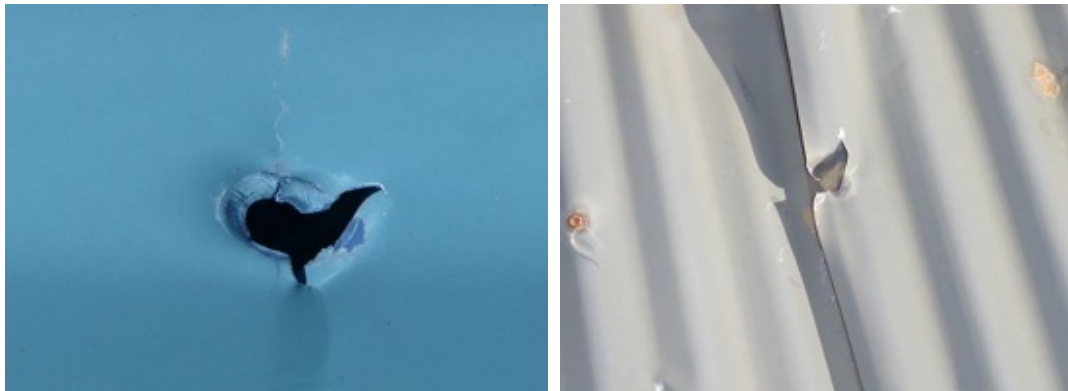
Figure 4-18 Failures in roof sheeting by fastener pull-through
