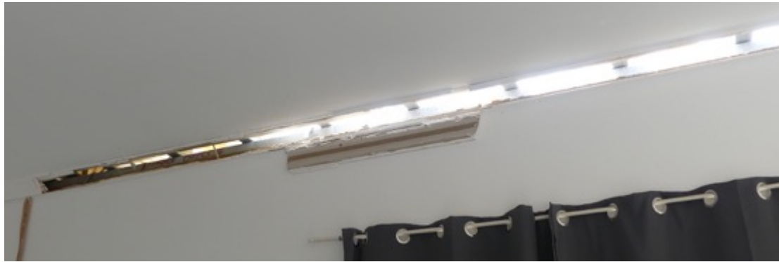
(a) Roof partially lifted off external walls
