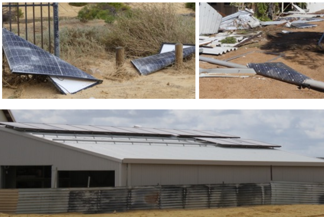
Figure 7-9 Damage to solar photovoltaic panels
