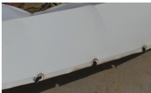
(a) Flashings fastened too close to the edge
