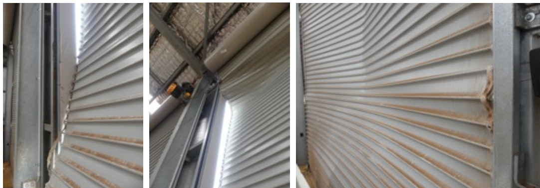
Figure 7-3 Damage to large access roller doors – View from inside shed
