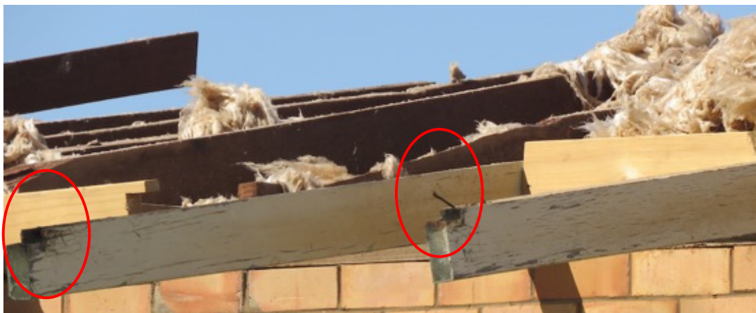
Figure 5-6 Rot in exposed rafter ends
