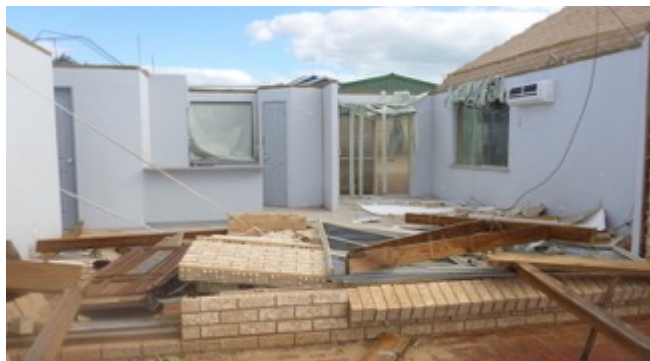
Figure 4-24 Failure of a wall with large openings
