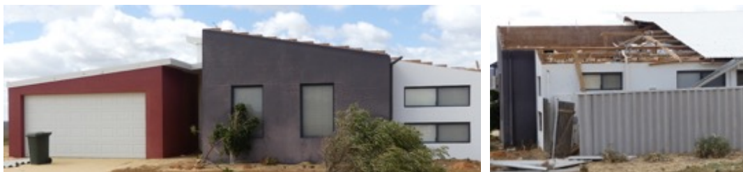
Figure 4-10 Failure of a skillion roof at the roof to wall connection
