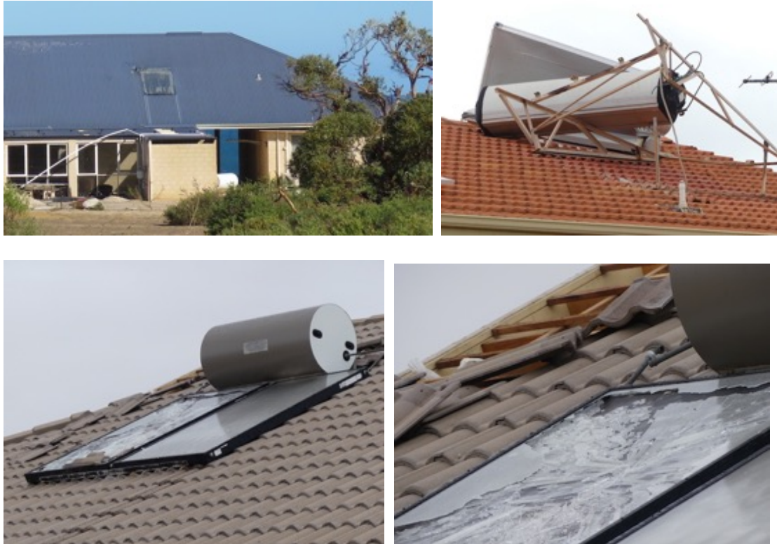
Figure 7-10 Damage to hot water systems
