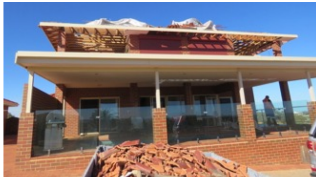
Figure 4-20 Loss of tile battens and roof tiles
