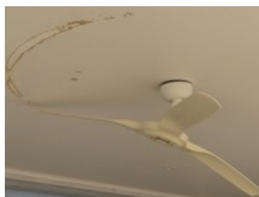
Figure 7-8 Damage to outdoor ceilings from ceiling fans
