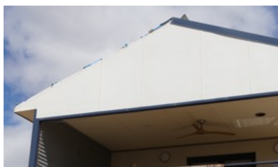
(b) Fasteners installed too far apart
