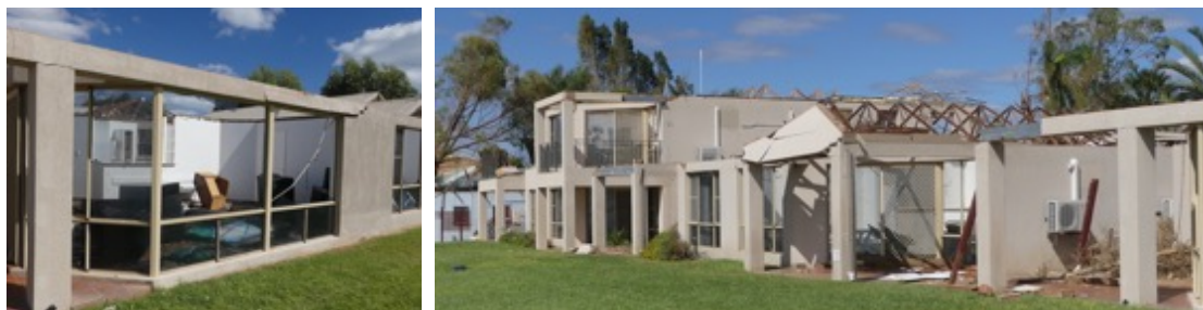
Figure 4-13 Refurbished buildings with broken windows and substantial roof loss
