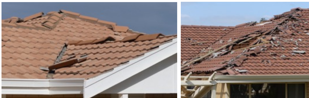
Figure 4-19 Examples of damage to ridges and hips on tile roofs
