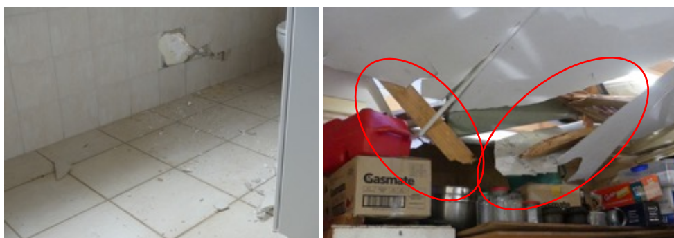
Figure 4-4 Examples of wind-borne debris damage to houses
