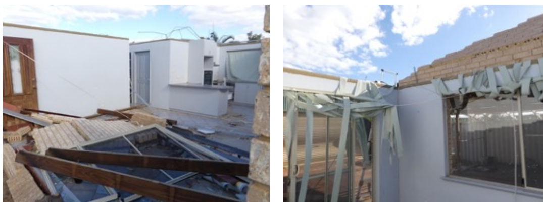
Figure 4-8 Loss of roof structure due to the withdrawal of tie-down straps
