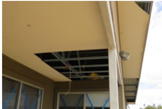
Figure 4-36 Damage to eaves linings
