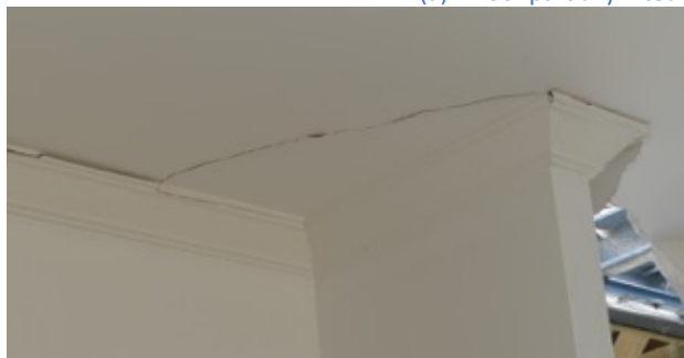
(b) Roof partially lifted off internal walls
