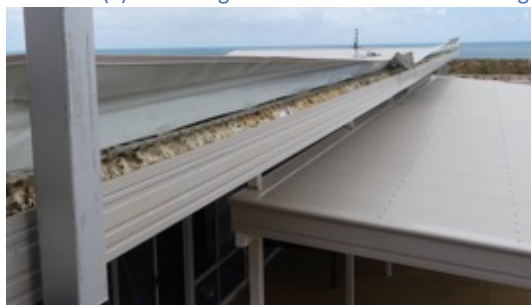
(c) Flashings fastened with pop rivets
