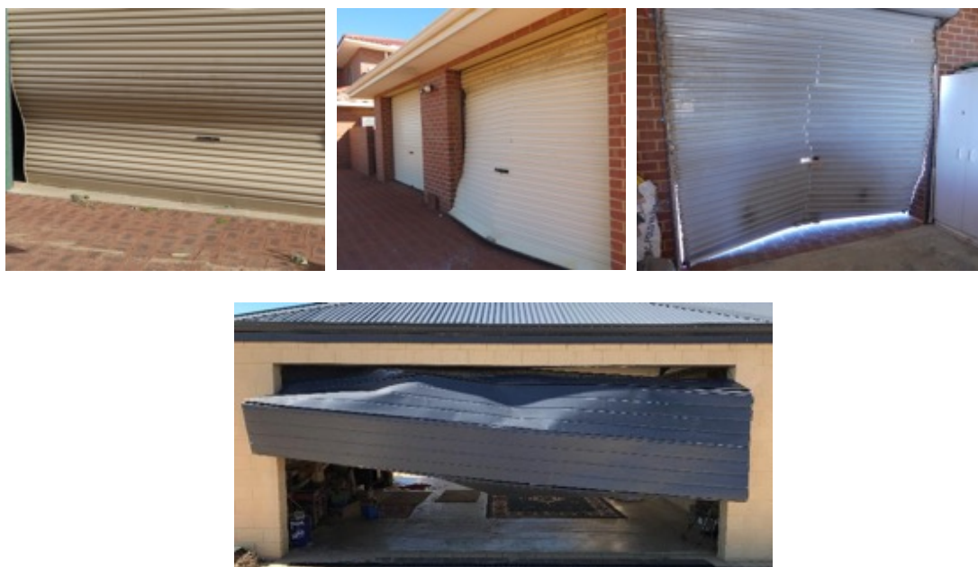
Figure 4-33 Failure of garage doors in Kalbarri
