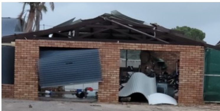
Figure 4-34 Failure of garage doors in Geraldton
