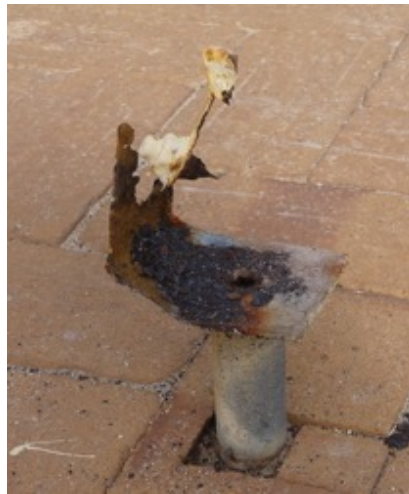
Figure 5-5 Corrosion in stirrups for veranda posts
