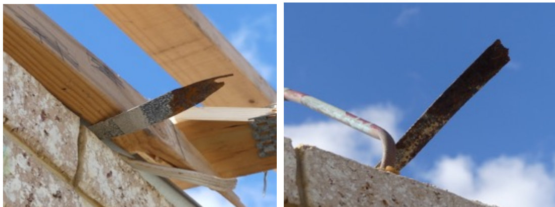
Figure 5-3 Corrosion in tie-down straps that led to the loss of timber-framed roofs
