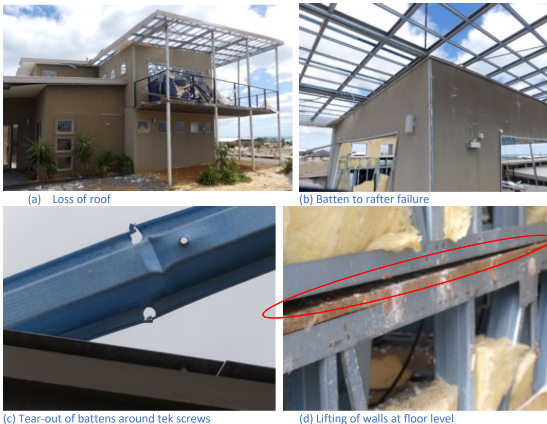
Figure 4-14 Failure of a skillion roof at batten to rafter connections
