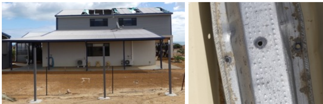
Figure 4-15 Failure of batten to rafter connection by the withdrawal of tek screws
