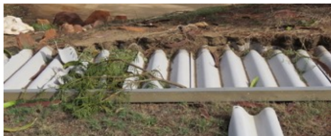
Figure 7-7 Damage to fibre cement fences
