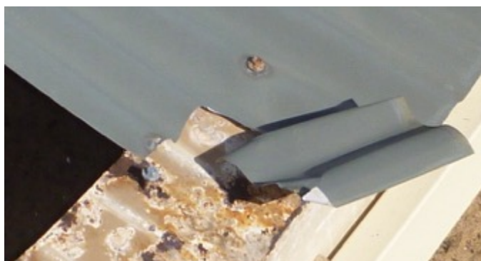
Figure 5-4 Corrosion of flashings and fasteners
