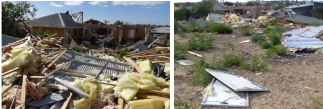
Figure 4-9 Roof loss following the failure of garage doors
