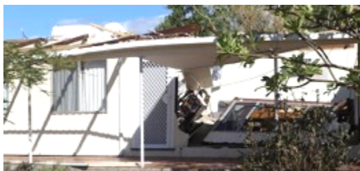
Figure 5-2 Broken windows leading to failure of the roof structure in an older house
