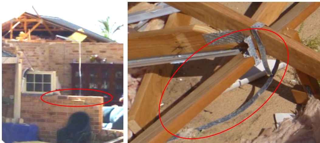
(a) Failure of brickwork at embedment depth (b) Tie-down strap attached to roof members
