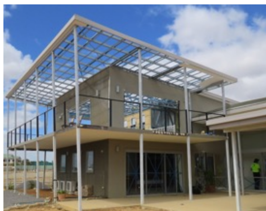
Figure 9-2 Roof loss and damage to walls
