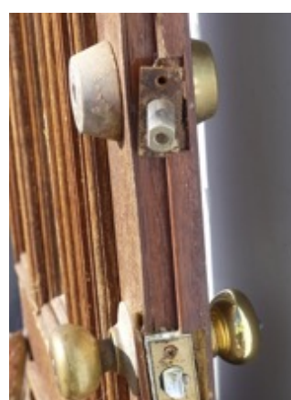
(b) Door latch failure
