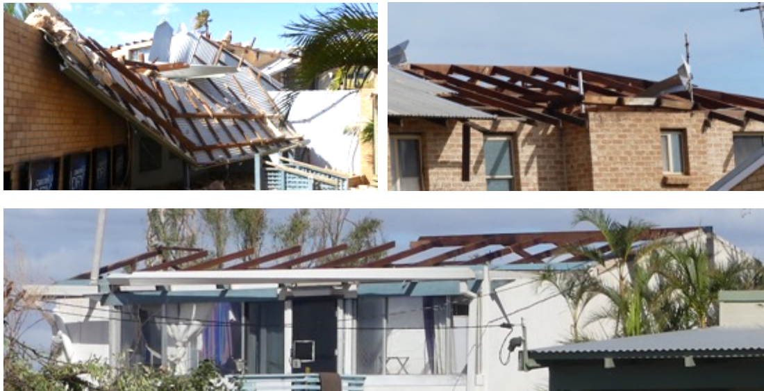
Figure 5-7 Failure of nailed batten to rafter connections or skew nailed rafter to wall connections
