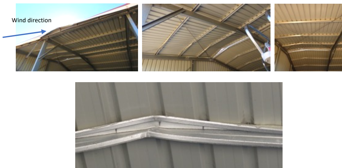
Figure 7-1 Damage to purlins in a large shed
