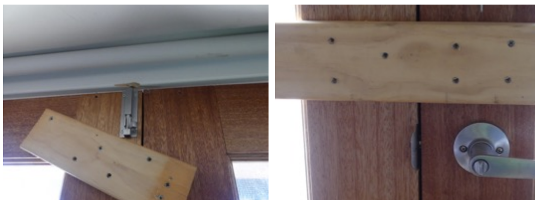
Figure 4-32 Temporary brace on the double front door
