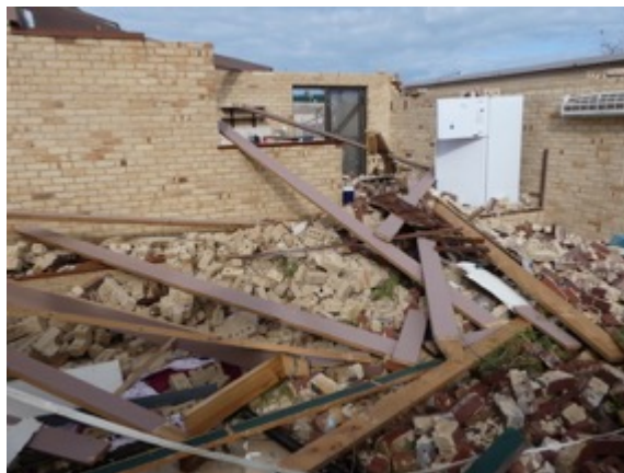
Figure 4-22 Failure of a windward wall under wind actions.
