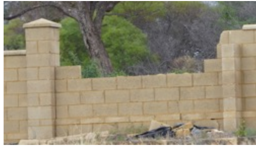
(b) Reinforced pillars with unreinforced blockwork
