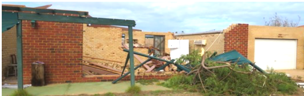
Figure 4-7 Loss of timber-framed roof due to failure of tie-down straps in brickwork
