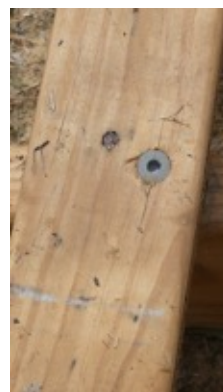
(b) Screws at base of rafter
