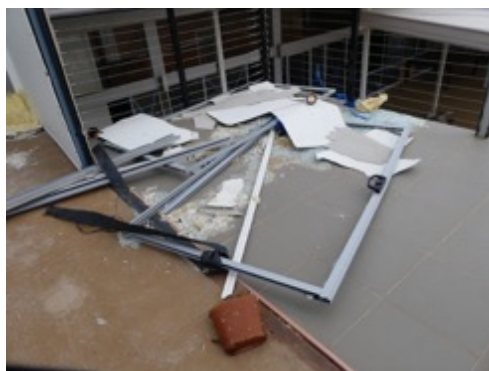
Figure 4-29 Detachment of glass sliding door frame under wind loads
