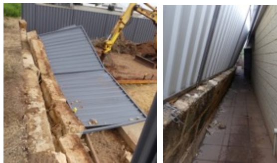
Figure 7-6 Damage to retaining walls caused by wind loads on attached fence panels
