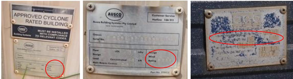
Figure 7-3 Wind rating plates on dongas
