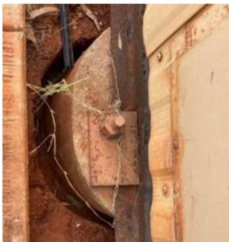
Figure 7-11 Clamped donga anchorage
