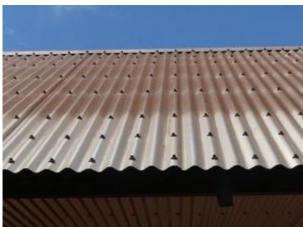
Figure 8-1 Roof with closely-spaced fasteners performed well
