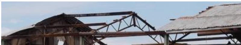
Figure 6-4 Deterioration of timber in shed elements
