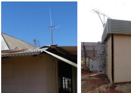
Figure 8-11 Examples of aerials that performed well during TC Ilsa
