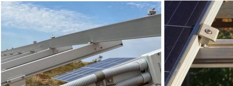
Figure 5-8 Clamps that have released the panels
