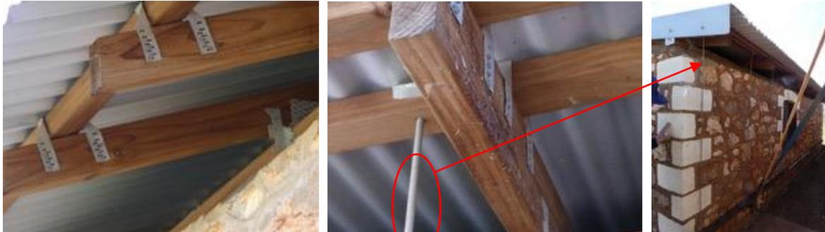
Figure 8-3 Upgraded tie-down connections on a heritage building
