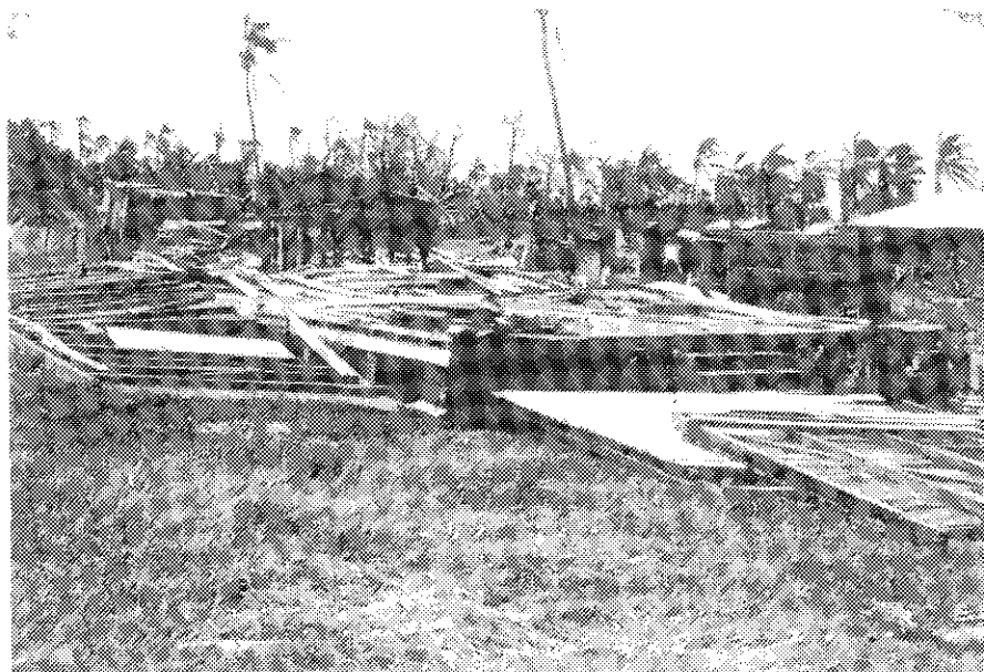
Figure 13. Walls blown clear of floor.
