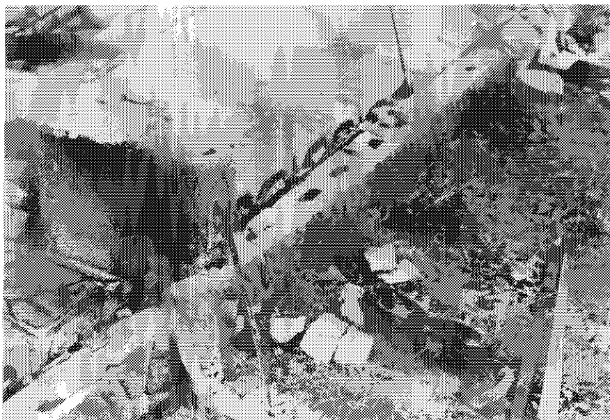
Figure 19. Wall failure due to insufficient bond strength.
