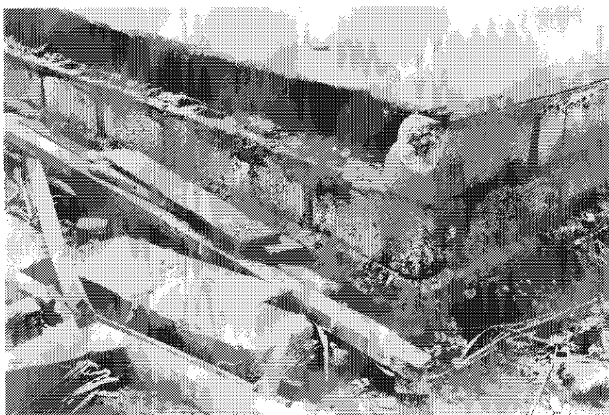
Figure 5. Typical floor slab for domestic construction. Note nominal thickness of concrete.
