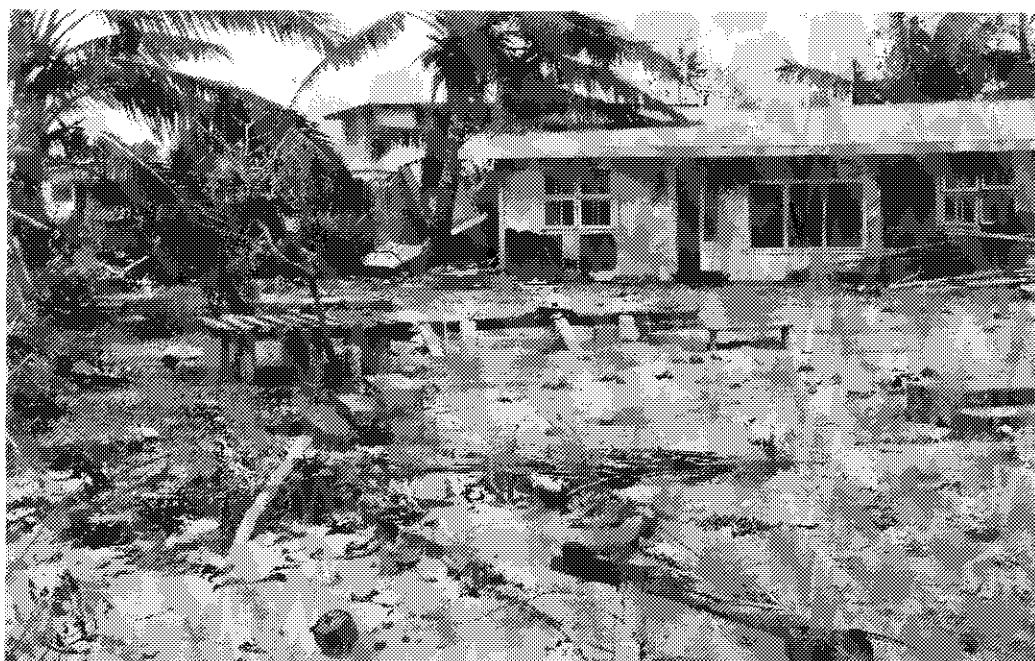
Figure 23. House washed from stumps by storm surge.
