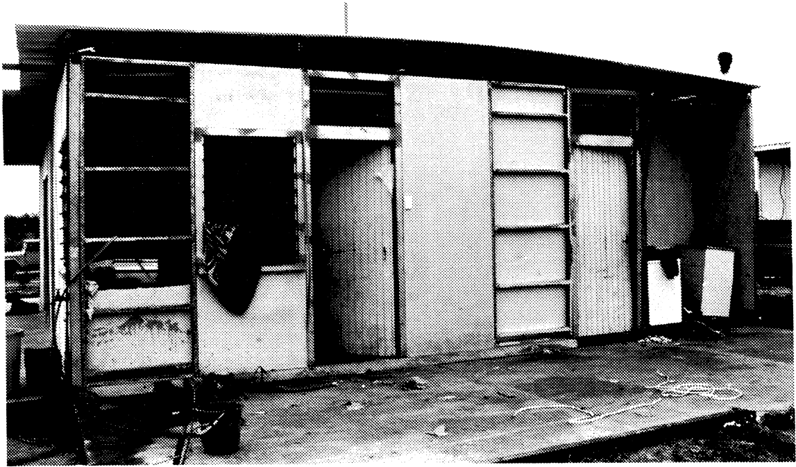
Figure 19 This steel framed aboriginal house lost some external cladding, and a large open verandah.
