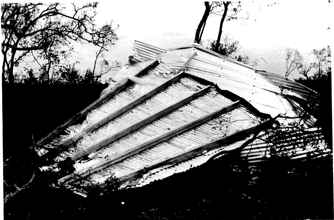
Figure 12 This complete roof structure was removed from its house causing almost total loss of walls.
