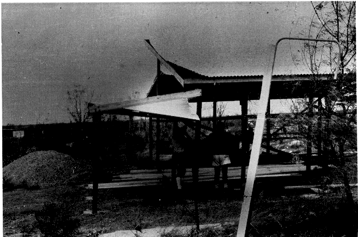
Figure 26 Partially completed house showing racking of the frame
