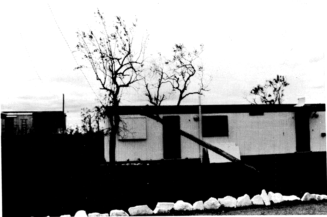
Figure 13 The tie down facility of this ATCO transportable prevented overturning.
