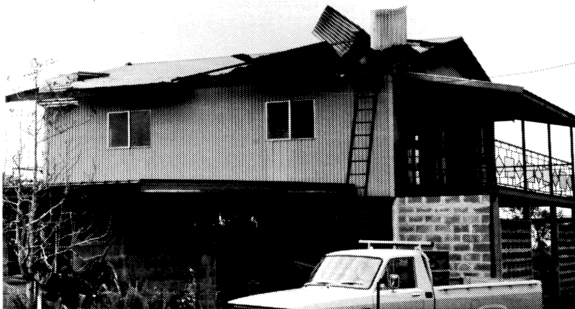
Figure 8 Roof damage near corners.
