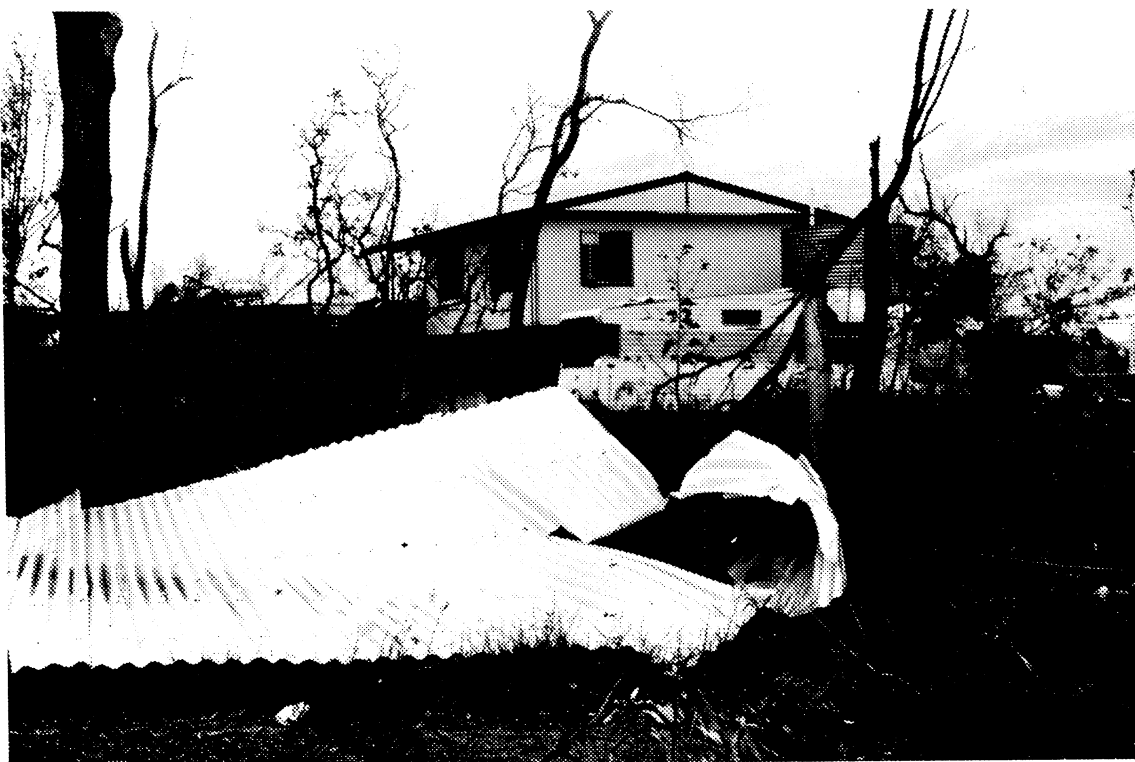
Figure 7 This carport was removed from the otherwise undamaged house in the background.
