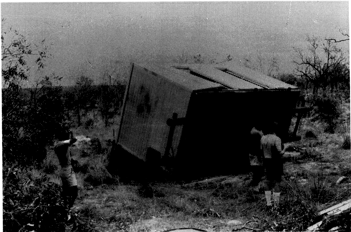
Figure 14 This transportable had no restraint against overturning - it had only just been positioned on site.
