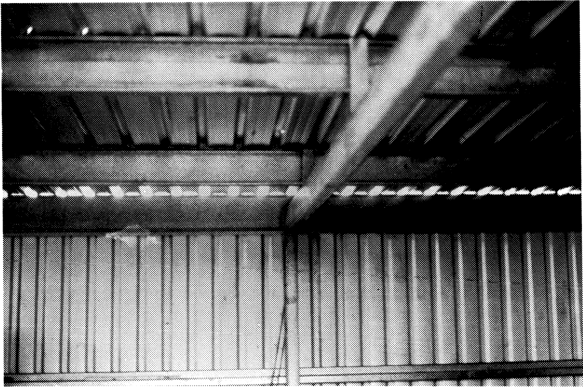
Figure 24 View inside light gauge steel building showing total lack of bracing members.
