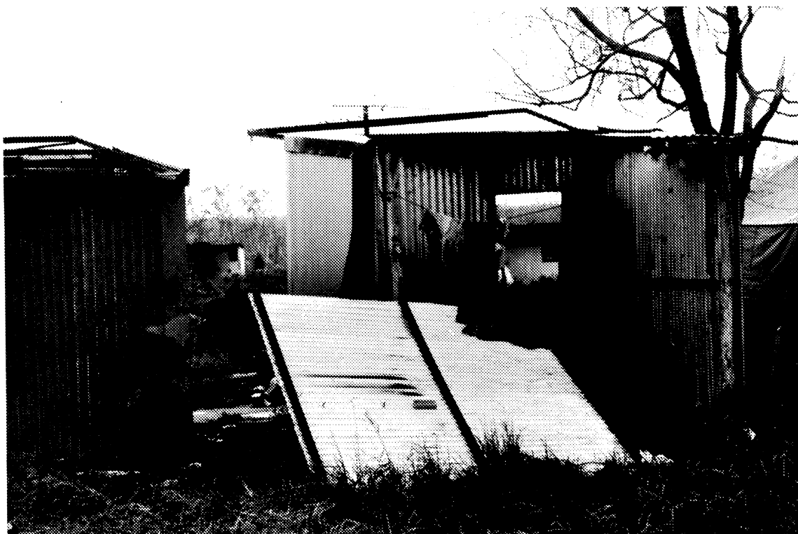
Figure 23 An almost identical building totally destroyed - Verandah and dominant openings on windward side.
