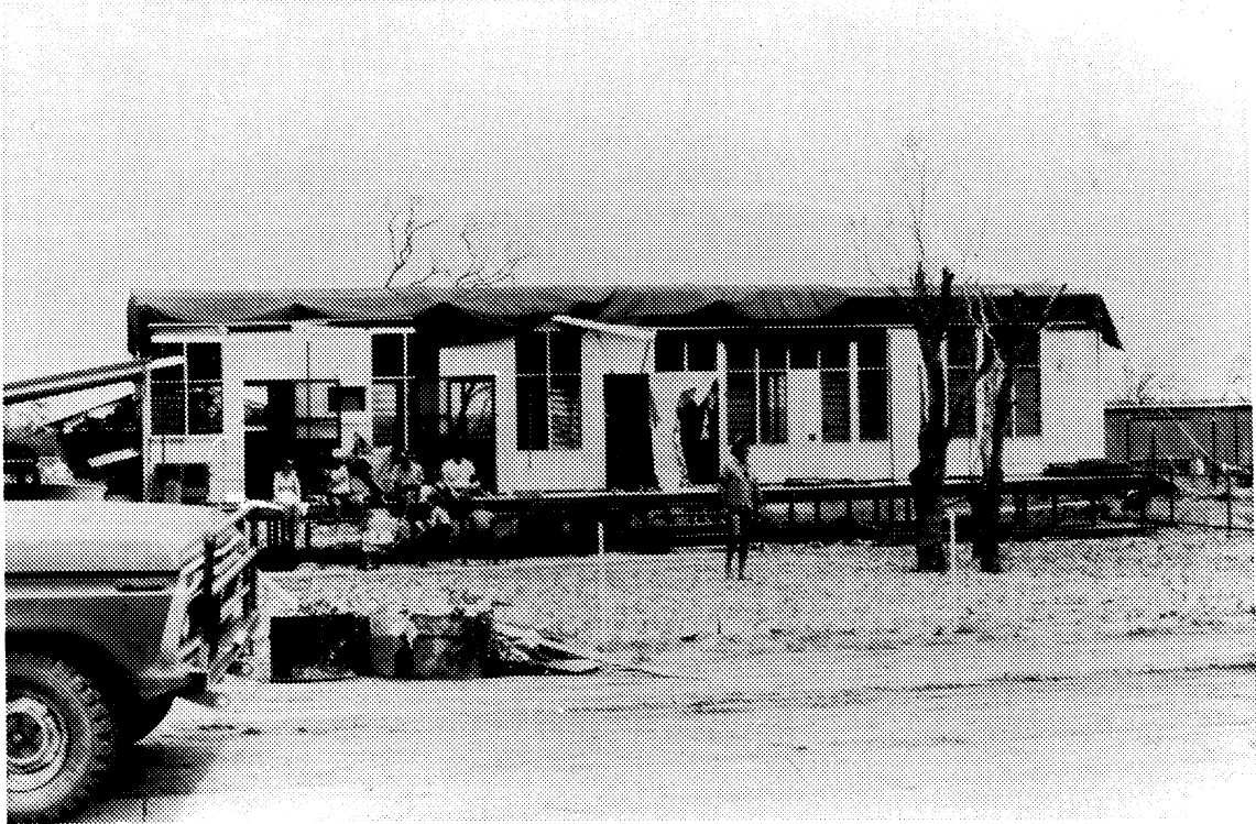
Figure 11 Recently transported house from outside cyclone area lost its roof structure.
