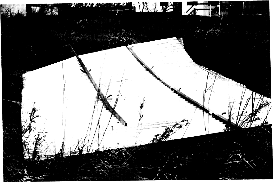
Figure 9 Roof panel removed with sheeting still attached to battens.
