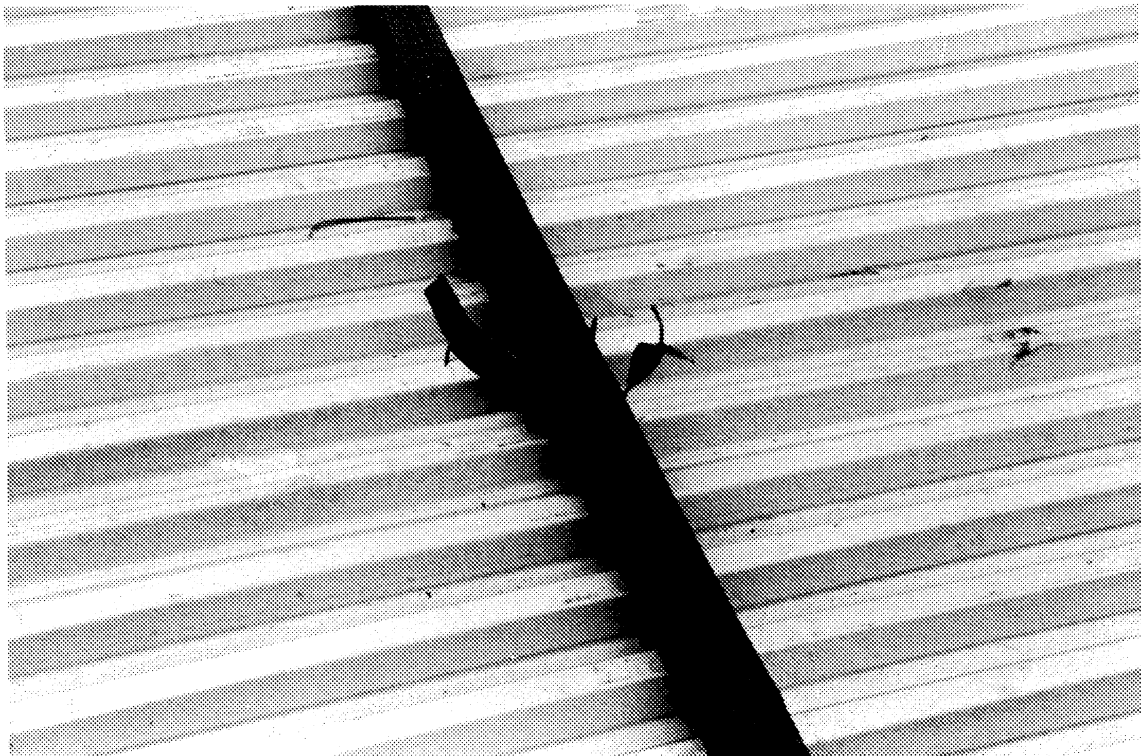
Figure 10 Detail of same panel showing one nail through batten and only one nail in each end of the strap.
