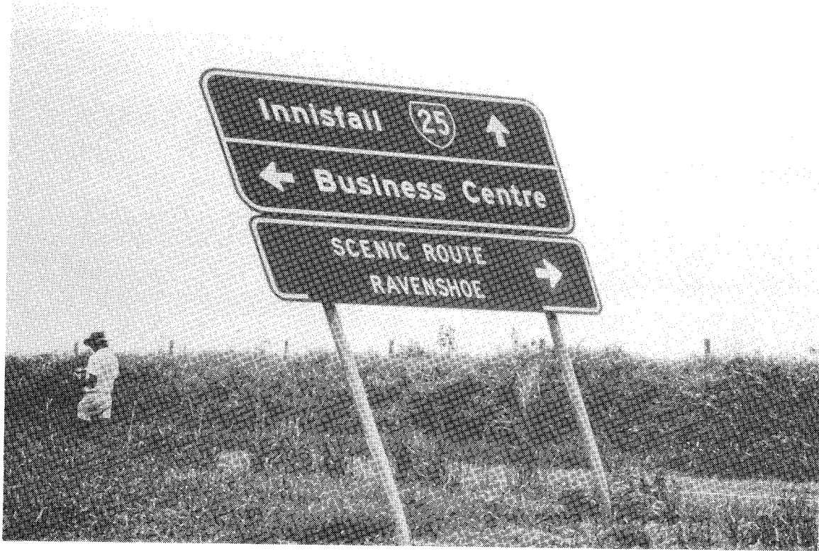
Figure 9. Road Sign Bent by Wind Forces
