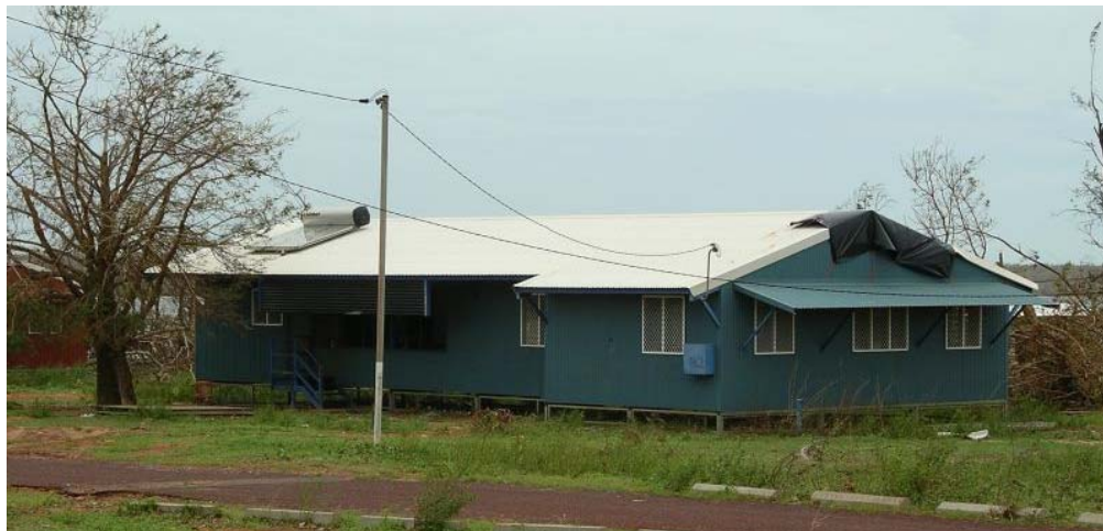
Figure 11: Minor loss of flashing
