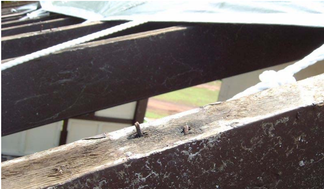
Figure 28: Corroded and inadequate batten fixings
