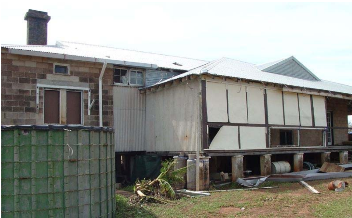
Figure 35: Loss of guttering, fascia and awnings at Cape Don (photo from DIPE)
