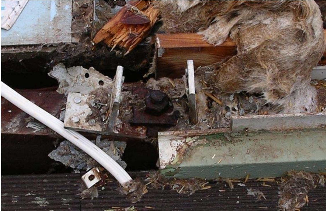
Figure 20: Aluminium inverted T brackets and rusted hold down bolt
