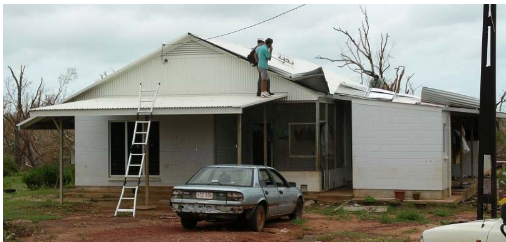
Figure 12: Roof structure damage to new house (windward wall)
