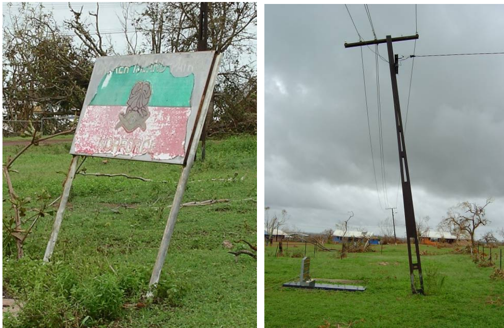
Figure 5: Footing failures - poor ‘windicators’
