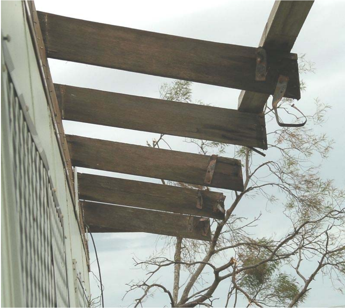
Figure 16: Corroded batten hold down straps
