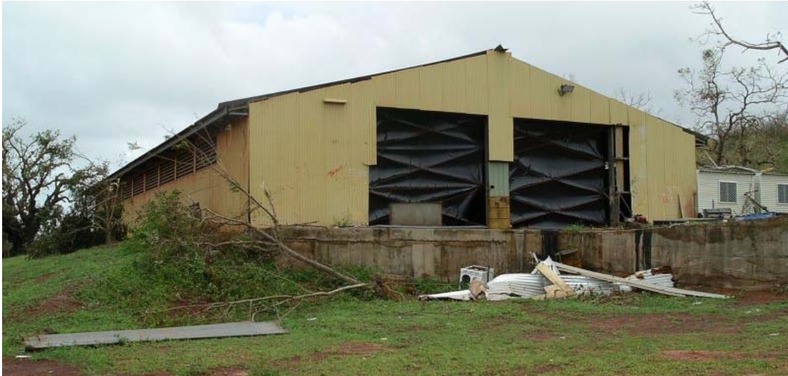
Figure 24: Wind ward wall (North face) Note openings have been covered with plastic
