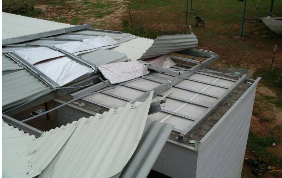
Figure 13: View of damaged roof on new house
