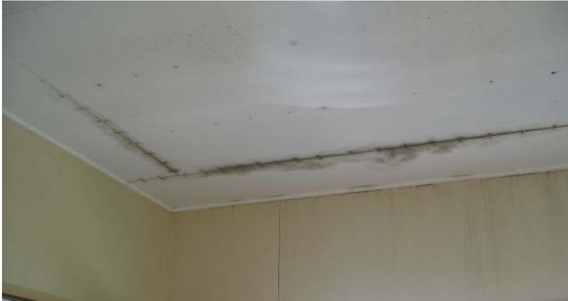
Figure 34: Water ingress at Ranger house on Smith Point
