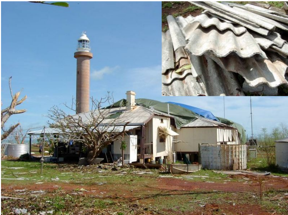
Figure 29: Rear of guest lodge with scatter of corrugated asbestos cladding
