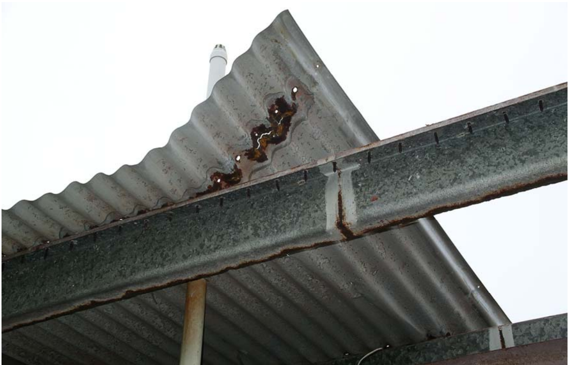
Figure 43: Corroded screws and cladding at Minjilang
