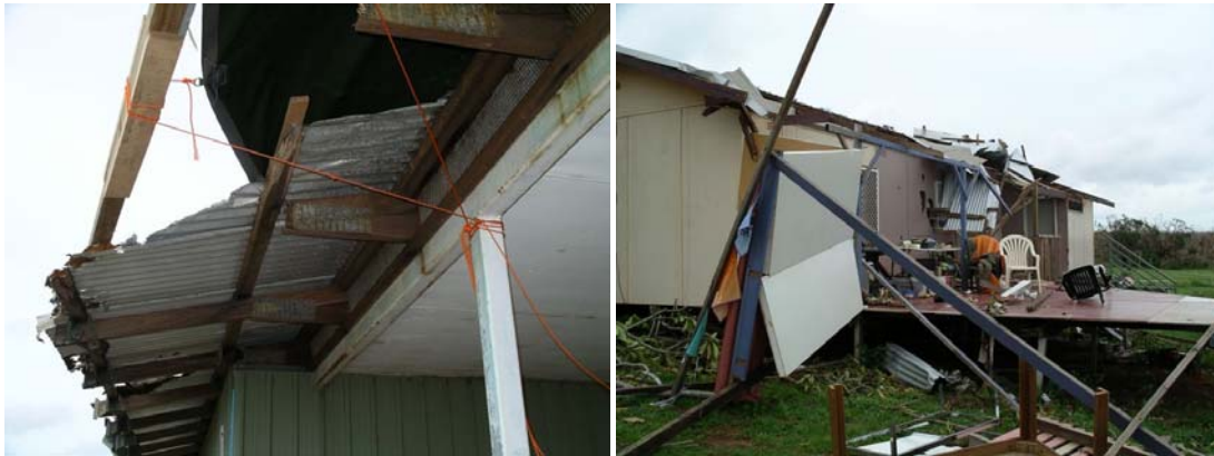
Figure 32 (a) and (b): Failure of eaves, awnings and associated damage to structures
