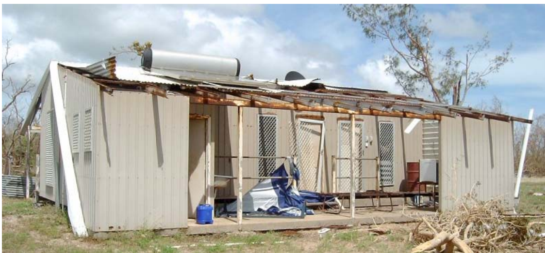
Figure 41: Corrosion of frames, battens, fixings and claddings
