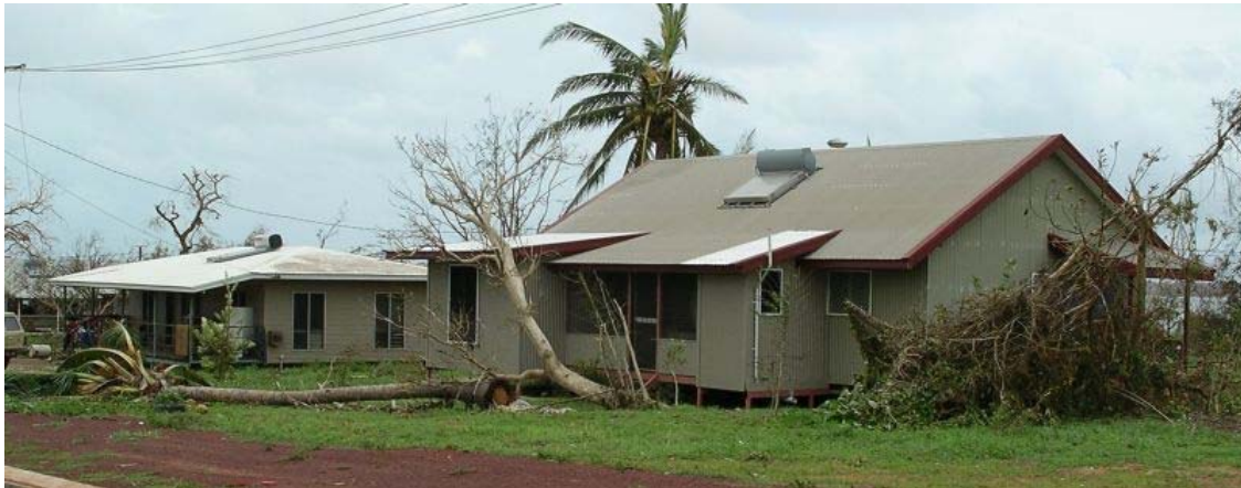
Figure 10: Minor tree damage to post Tracy houses
