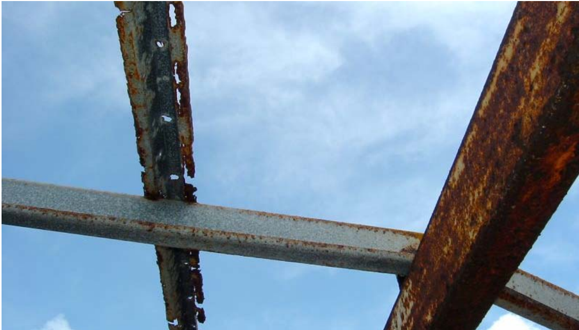
Figure 42: Detail of corrosion of top hat batten
