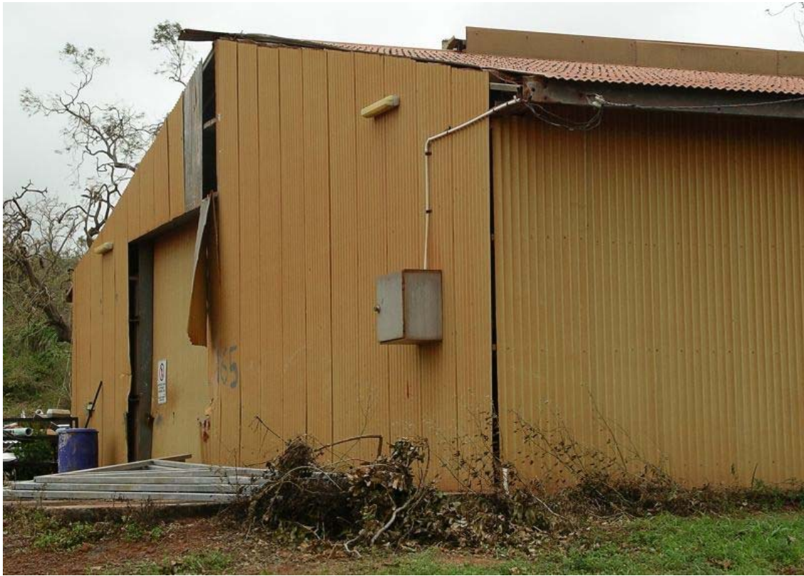
Figure 26: Leeward wall cladding and flashing failure
