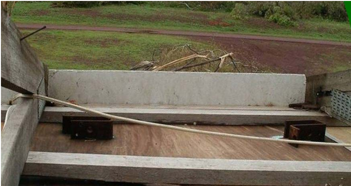
Figure 17: Truss hold down brackets not installed to a couple of trusses
