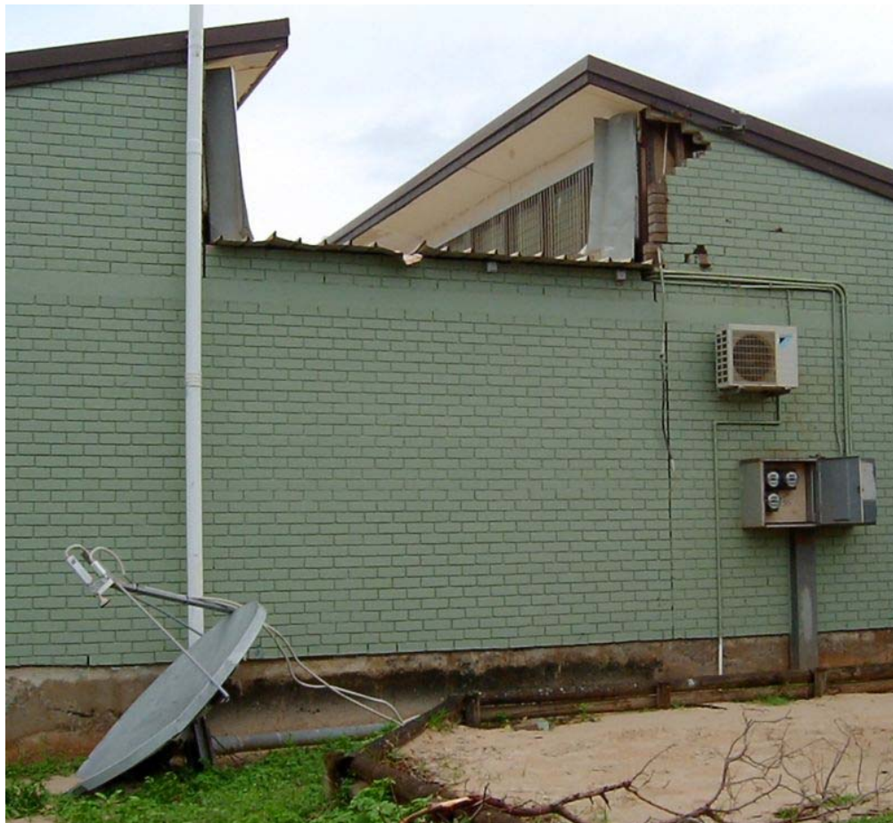
Figure 23: Failure of mounting point for satellite dish
