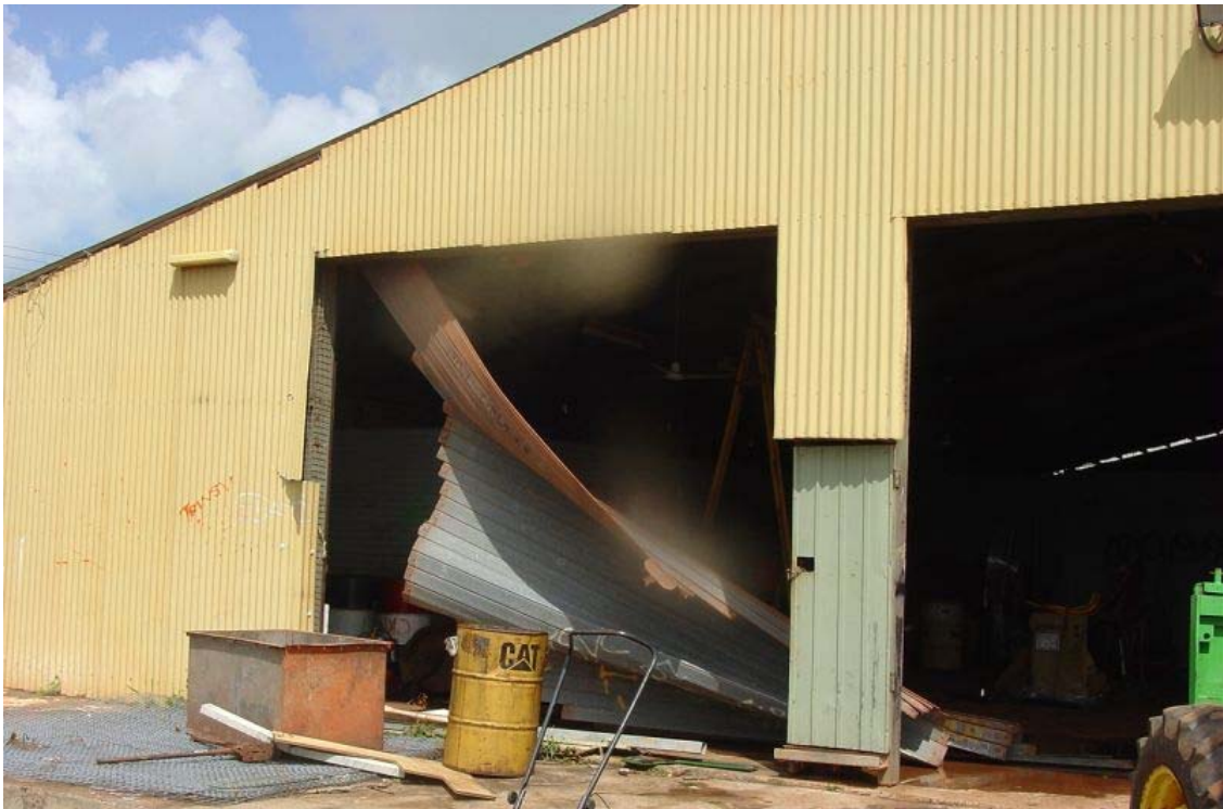
Figure 25: Roller door failure (Photo from DIPE)
