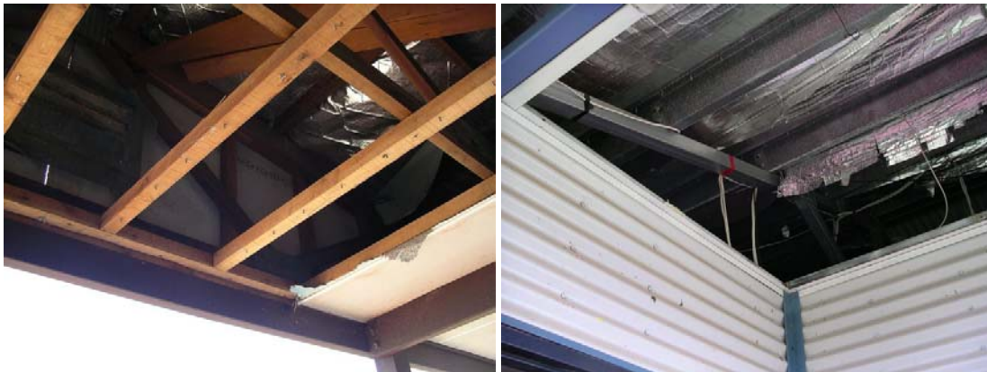
Figure 33 (a) and (b): Soffit damage at Smith Point and Minjilang
