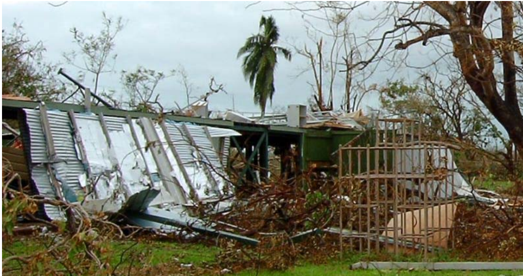
Figure 18: Elevated school platform (roofing screwed to I beams)
