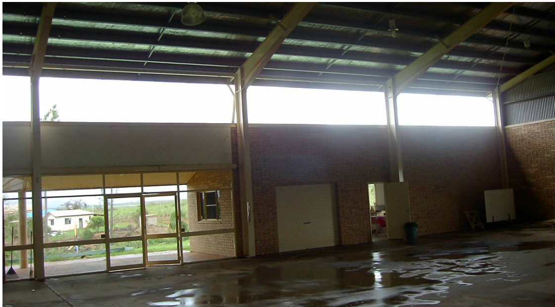
Figure 7.25: View of Failed Banks of Louvre Windows to Large Hall
