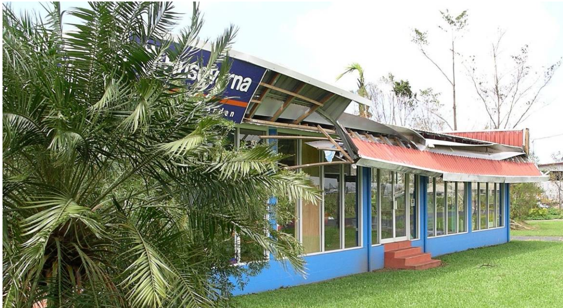
Figure 6.19: Parapet failure
