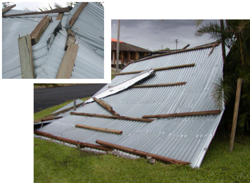
Figure 7.5: Batten to rafter connection failure
