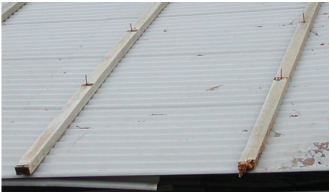
Figure 7.6: Batten to rafter failure with one nail per joint
