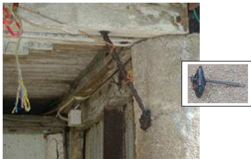
Figure 6.1: Corrosion of Connections
