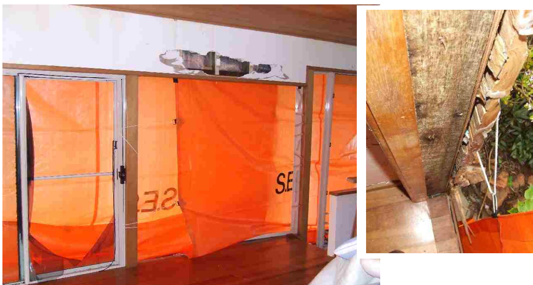
Figure 7.4: Failure of Windows & Frames in windward Wall at Main Level
