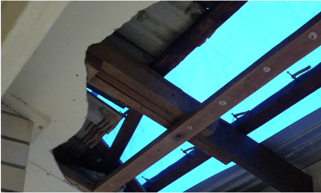
Figure 6.23: Detail of tile roof cladding failure
