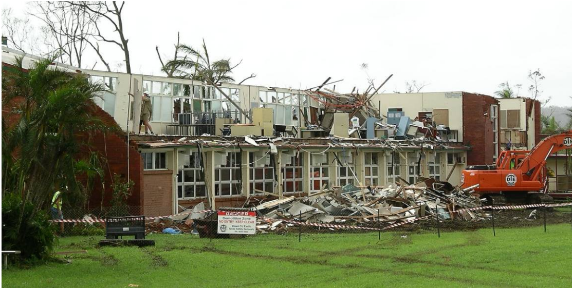
Figure 7.20: Loss of roof and wall structure
