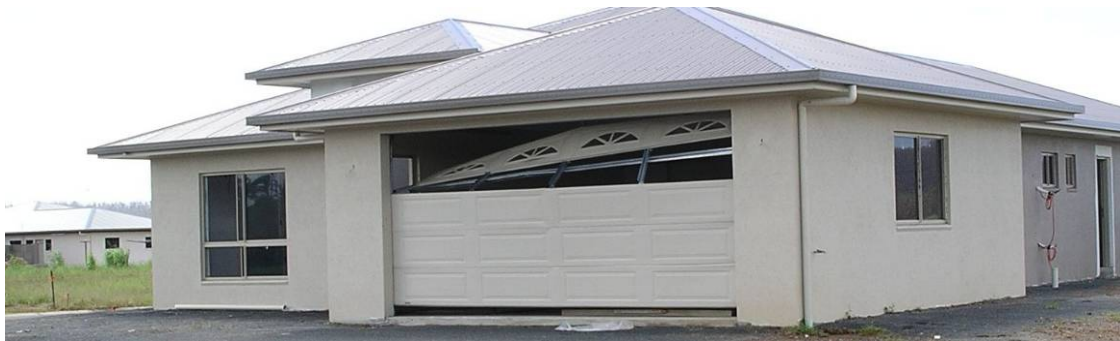
Figure 5.13: Panel garage door failure
