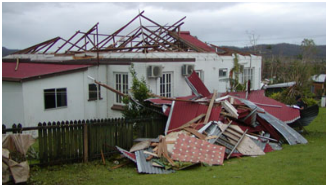
Figure 6.6: Loss of ridge beams
