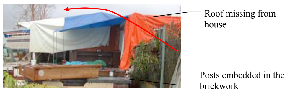
Figure 7.12: Missing barbeque area roof
