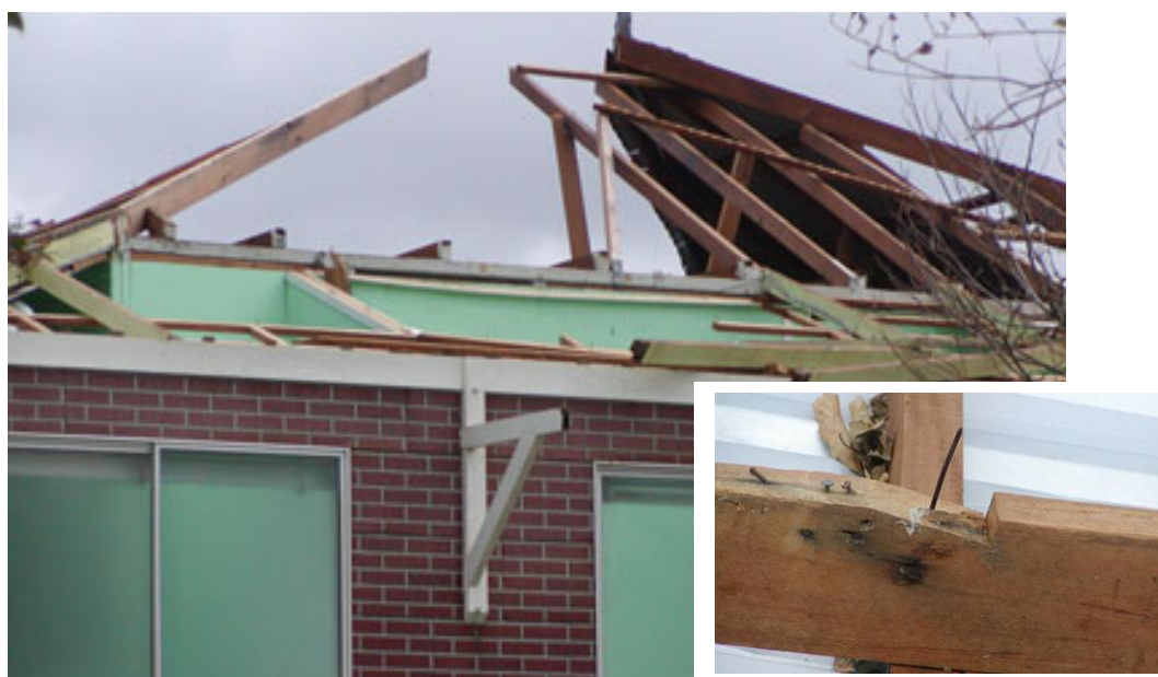
Figure 6.4: Failure of rafter to wall connection
