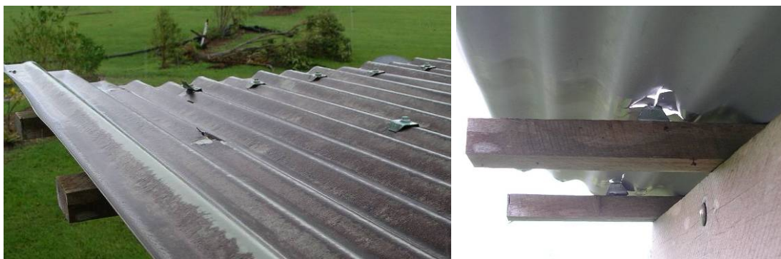
Figure 6.20: Inadequate fixing spacing and excessive side edge distance
