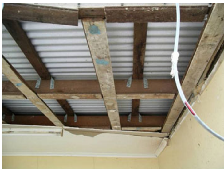
Figure 6.8: Improvements in batten-to-rafter connection
