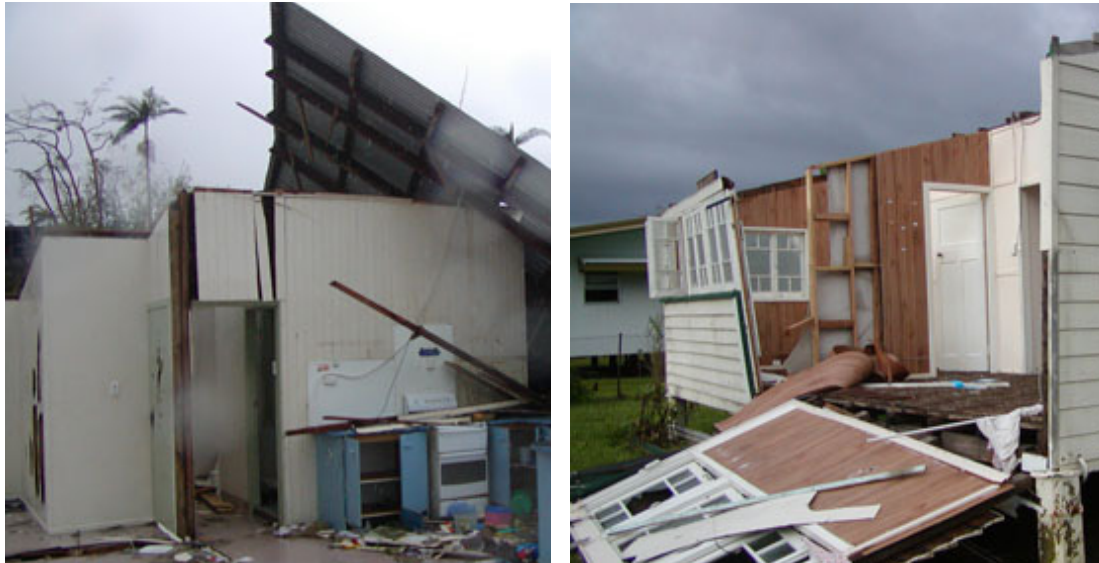
(a) Spliced rafters separated from walls
