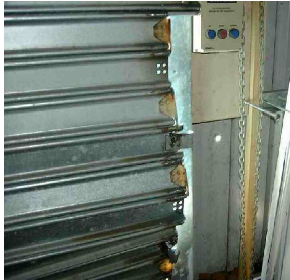
Figure 7.18: Detailed View of Failed Wind Locks to Roller Door (Wind locks fitted to every second slat)
