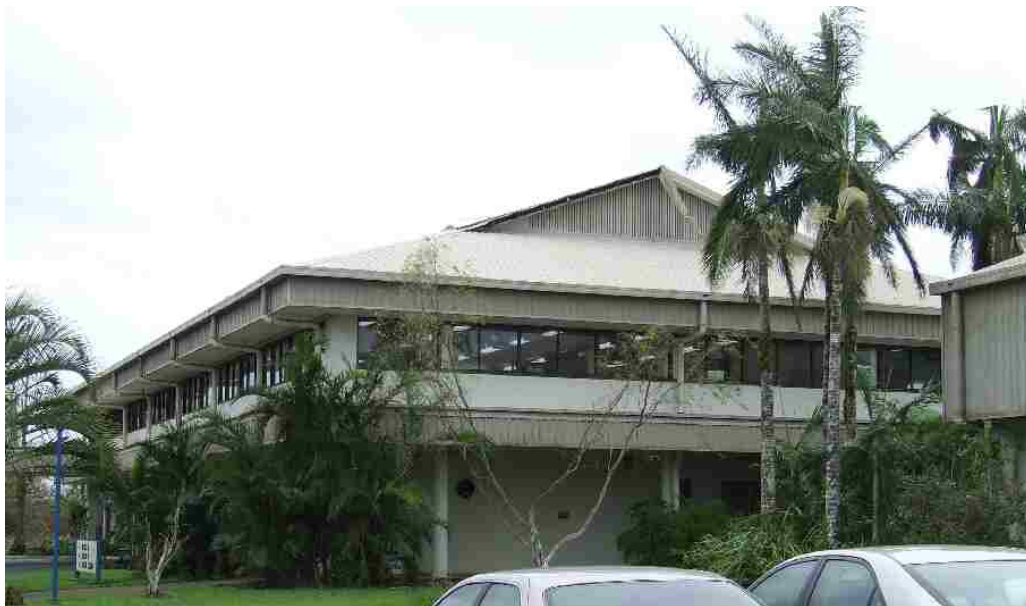
Figure 7.23: Loss of flashing at Dutch gable end
