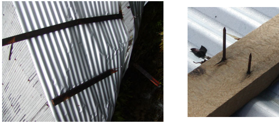
Figure 6.3: Failure of batten-to-rafter connection (Refurbished roofing on an “Old Queenslander”)
