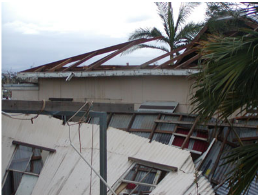
Figure 7.13: Garage damage and partial loss of house roof
