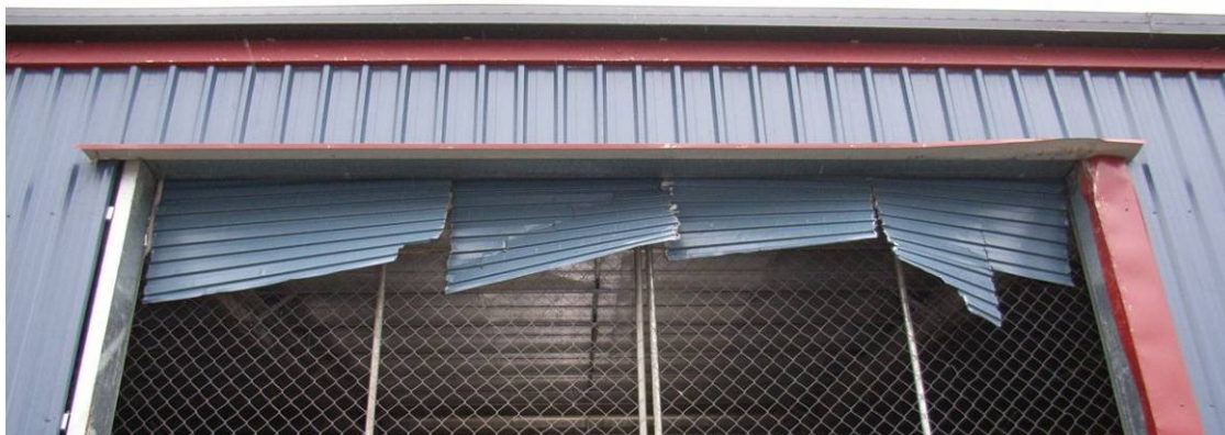
Figure 5.10: Torn sheet type roller door
