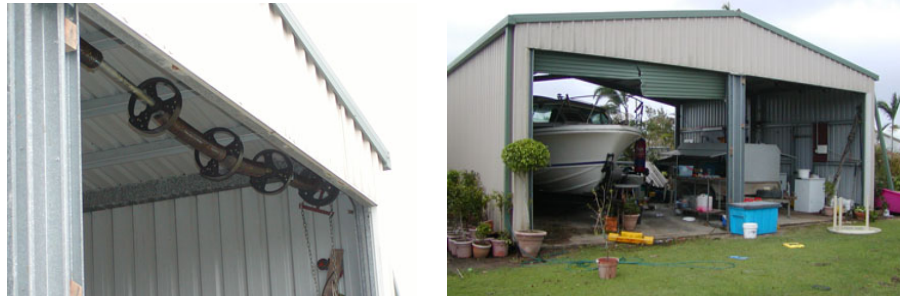
Figure 7.19: Failure of roller doors and back wall of shed
