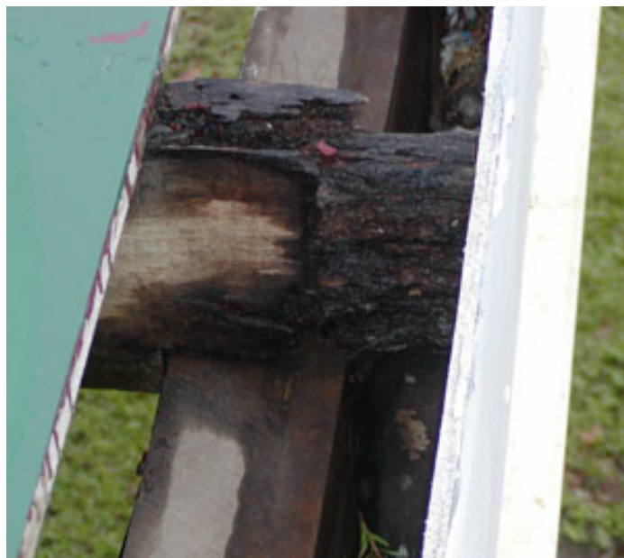
Figure 6.2: Deterioration of Timber (Floor joist at external wall connection in refurbished house)
