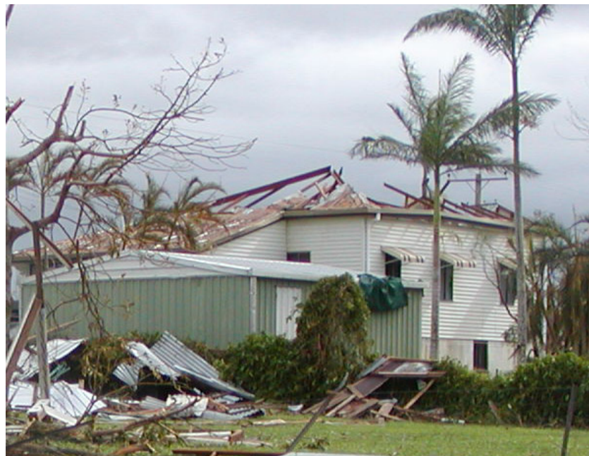
Figure 7.8: Loss of ridge and struts
