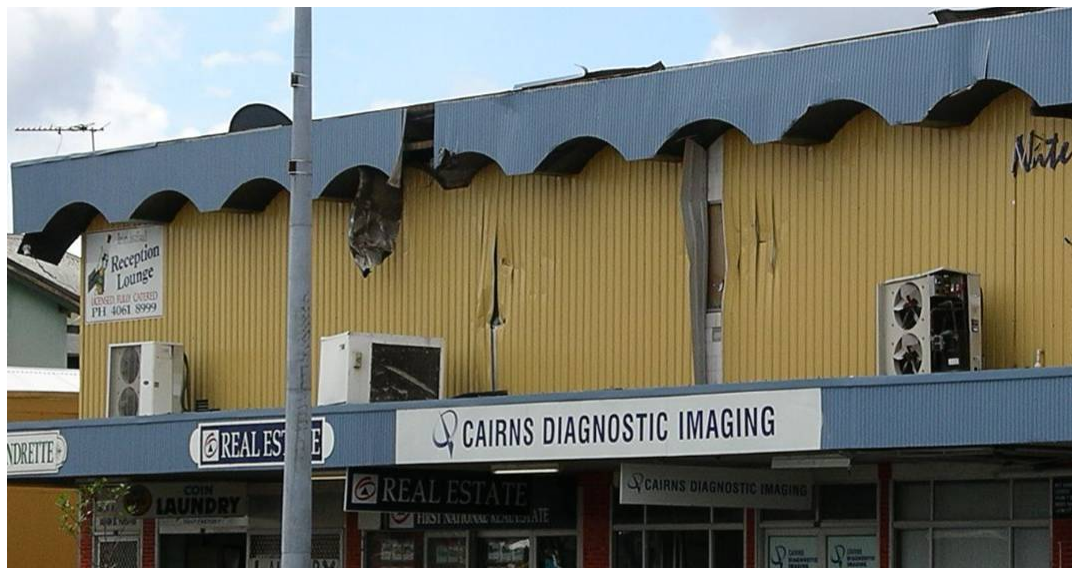
Figure 6.16: Damage to and from air conditioning units
