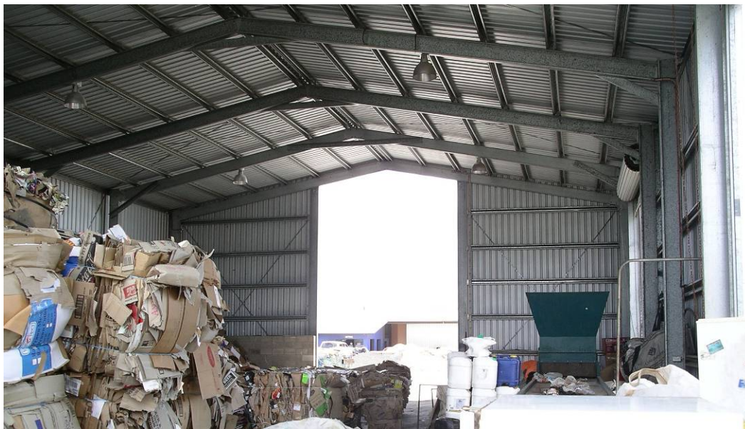
Figure 4.7: Example of a cold formed steel frame industrial shed
