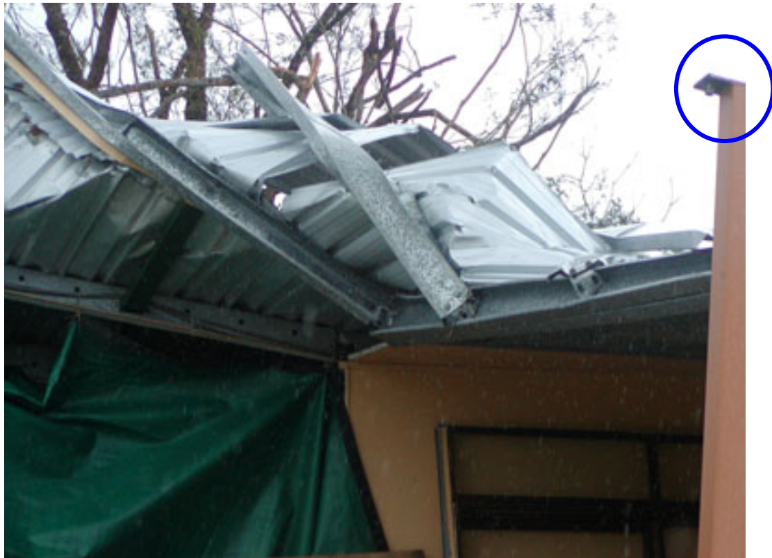
Figure 7.10: Failure of steel beam to post connection
