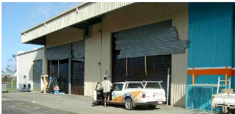
Figure 7.17: Two of the failed roller doors
