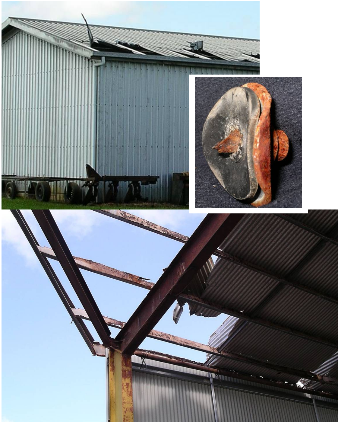
Figure 6.18: Corrosion in buildings
