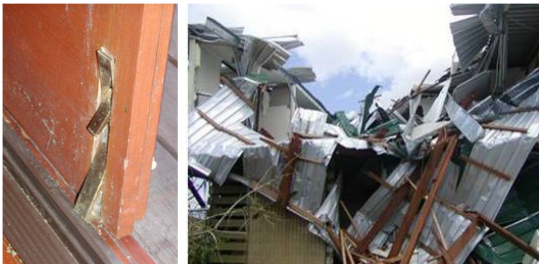
(a) window and door furniture (b) large debris damaging whole walls
