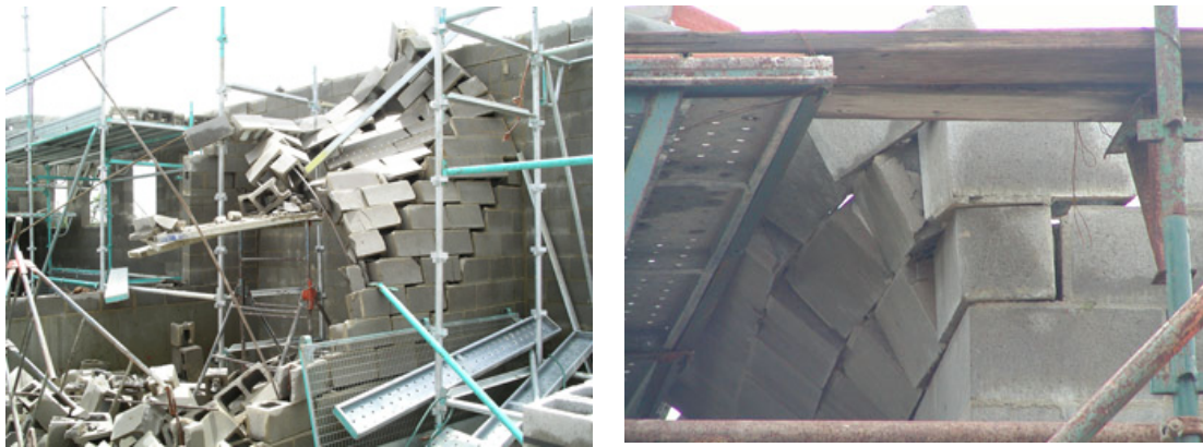
Figure 6.11: Damage to Concrete block work under construction
