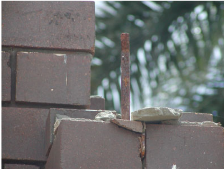
Figure 7.15: Broken tie-down bolt at garage lintel
