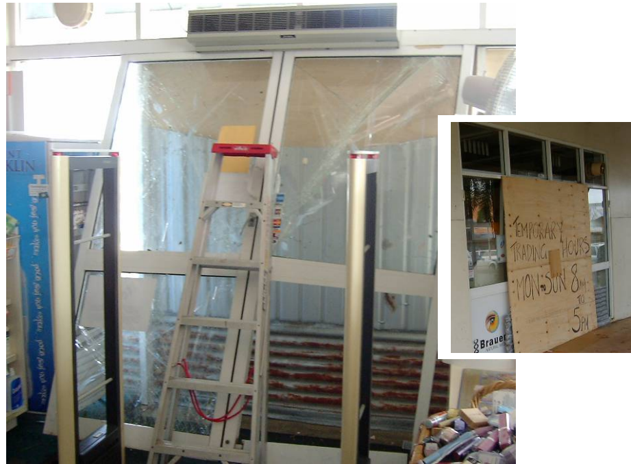
Figure 6.14: Damaged sliding shop doors
