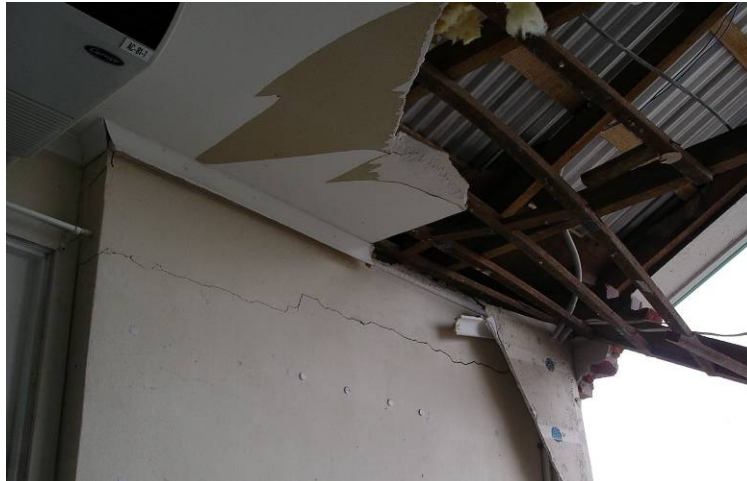
(a) Crack in pier
