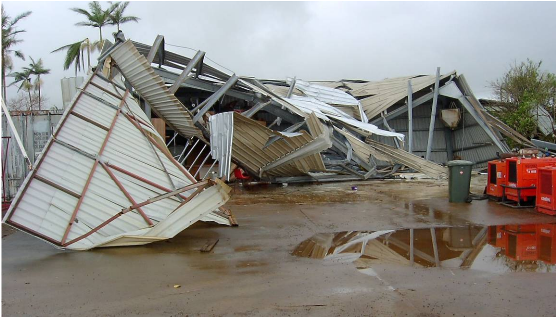
Figure 5.8: Collapse of cold formed steel industrial shed
