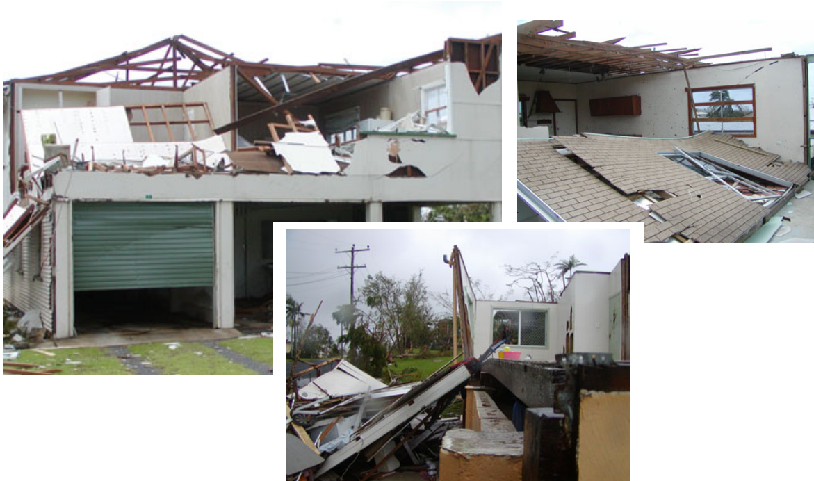
Figure 6.5: Loss of walls following roof structure damage
