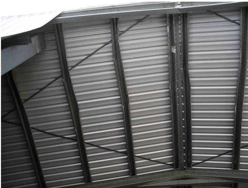
Figure 7.26: Buckled top hat roof battens in end bay
