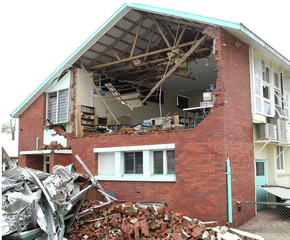
(b) End wall collapse
