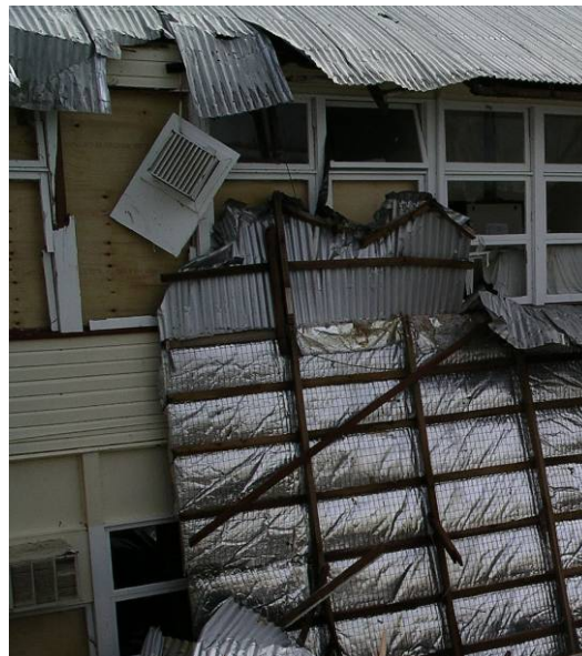
Figure 7.21: Impact damage from leaf of roof
