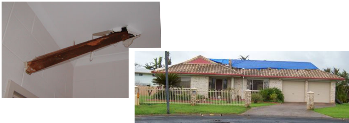
(a) debris penetration through metal roof (b) tile damage after debris impact
