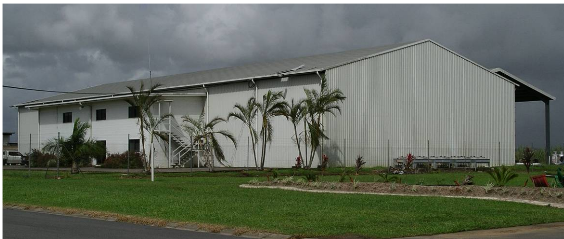
Figure 5.6: Hot rolled steel framed shed
