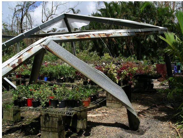
Figure 6.15 Damage to shade cloth structures
