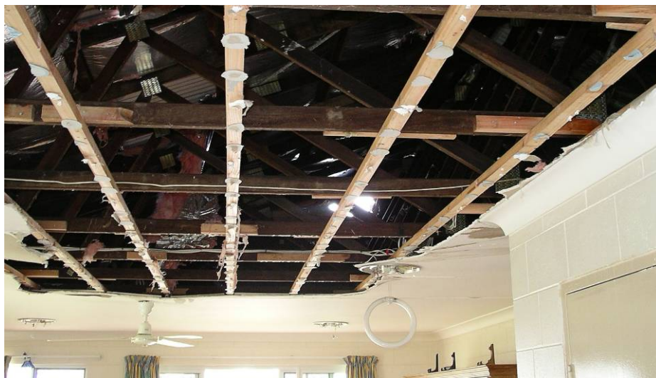
Figure 6.10: Debris damage to Dutch gable and roof cladding leading to collapse of ceiling from water ingress
