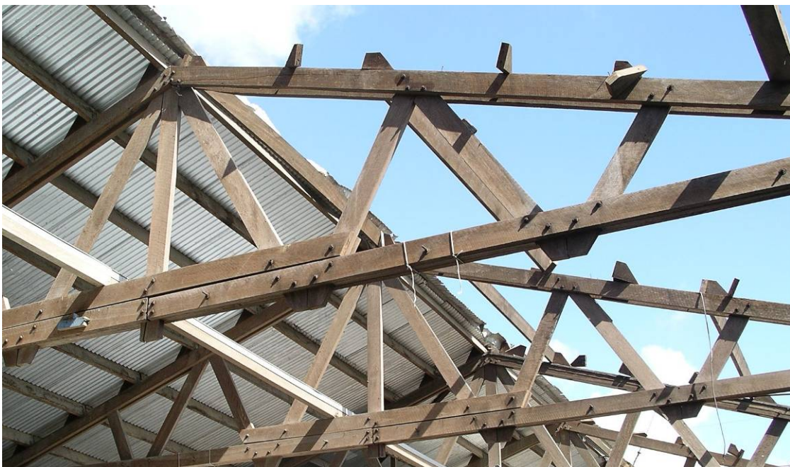
Figure 5.9: Loss of timber purlins and new cladding from old industrial shed
