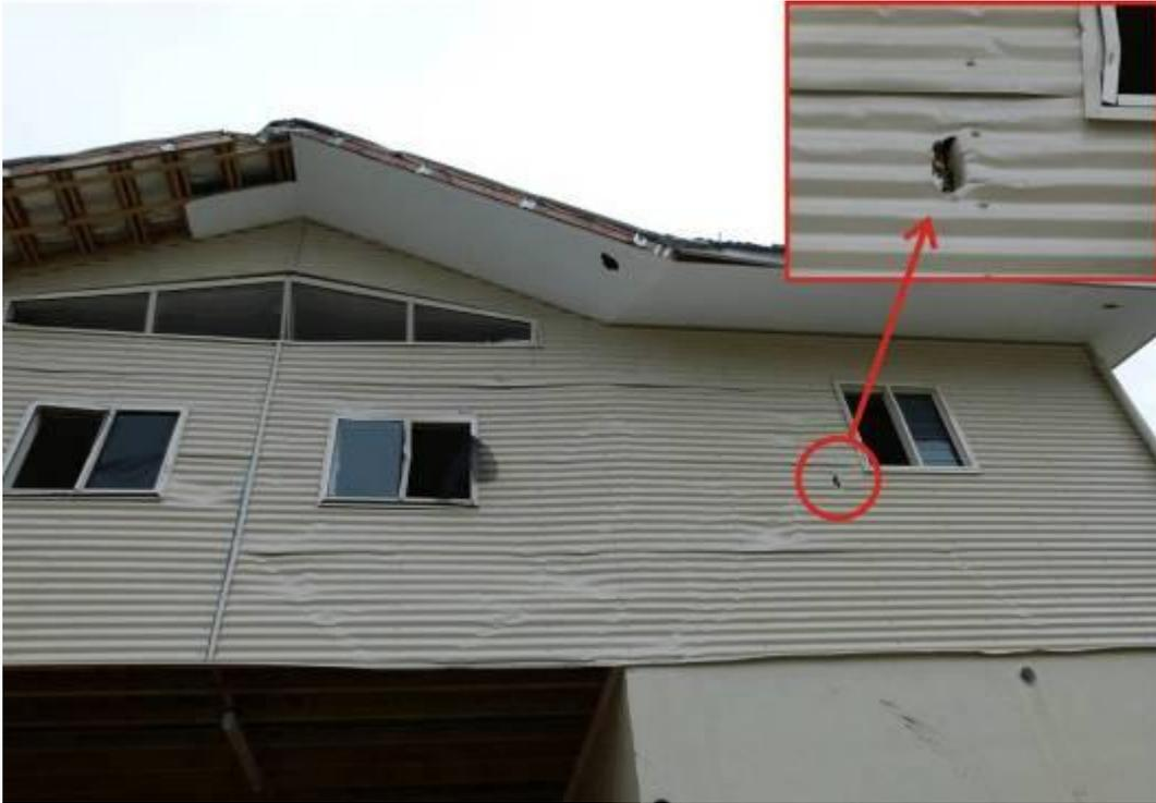
**Figure 3.58 Impact damage on metal cladding without complete missile penetration**
