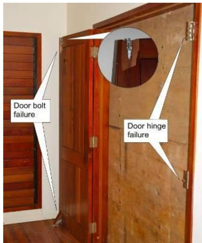
**Figure 3.20 Door bolt and hinge failure**
