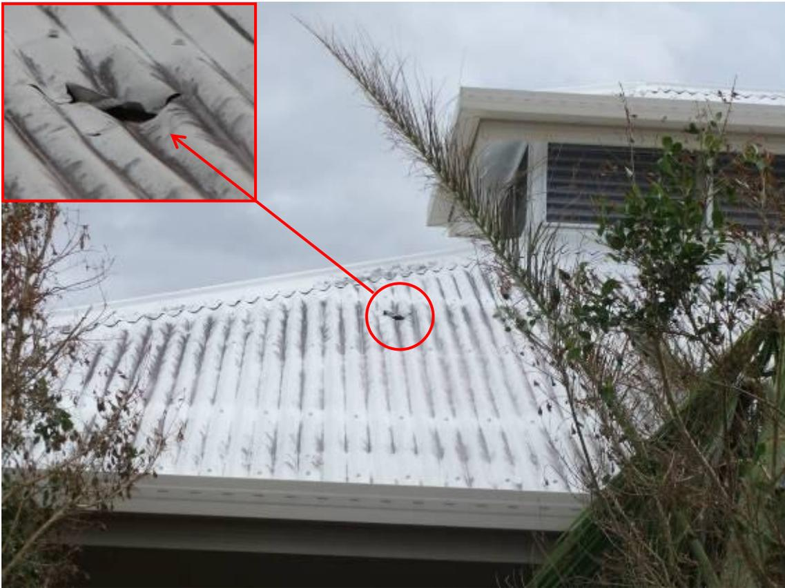
**Figure 3.57 Metal roof damaged by dislodged roof tile**
