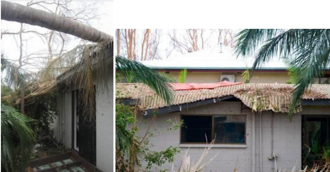
Figure 3.52(a) Tree damage to housing
