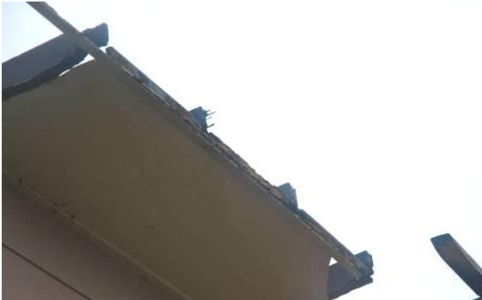
**Figure 3.46 Deterioration of timber at the very edge of a roof**
