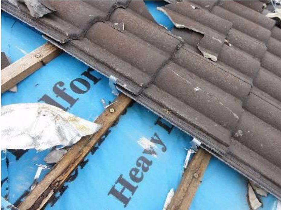
**Figure 3.32 Failed tile roof with clips from initial installation and an upgrade**
