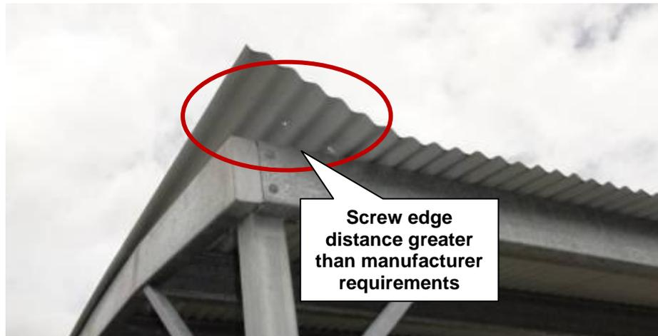
**Figure 3.36 Large edge distance led to fatigue failures in sheeting**
