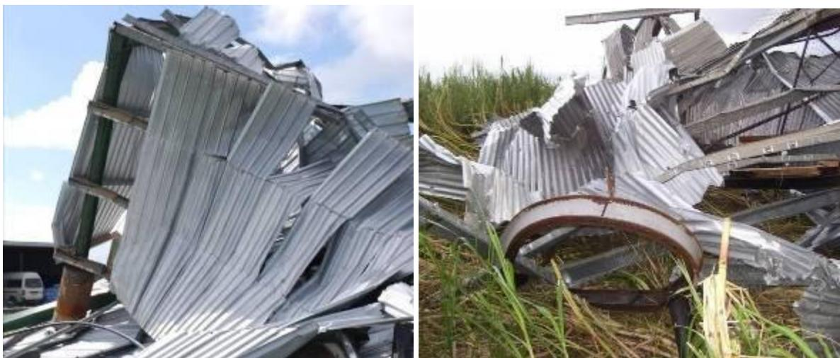
**Figure 3.41** Farm sheds with footings removed intact
