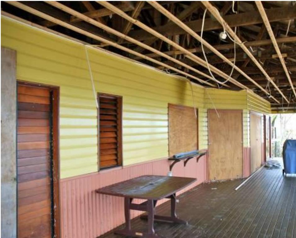
**Figure 3.65 Soffit failure under large outdoor entertainment area**
