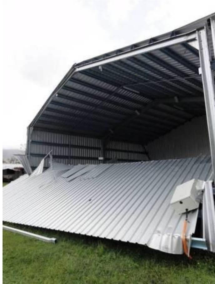
**Figure 3.40** loss of end wall under lateral loads
