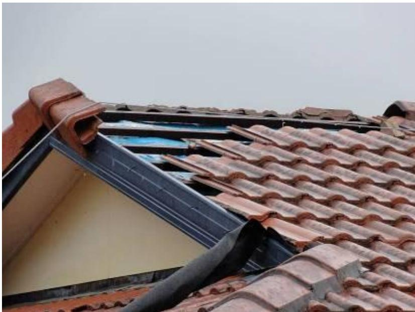
**Figure 3.33 Failure of ridge capping**
