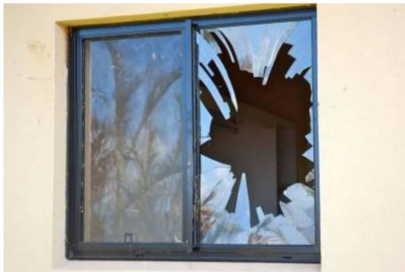
**Figure 3.15 Broken window due to concrete roof tile impact**
