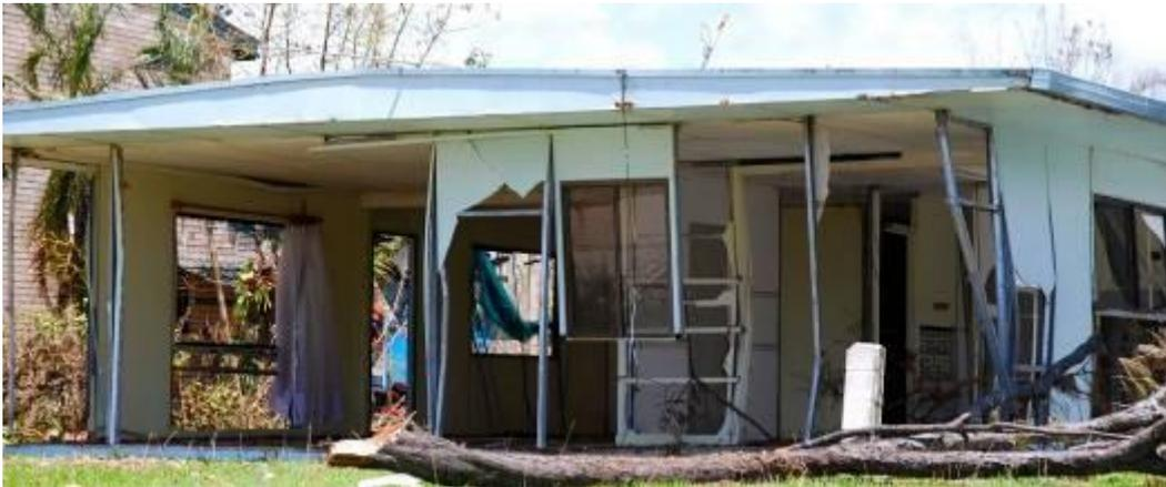
**Figure 4.12** Damage to external walls on the seaward side of a house
