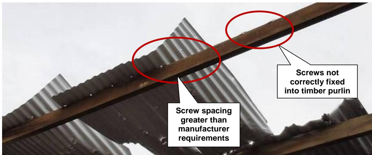
**Figure 3.35 Large fastener spacings led to fatigue failures of sheeting**
