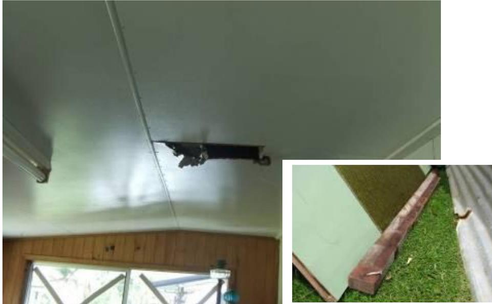
**Figure 3.60 Debris complete penetration through steel roof (inset shows missile)**
