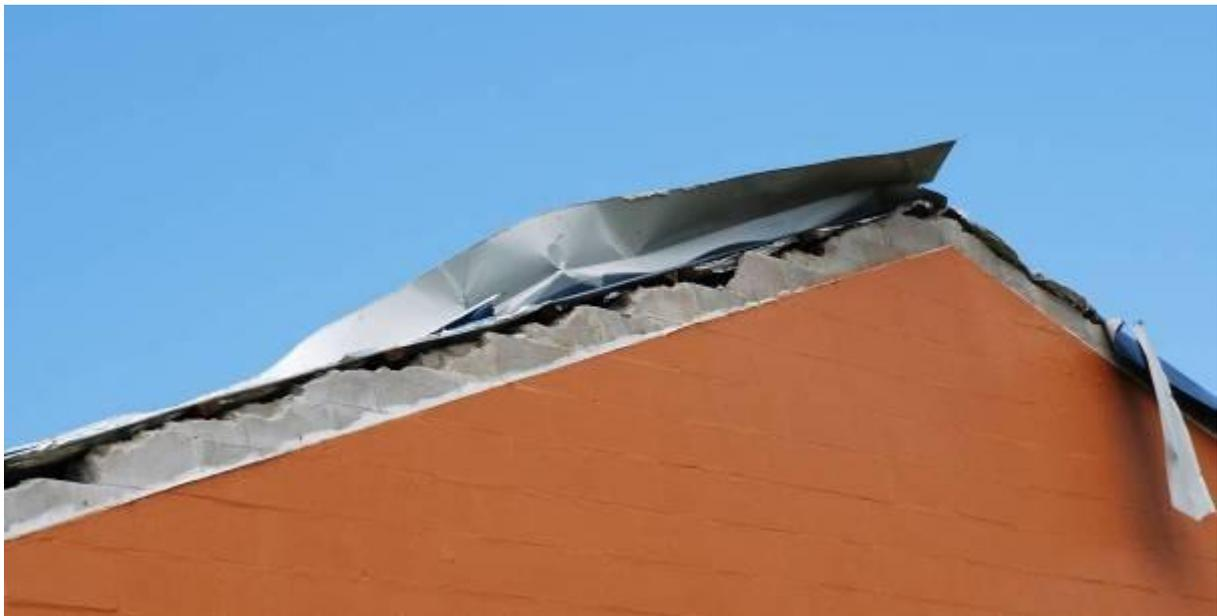
**Figure 3.68 Flashing loss**
