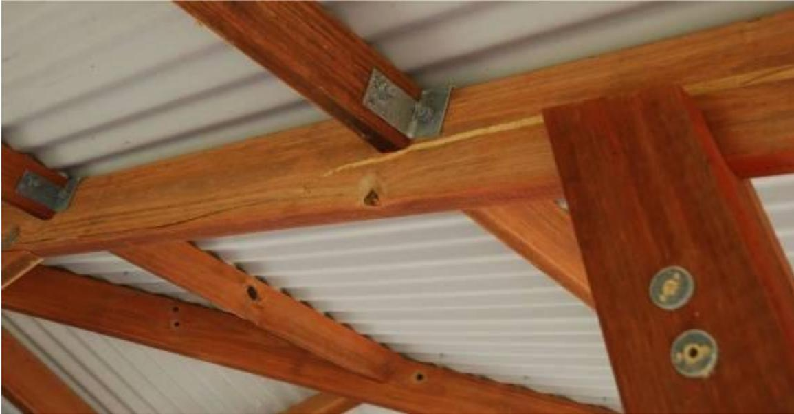
**Figure 3.47 Tension perpendicular to grain failure in rafter**
