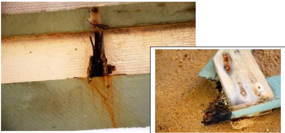
**Figure 3.45 Corrosion of nail plates and anchorages on a truss adjacent to the beach**
