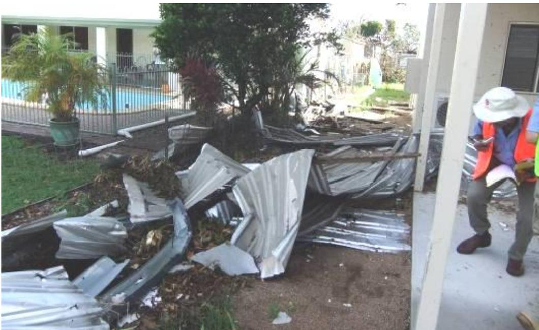
**Figure 3.11 Roofing with battens attached from house shown in Figure 3.10**
