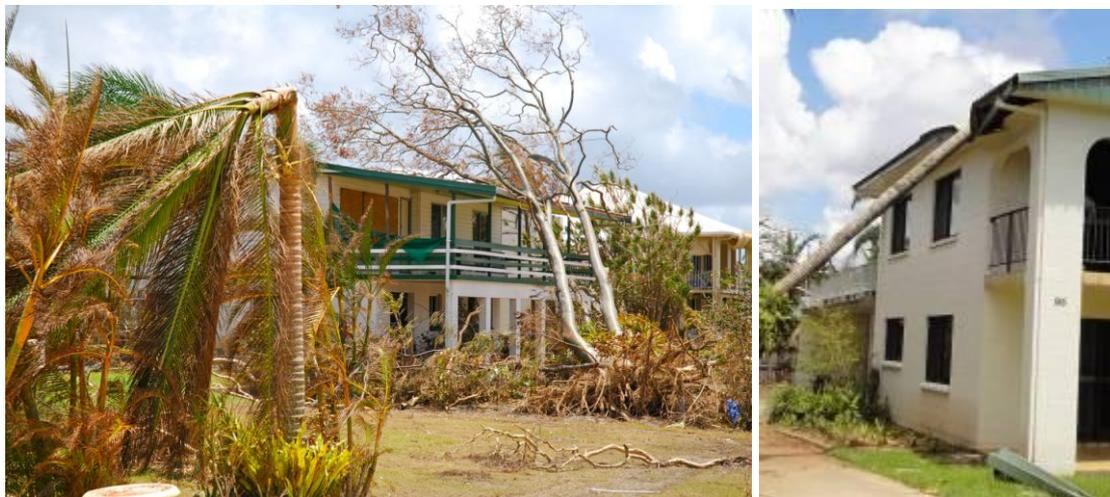
Figure 3.52(b) Tree damage to housing
