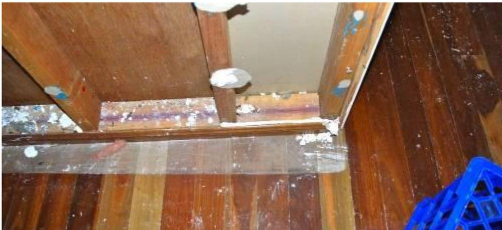
**Figure 3.49 Internal wall moved by differential air pressure**
