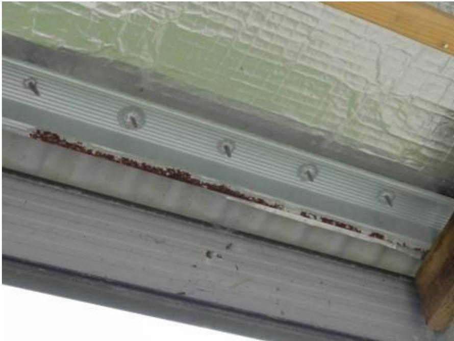
**Figure 3.44 Corrosion of eaves top hat section in beach-front house**
