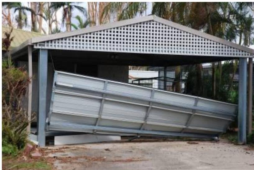
**Figure 3.30 Sectional door failure after debris impact.**
