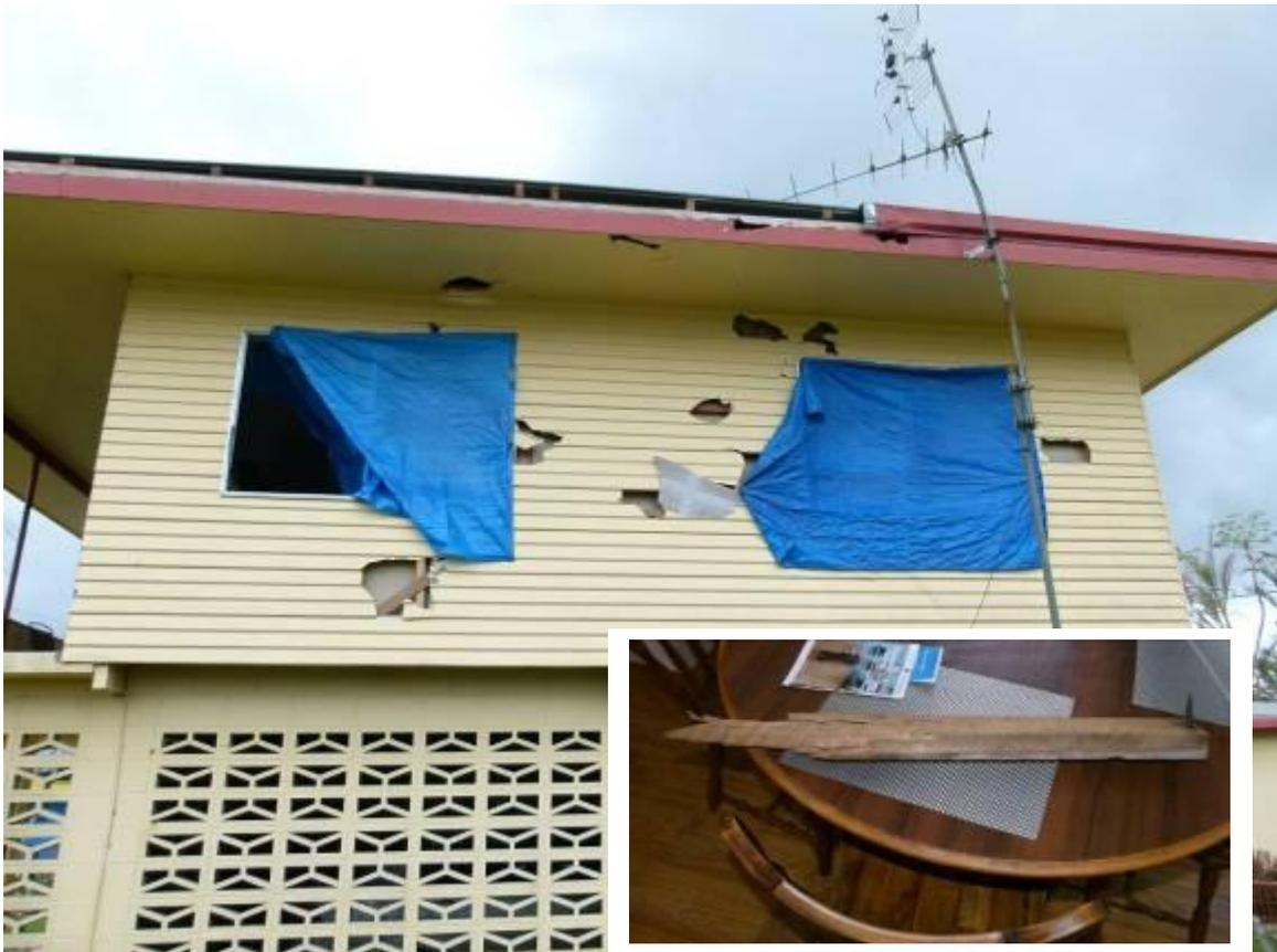
**Figure 3.61 Complete penetration through window (Inset shows missile)**
