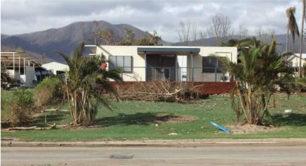
**Figure 3.10 Roof loss after door failure**
