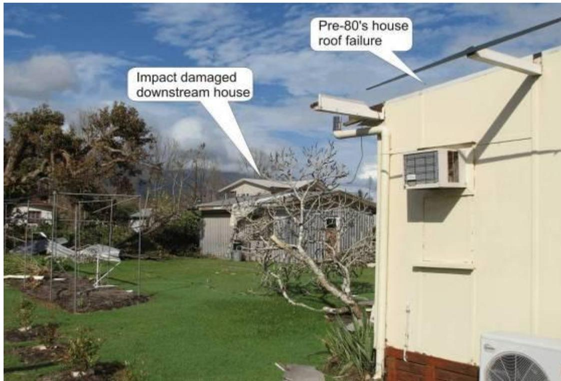
**Figure 3.55 Roof as wind-borne debris**
