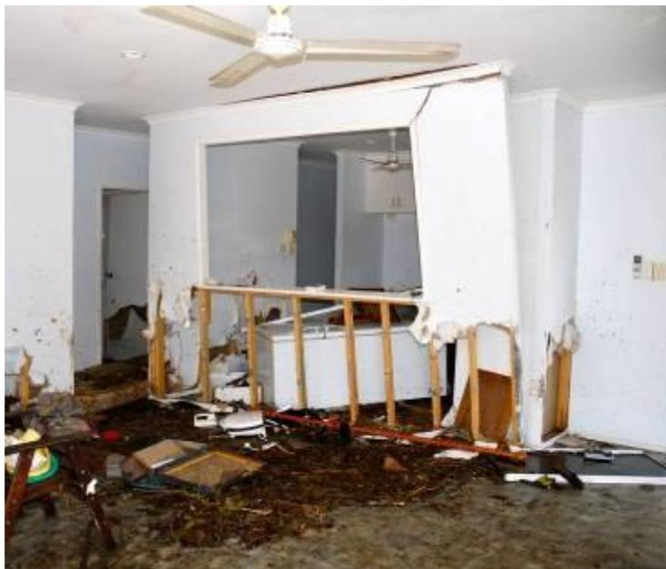
**Figure 4.10 Damage to internal linings and movement of internal walls**
