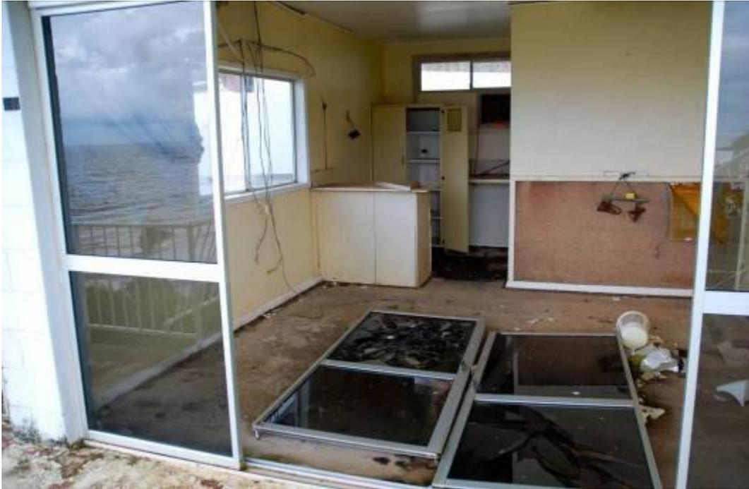
**Figure 3.16 Sliding door and window glass failures**
