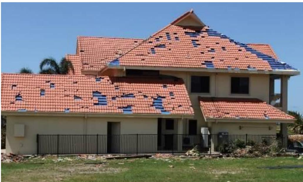
**Figure 3.56 Damaged tiled roof, each lost tile being a potential missile**
