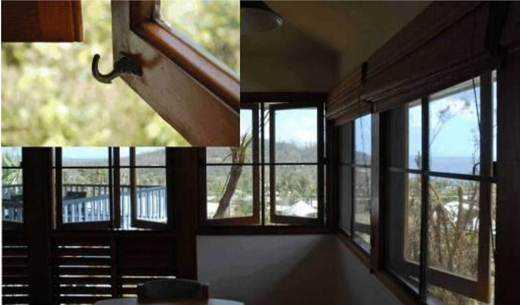
**Figure 3.23 Window latch disengagement**
