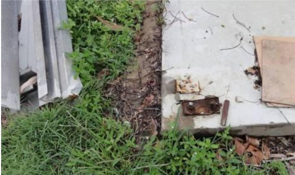
**Figure 3.42 corrosion of base plate previously welded to cold formed column**
