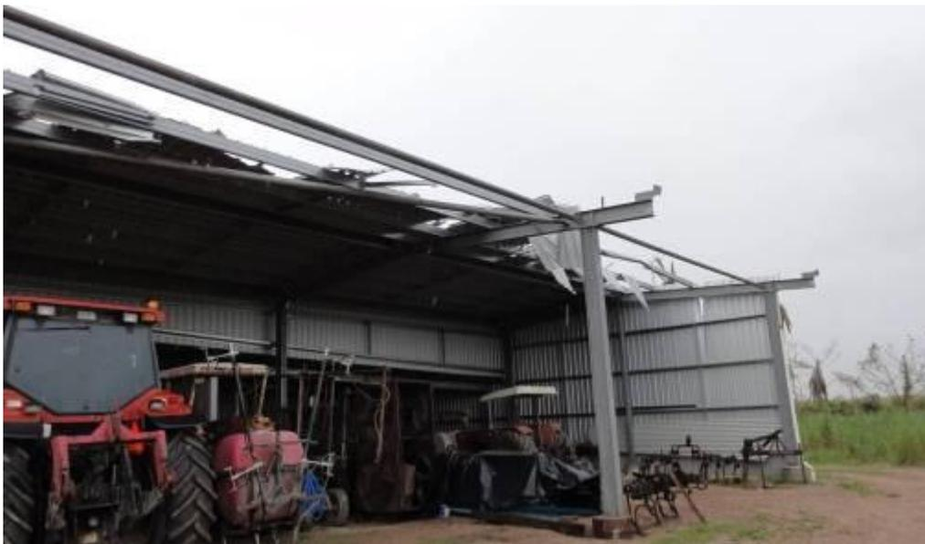
**Figure 3.39 Buckling of purlins and loss of cladding.**
