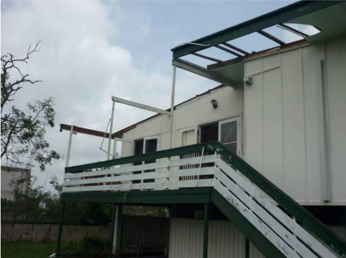
**Figure 3.9 Batten to rafter failure at 55% design wind speed**
