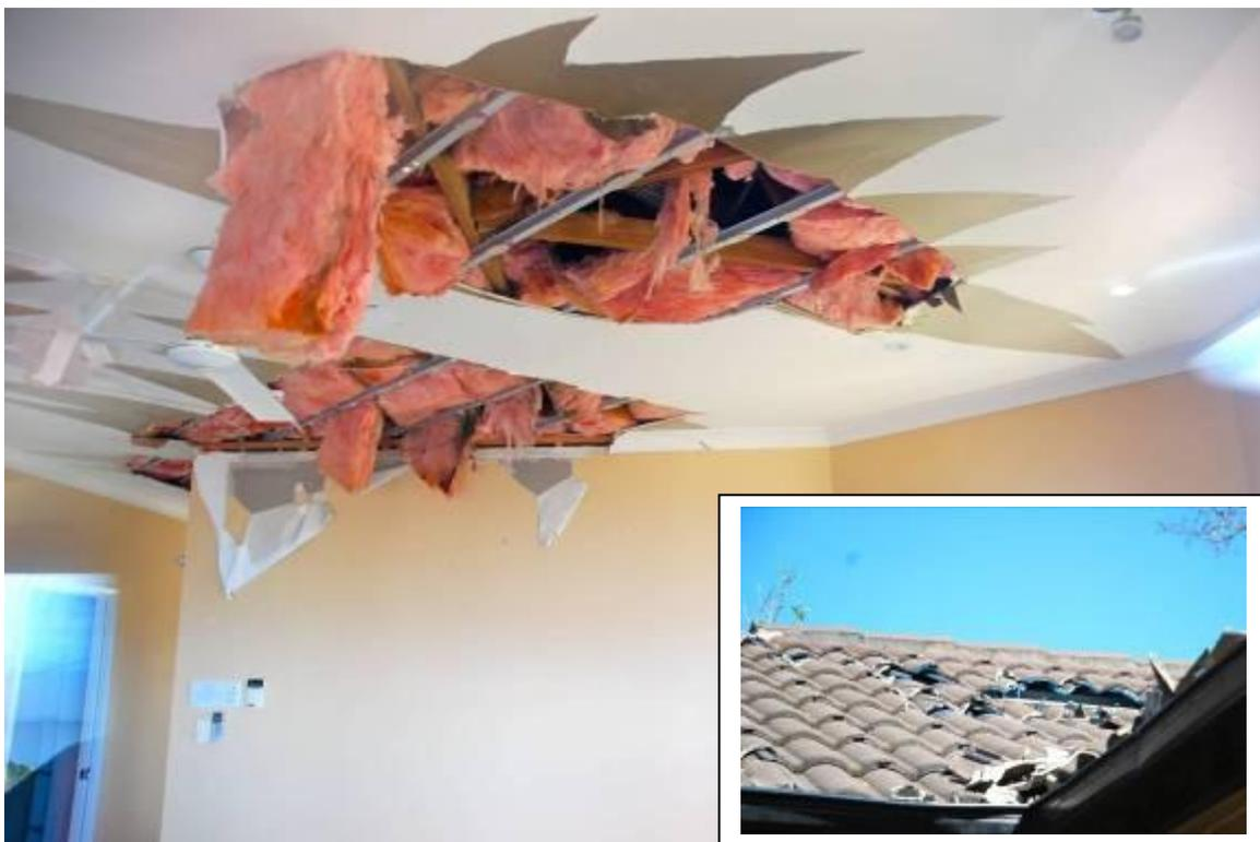
**Figure 3.34 Ceiling damage under tile damage**
