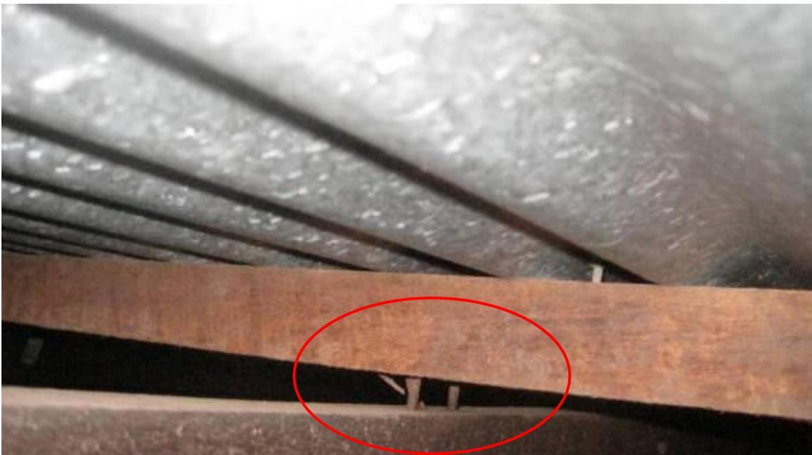
**Figure 3.43 Partial withdrawal of nails in batten to rafter connection**
