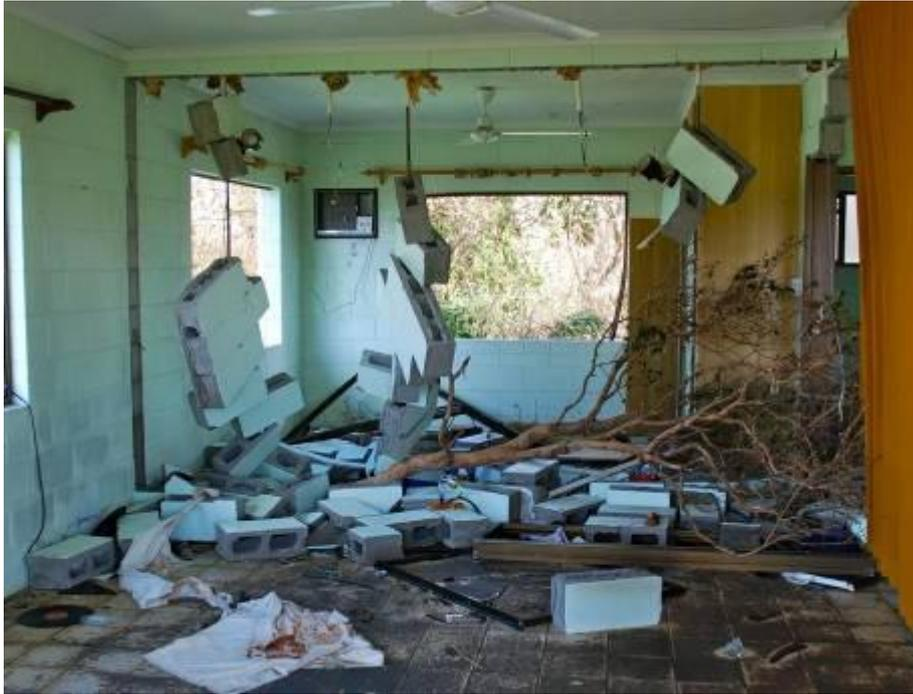
**Figure 3.50 Internal unreinforced blockwork under storm surge loading**
