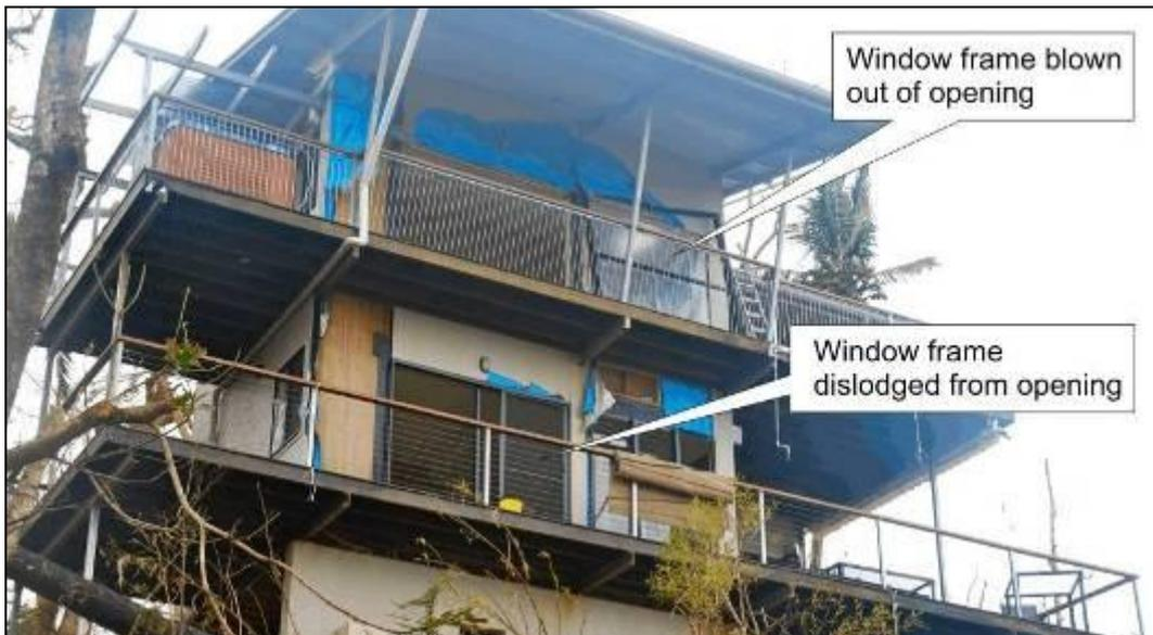
**Figure 3.17 Loss of window frames under differential pressure**
