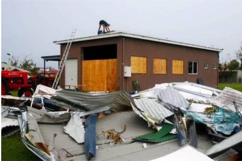
**Figure 3.67 Guttering loss**
