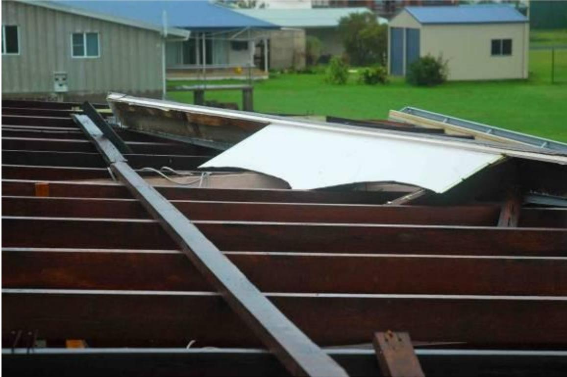
**Figure 3.7 Roof and batten loss for a second time**
