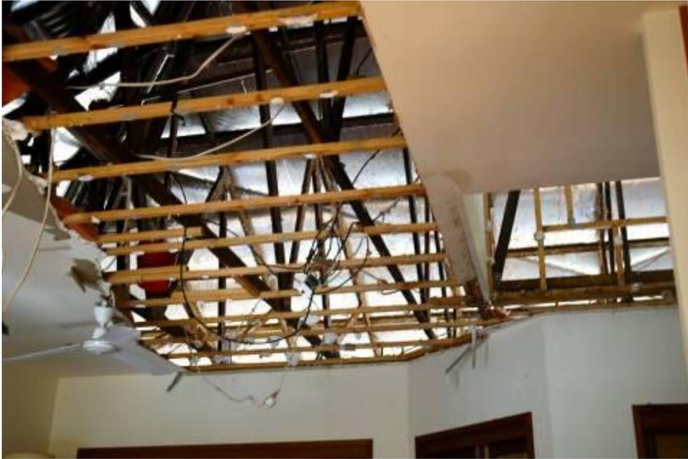
**Figure 3.64 Loss of ceiling under damaged roof**
