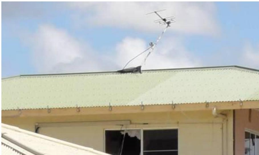
(b) damaged aerial and consequential roofing damage
