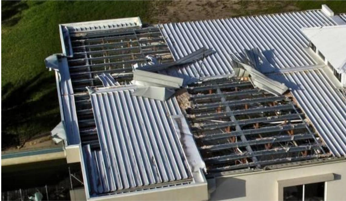
**Figure 3.37 Failure of secret fixed roofing.**
