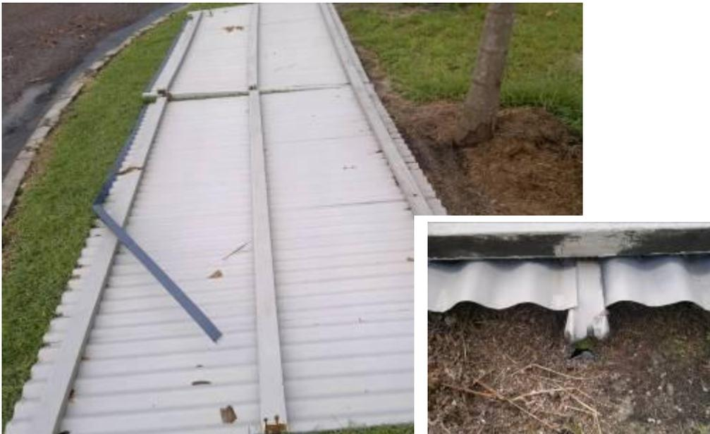
**Figure 3.76 Failed fence**
