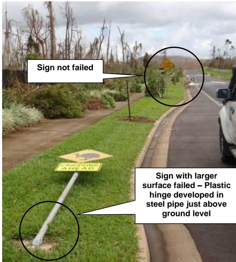
**Figure 2.1 Failed road sign with increased signage area compared to upright sign in background**
