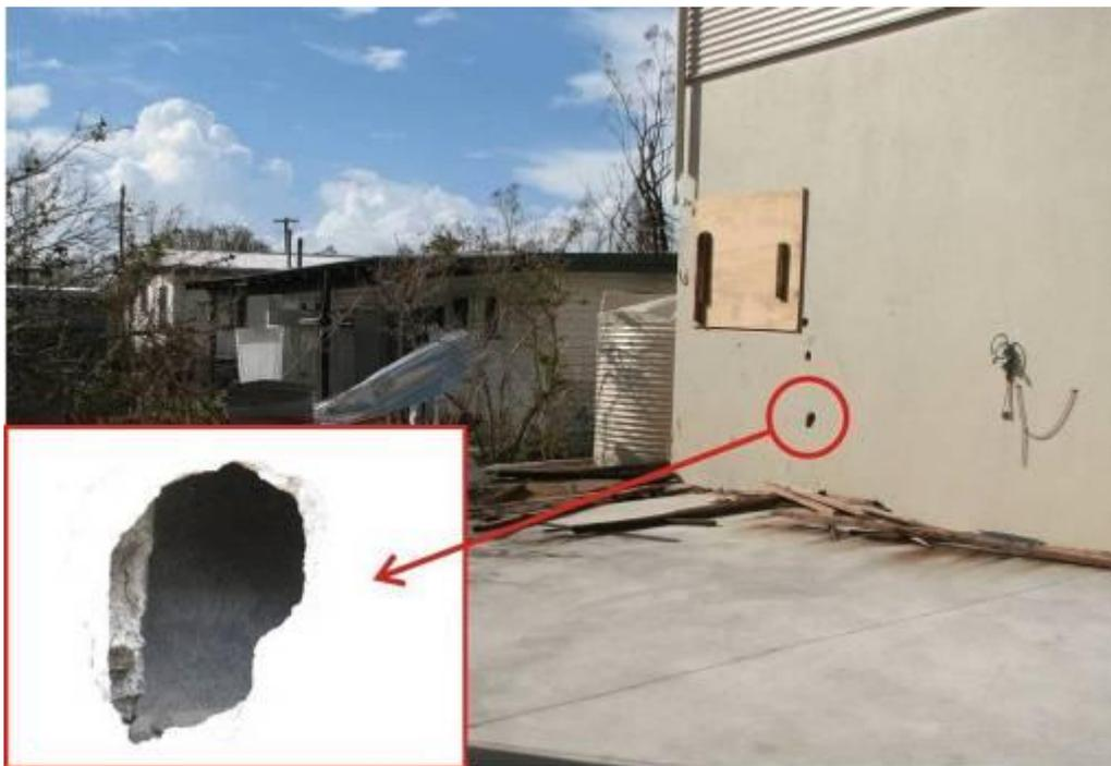
**Figure 3.59: Impact damage on concrete block wall without complete missile penetration**
