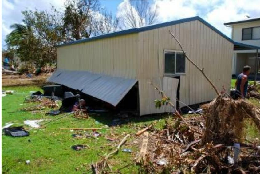
**Figure 4.11** Damage to external wall due to water flow through shed
