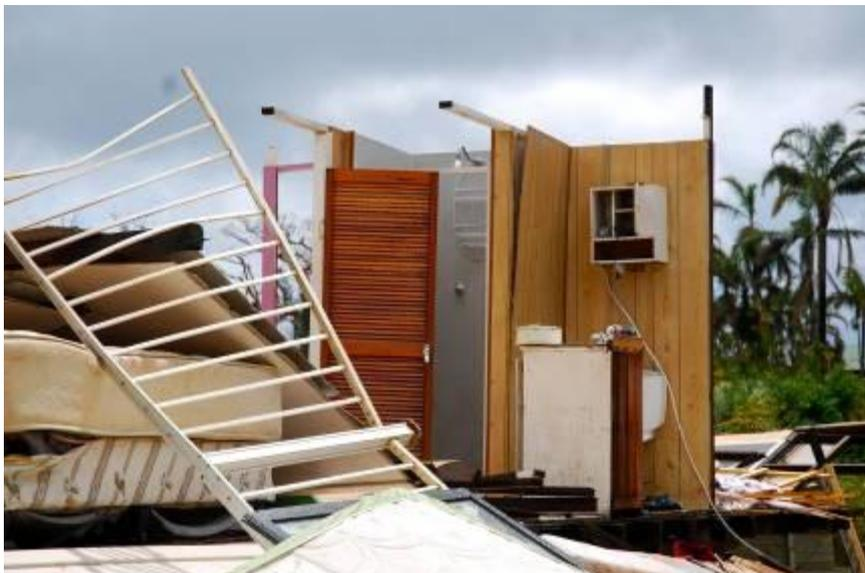
**Figure 3.51 Small rooms remaining after extreme wind damage**
