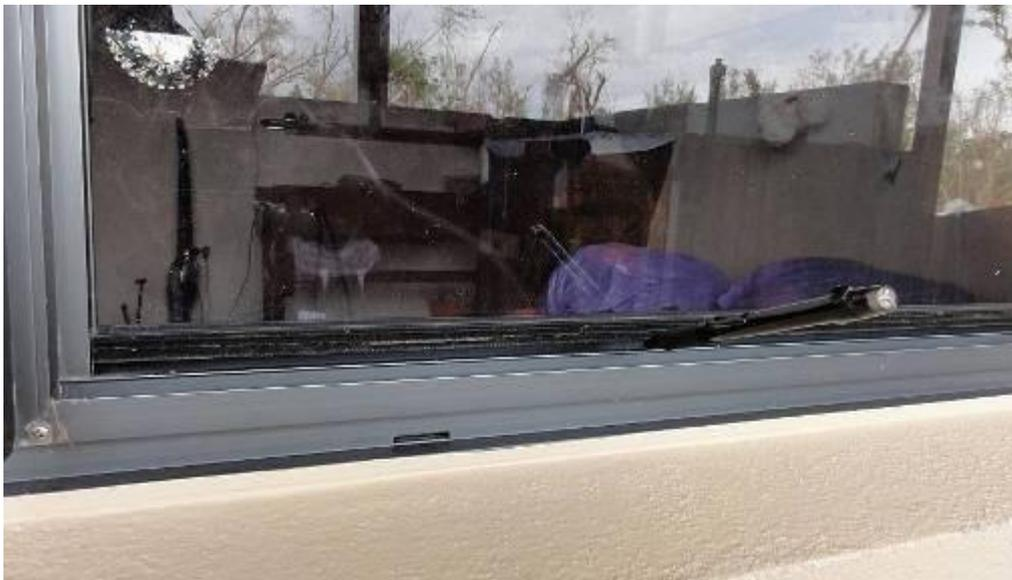
**Figure 3.22 Jamming of window in the frame**
