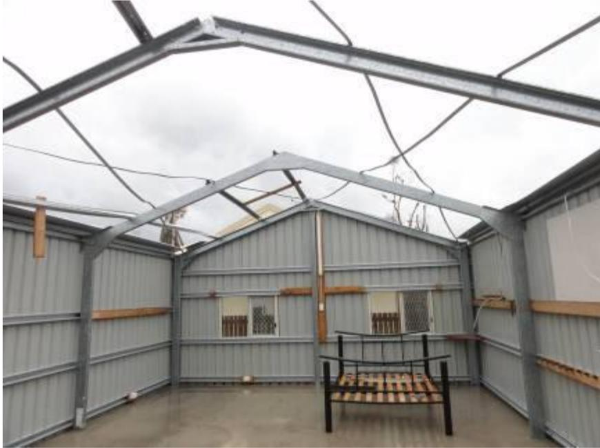
**Figure 3.38 Loss of roofing envelope after purlins buckled**
