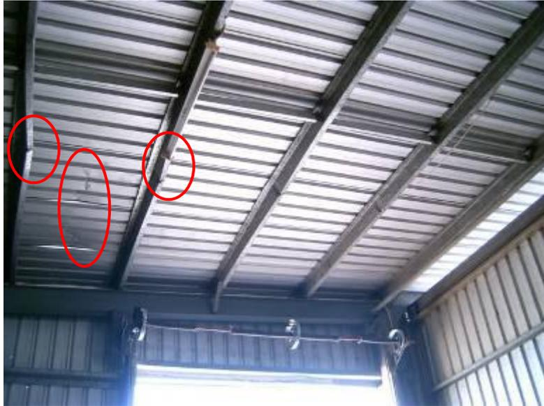
**Figure 3.27 Roller door detachment from drum**
