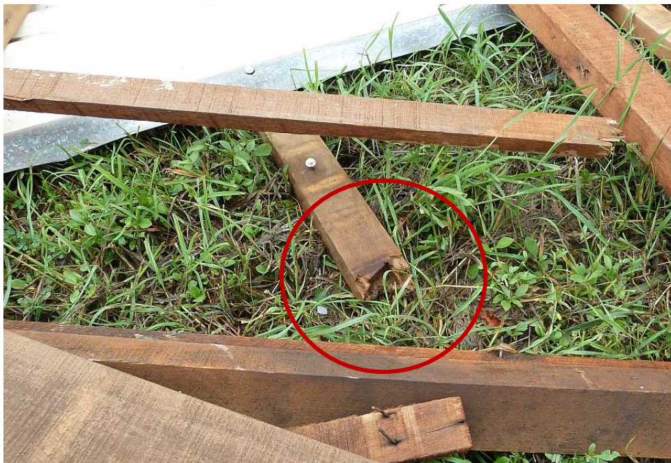
Figure 3.2 Checked recess in overbatten for rafter tie down
