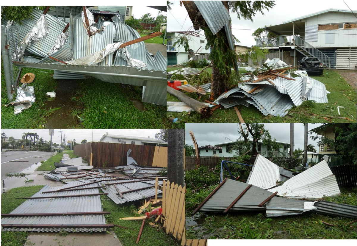
Figure 3.1 Roof cladding attached to battens (battens were only nailed to rafters)
