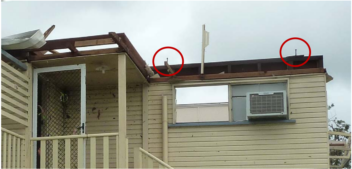
Figure 3.3 Tie down rods that were connected to the overbatten
