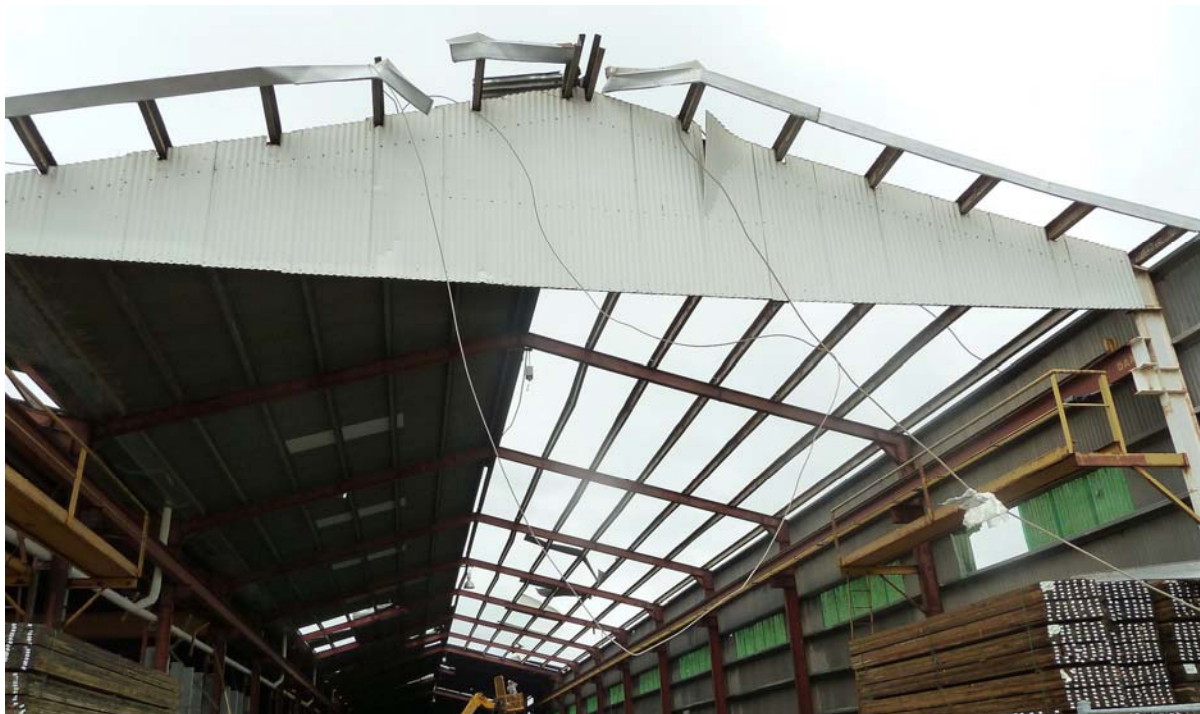
Figure 3.5: Loss of cladding and buckled purlins
