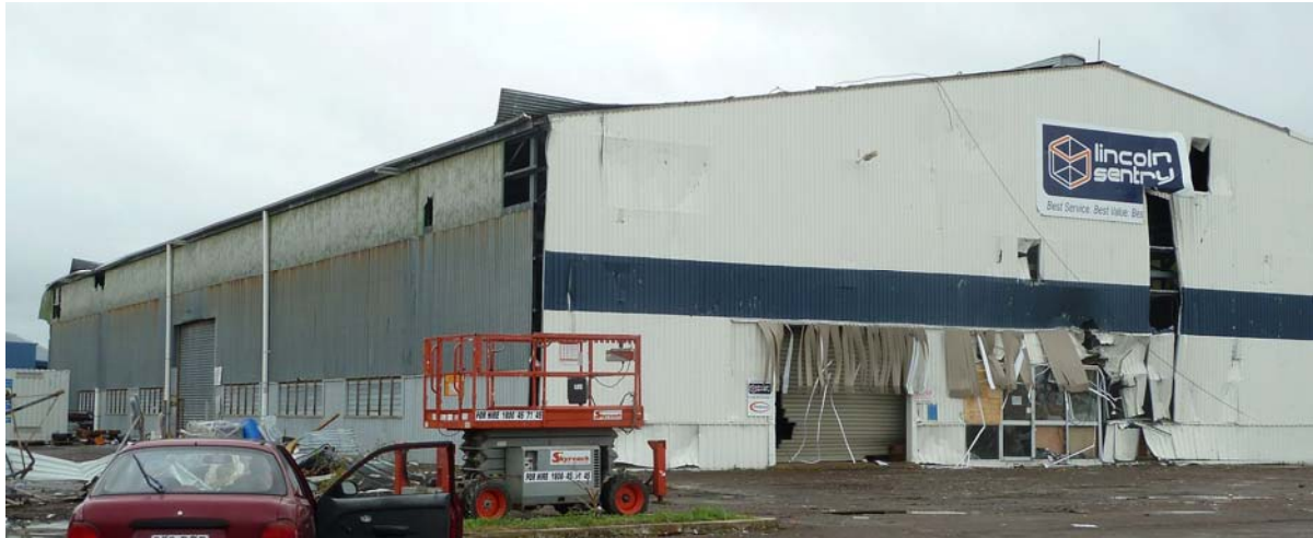
Figure 3.6: Debris damage and broken roller door on “windward” wall, and failed translucent wall cladding and peeled roofing on side wall
