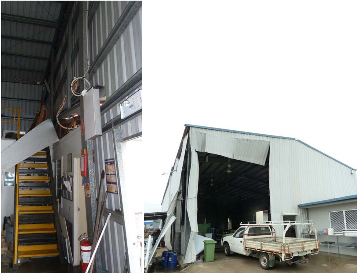
Figure 3.9: (a) Bend windward wall column, (b) Distortion of end portal frame and loss of roller door
