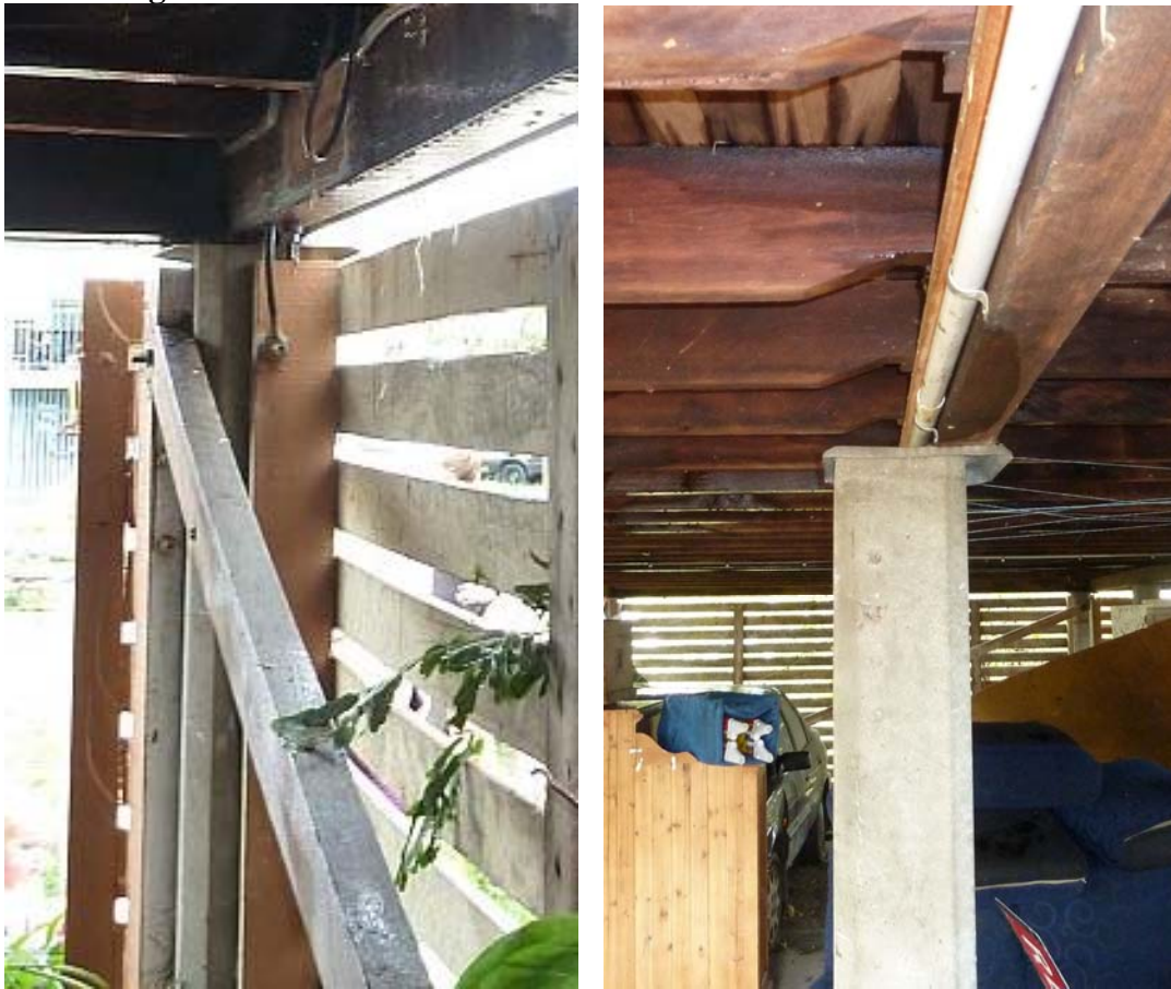
Figure 3.4 (a) Rotated cranked rod, (b) House shifted on piers
