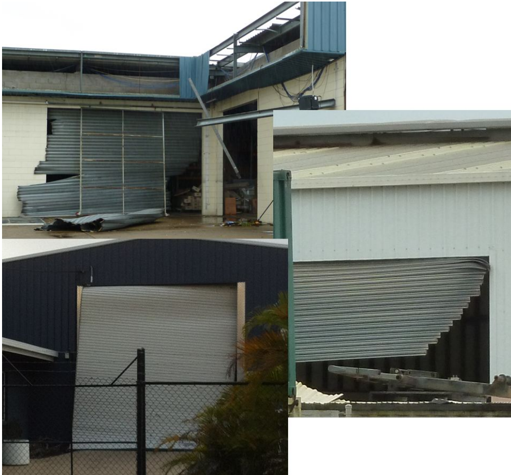
Figure 3.7: Damaged roller doors
