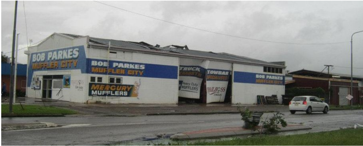
Figure 3.8: Impact to end wall, roof and failure of sliding doors and roof cladding
