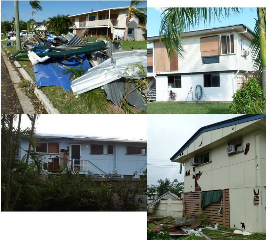
Figure 3.10: Wind driven debris and impacts on housing
