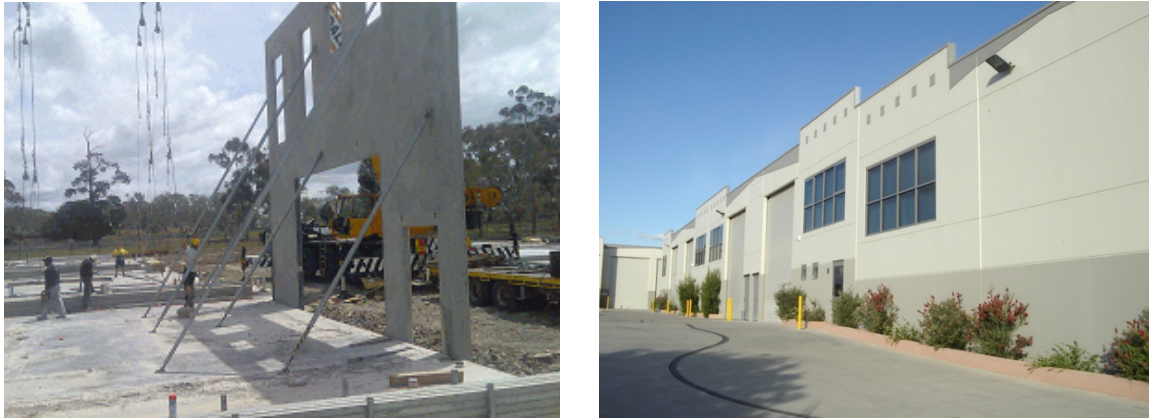
Figure 5: Concrete tilt-up buildings during and after construction
