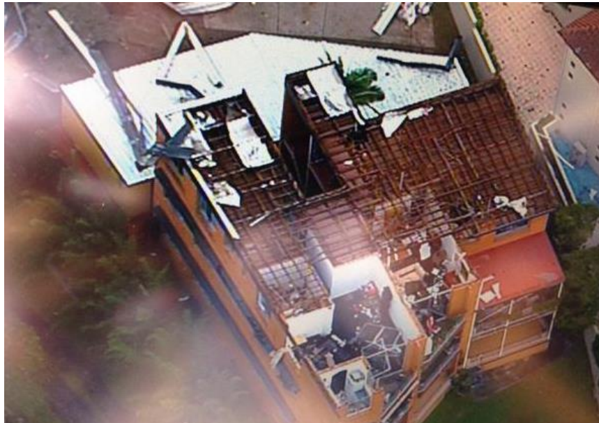
Concealed fixed roof sheeting torn off clips, unit complex with river frontage. Photographer: Peter Doherty. Location: Toowong. Source: < https://twitter.com/peterdoherty7 >
