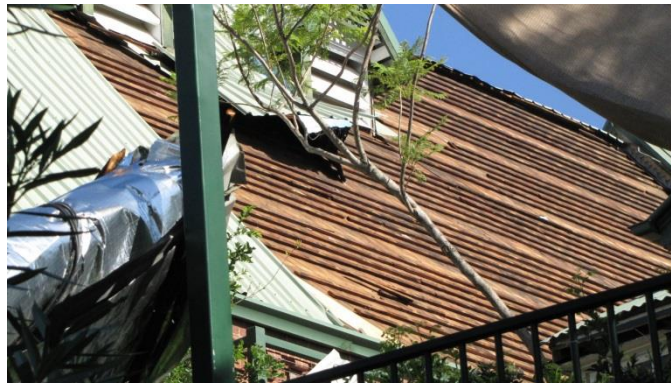
Figure 12: Loss of metal cladding and battens of a church. Originally a tile roof, the new metal roof was only secured to every 6 th timber batten.
