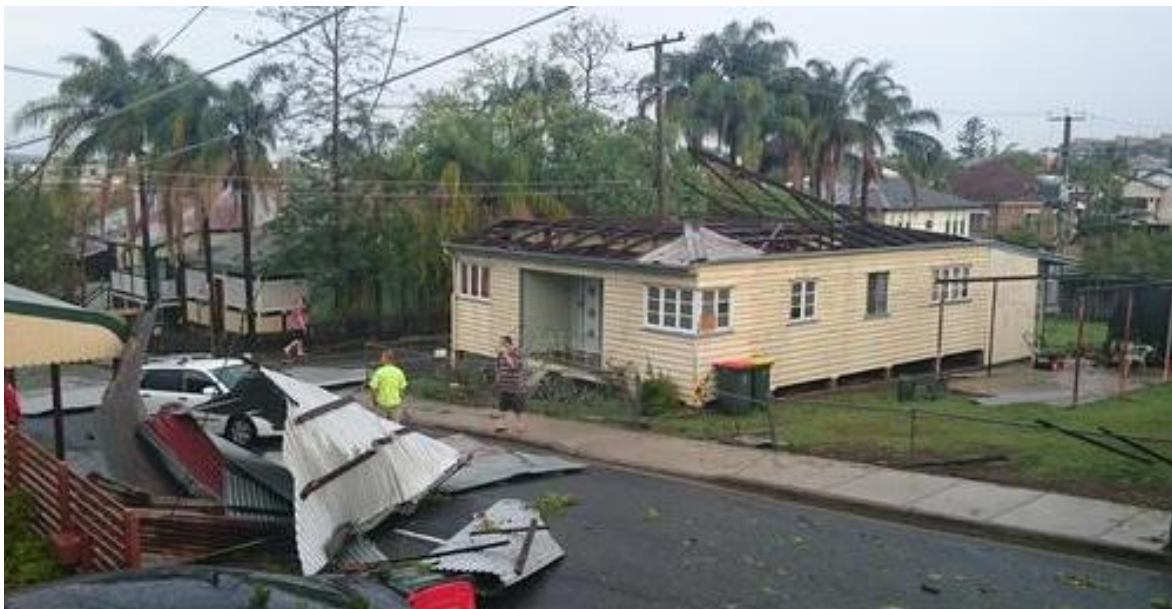
Roof sheeting attached to battens along with rafters have been torn off this worker's cottage. Photographer: Brad Schultz. Location: Ross St, Woolloongabba. Source: < https://twitter.com/superbrudd/status/537871622980382720/photo/1 >
