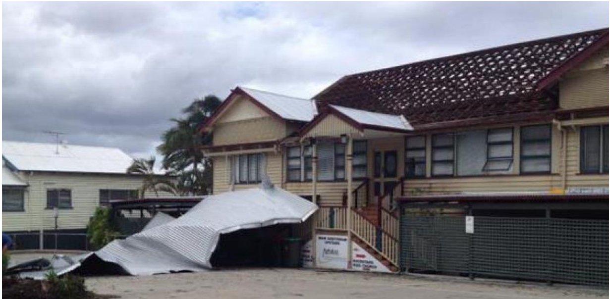
The roof sheeting from this church has been torn off its battens. The roof appears to have been tiled before being replaced by metal sheeting. Photographer: Andree Withey. Location: Ipswich road, Annerley. Source: < http://www.abc.net.au/news/2014-11-28/roof-gone-in-brisbane-storm/5926234 >
