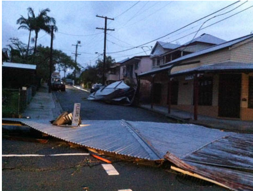
Roof sheeting with battens attached torn off building. Photographer: Brendan Fearn. Location: Woolloongabba. Source: < http://www.abc.net.au/news/2014-11-27/roofs-litter-the-streets-in-woolloongabba-after-the-storm/5923980 >
