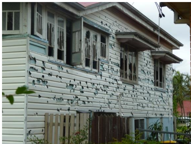
Figure 21: Hail damage to windows and vinyl cladding of an older house. The proximity of the neighbouring house on the right and the size of the window shades suggest hail being driven at a sharp angle by the wind.
