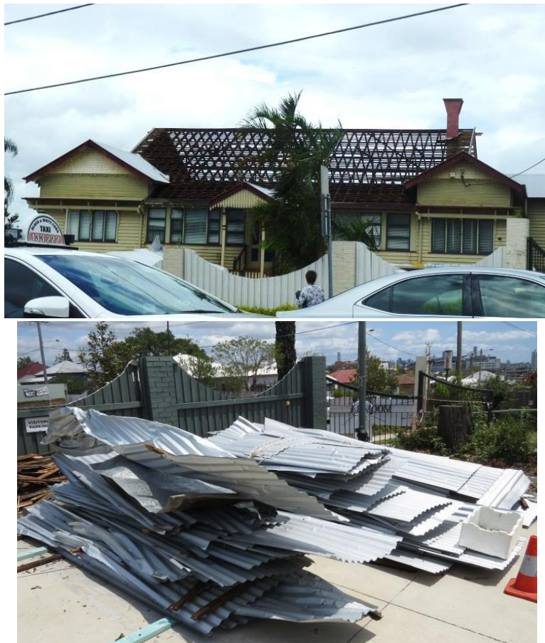
Figure 11: Loss of cladding and battens of a church hall. Originally a tile roof, new metal cladding was fixed to every 3 rd existing batten
