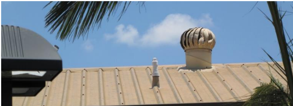
Figure 20: Typical hail damage to roof vent
