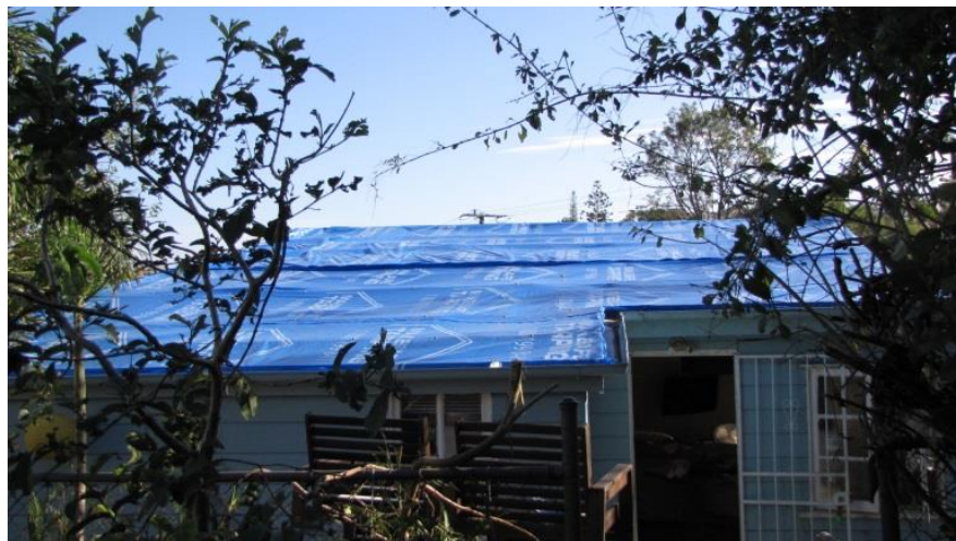
Figure 13: Loss of cladding and battens of an older home new cladding had been installed onto the original battens
