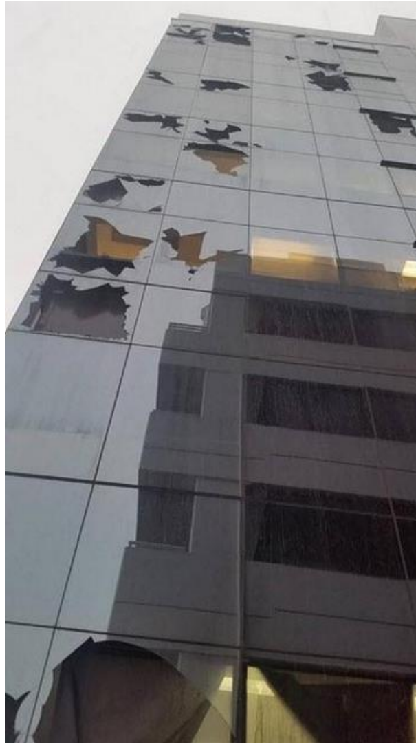
Hail damage to glass façade, Turbot St, Brisbane CBD. Source: Jessy Sahota < https://twitter.com/JessySahota >
