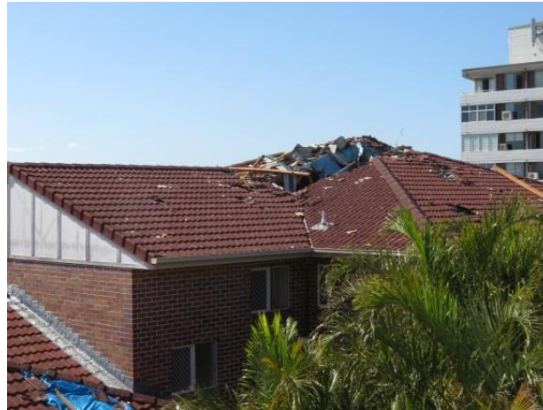
Figure 16: Damage caused by debris originating from a neighbouring apartment building. The tile roof, including the large south (windward) facing gable, appears otherwise undamaged
