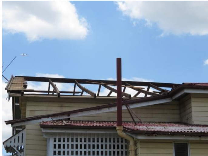
Figure 10: Loss of metal cladding and battens of an older house, original lead-headed nails were used to secure cladding to battens.
