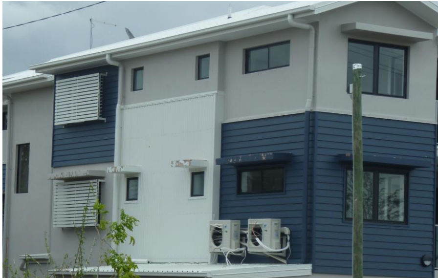
Figure 22: Significant hail damage to air-conditioning units of a newer apartment building. Note that all windows are undamaged, even those without overhanging eaves (far left), once again indicating the improved performance of new window glass in comparison to older windows in adjacent buildings.
