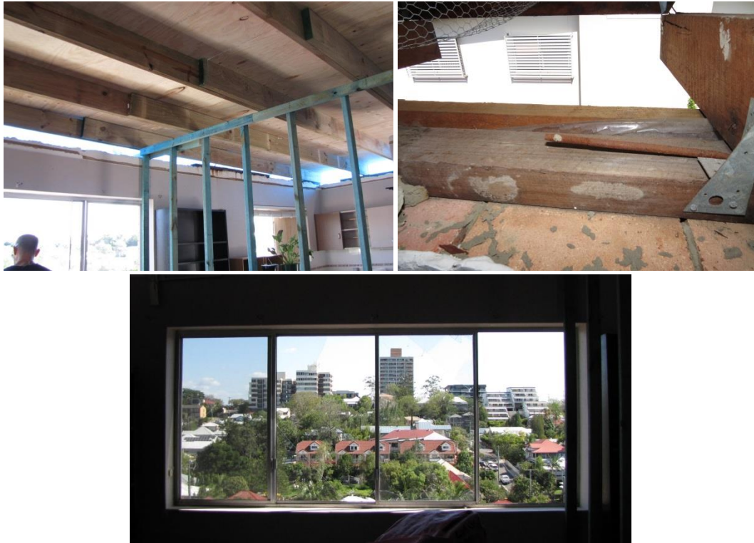
Figure 14: An example of complete roof loss of the top storey unit of a 3 storey apartment building (New roofing currently being installed). Original timber rafters had inadequate tie down to withstand internal pressure due to the breakage of a large Southern facing window. The unit was also located on top of an escarpment (outlook shown in the lower photograph) and may have experienced slightly higher wind speeds.
