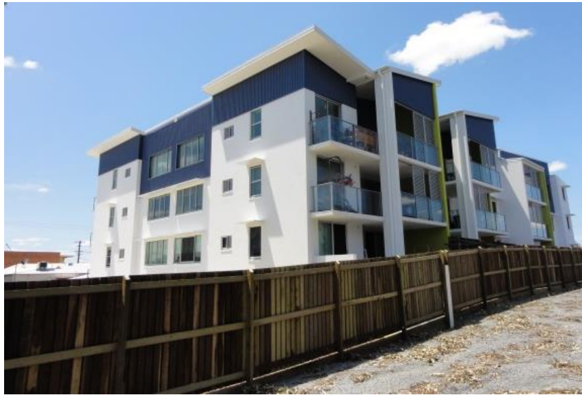
Figure 19: A new apartment building in a storm affected neighbourhood, all windows on the exposed southern side were undamaged, indicating the improved performance of new window glass.
