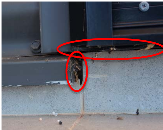
(a) Gaps between tiles and door frame
