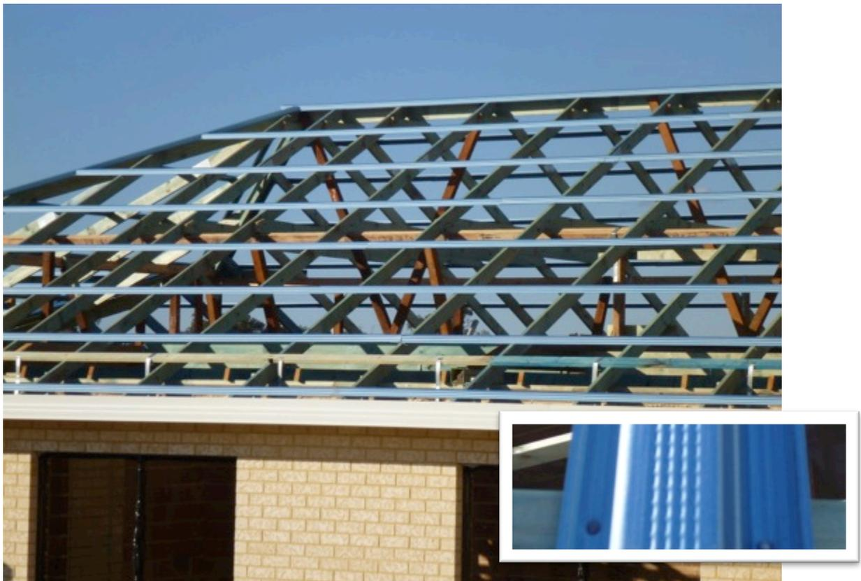
*Figure 1.1 – Gun-driven nails used in metal battens (inset shows top view of connection).*
