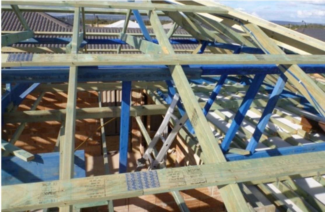
*Figure 1.3 – connections between 35 mm thick battens and rafters.*
