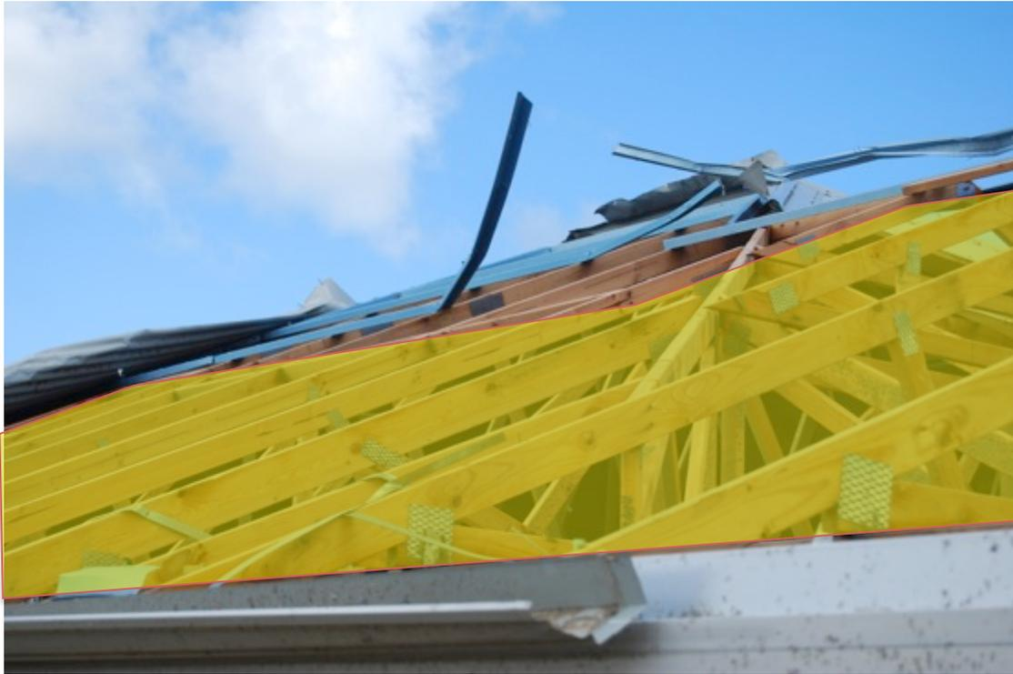
*Figure 1.2 – Failure of gun-driven nails connections between metal battens and trusses. (Shading shows area of batten to truss failure.)*
