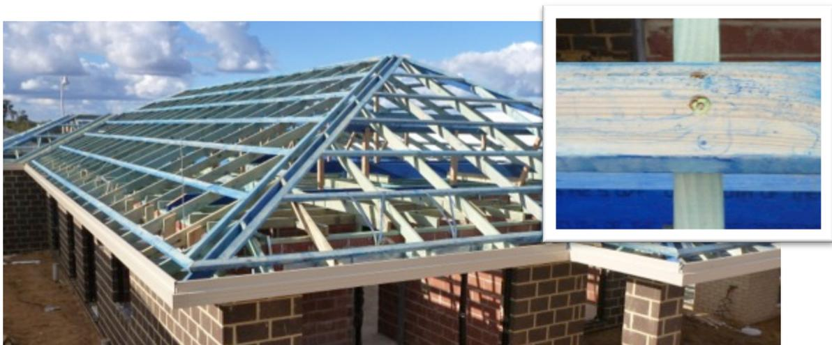
*Figure 1.4 – connections between 45 mm thick battens and rafters. (Inset shows connection detail.)*
